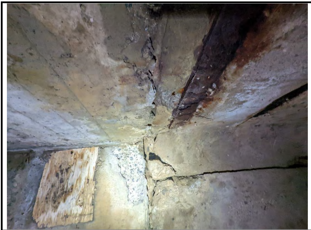
Photo 14 Rust and corrosion stains on soffit at section joints
