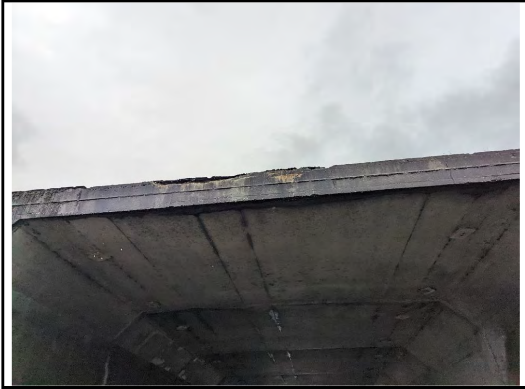
Photo 11 Spall with ECR at northeast barrel end
