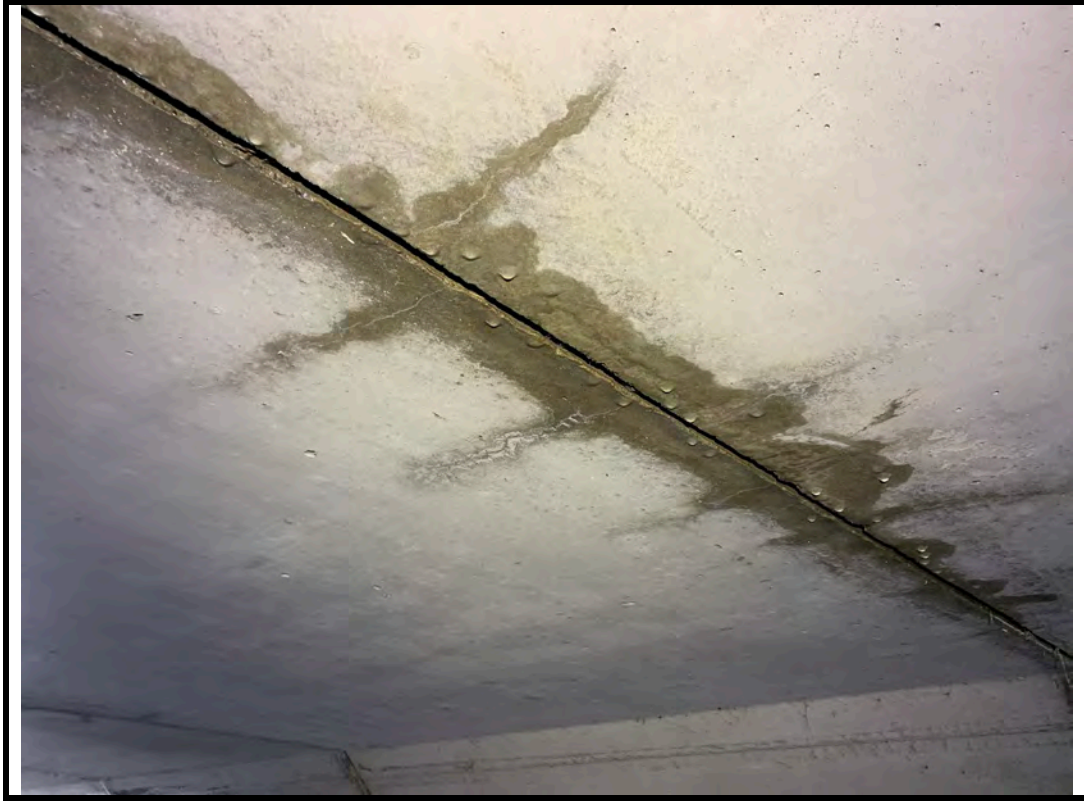
Photo 11 Active leaking at precast barrel joints
