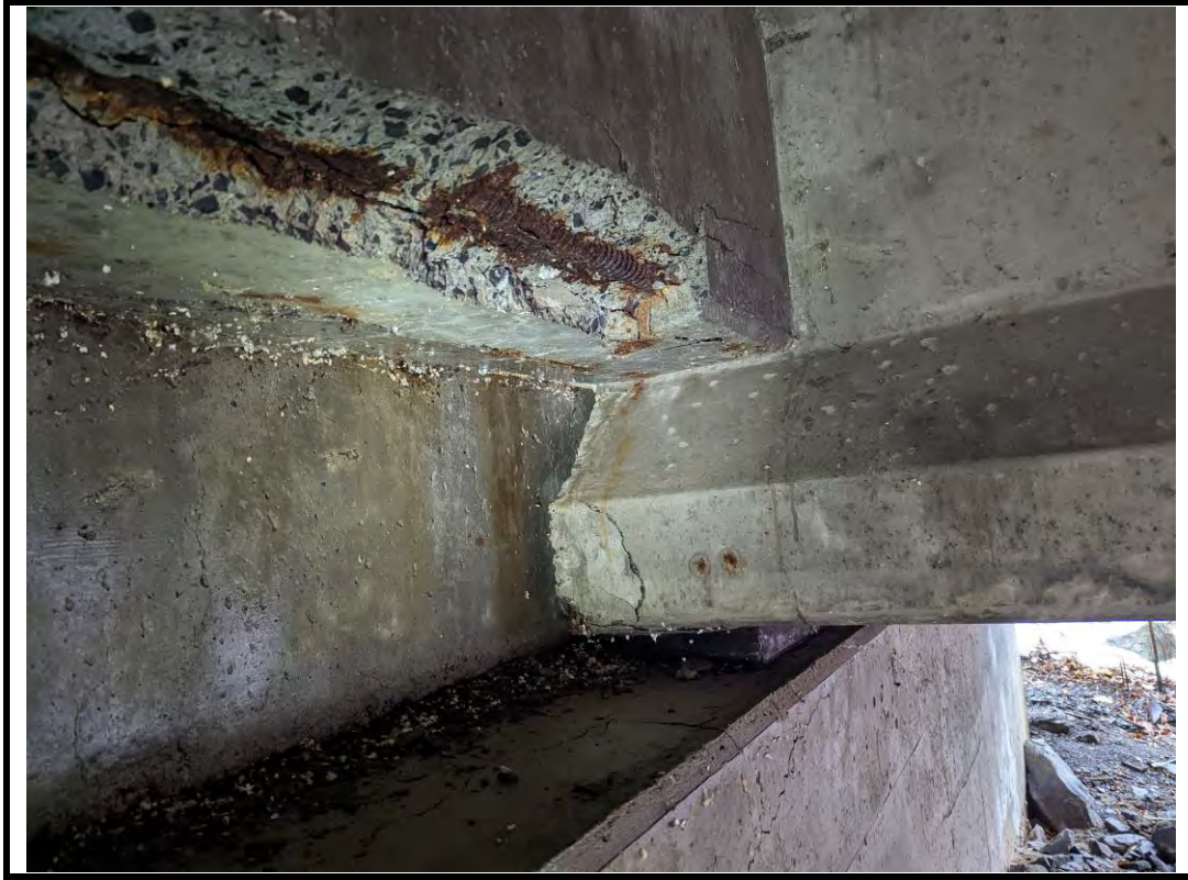
Photo 19 ECR and spalls at south girder ends and diaphragms
