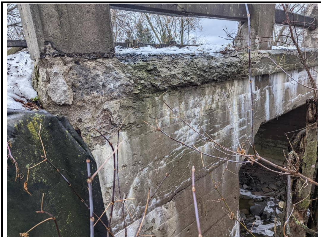
Photo 10 Spalls and efflorescence at northeast deck fascia/wingwall
