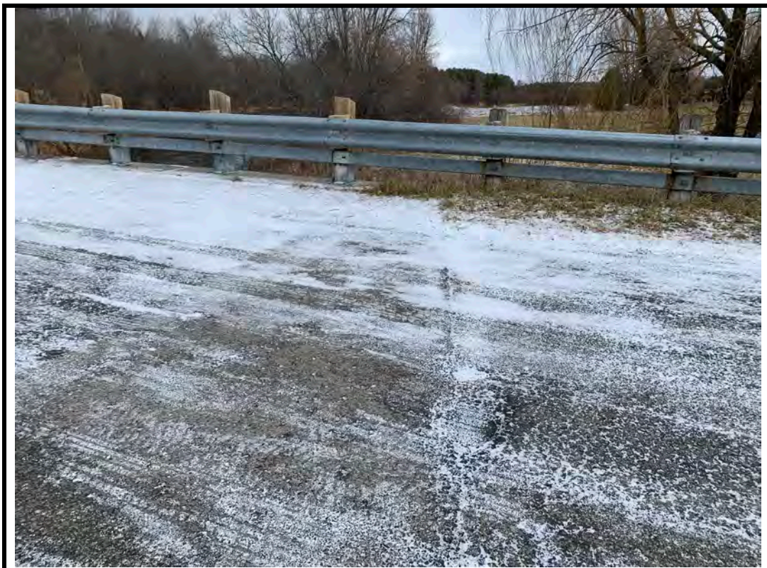
Photo 8 Wide crack at end of approach slab on east wearing surface
