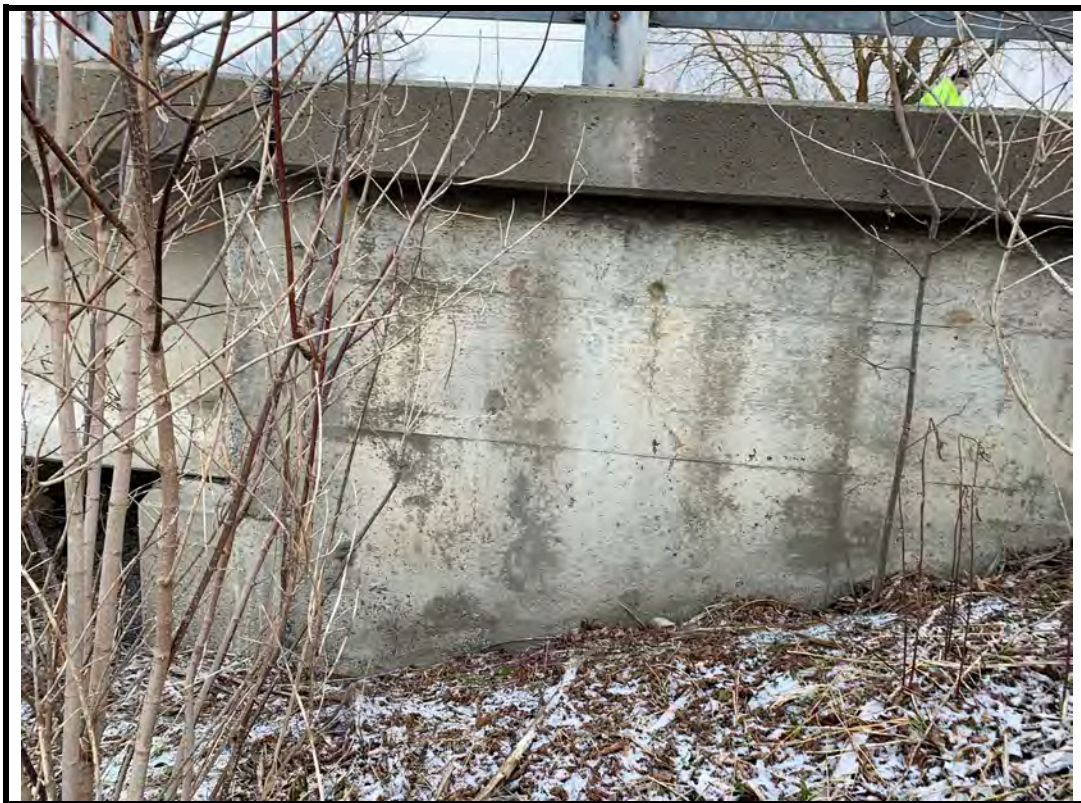
Photo 18 Narrow cracks on northwest wingwall
