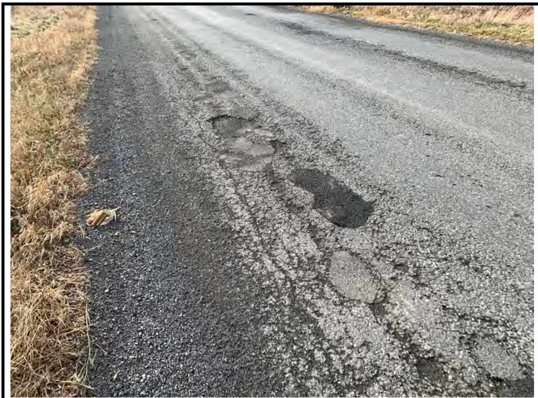
Photo 6 Potholes, and alligator cracks on edge of east wearing surface
