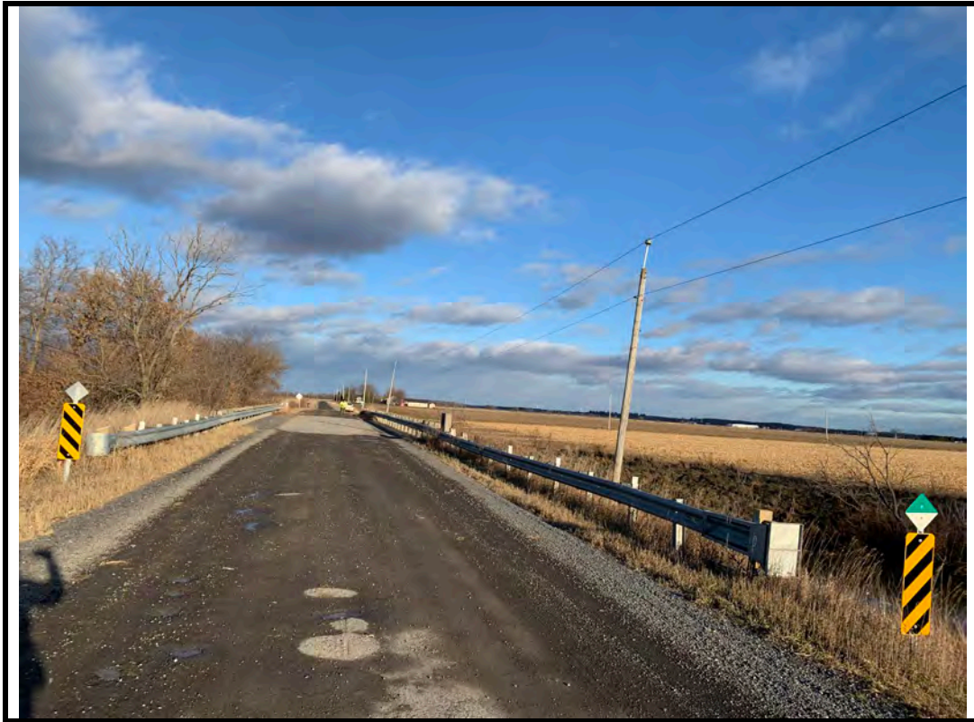
Photo 7 New end treatments at west end of structure
