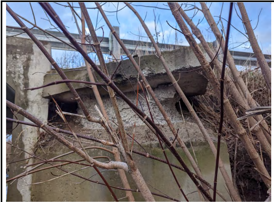
Photo 8 Severe disintegration at southwest retaining wall
