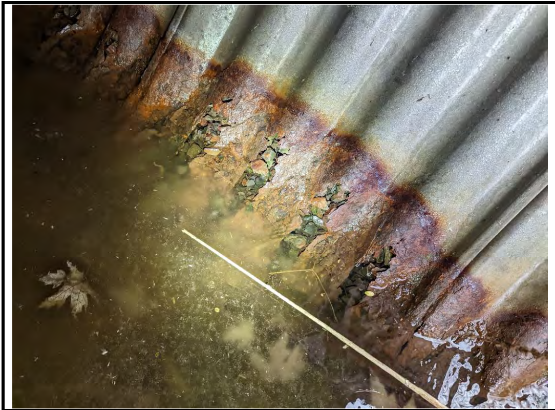
Photo 10 Perforations and corrosion at waterline in North barrel
