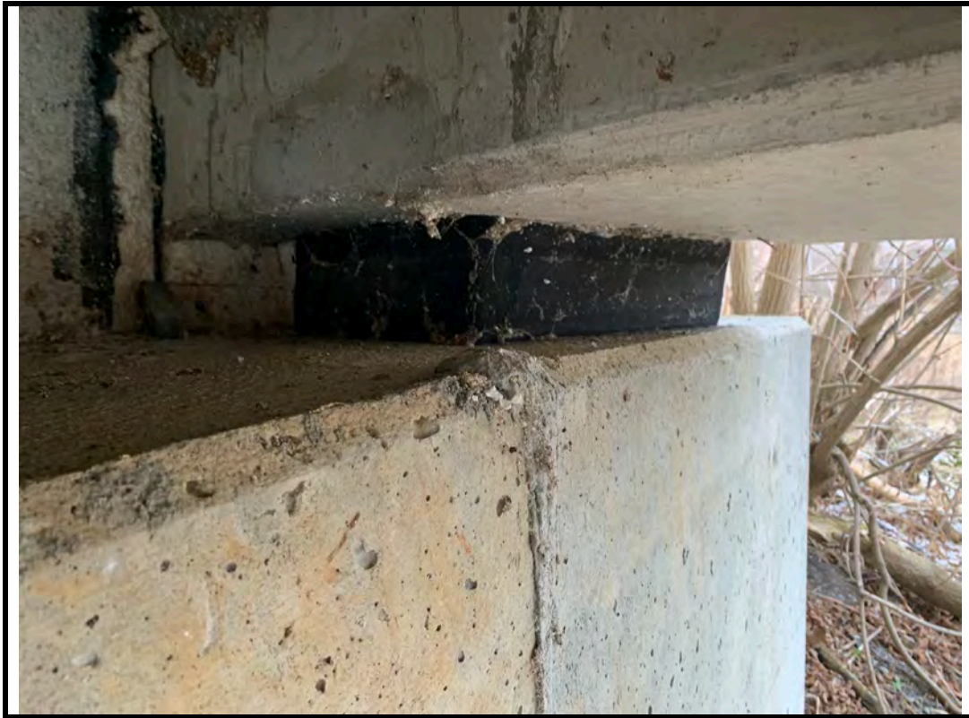
Photo 17 Bearing at northwest corner of structure
