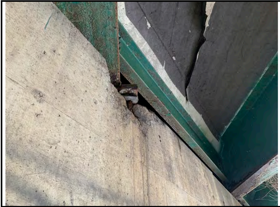
Photo 21 Spall below girder end on north abutment wall
