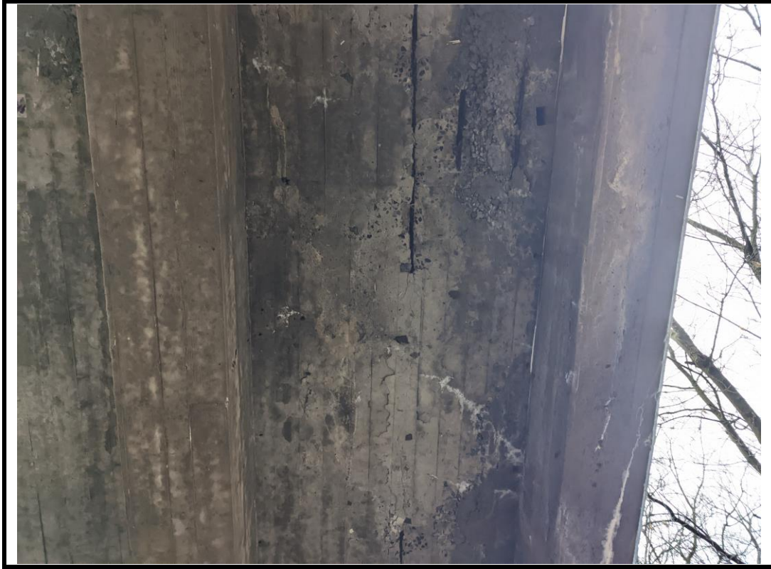
Photo 13 ECR, spalls, efflorescence and cracks on soffit (typ.)
