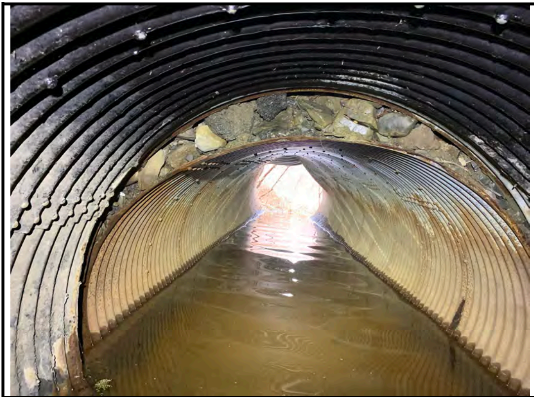
Photo 12 Separation and partial collapse of north barrel
