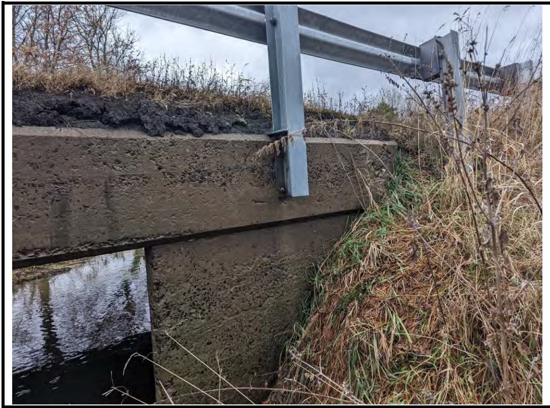
Photo 17 Scaling on wingwalls
