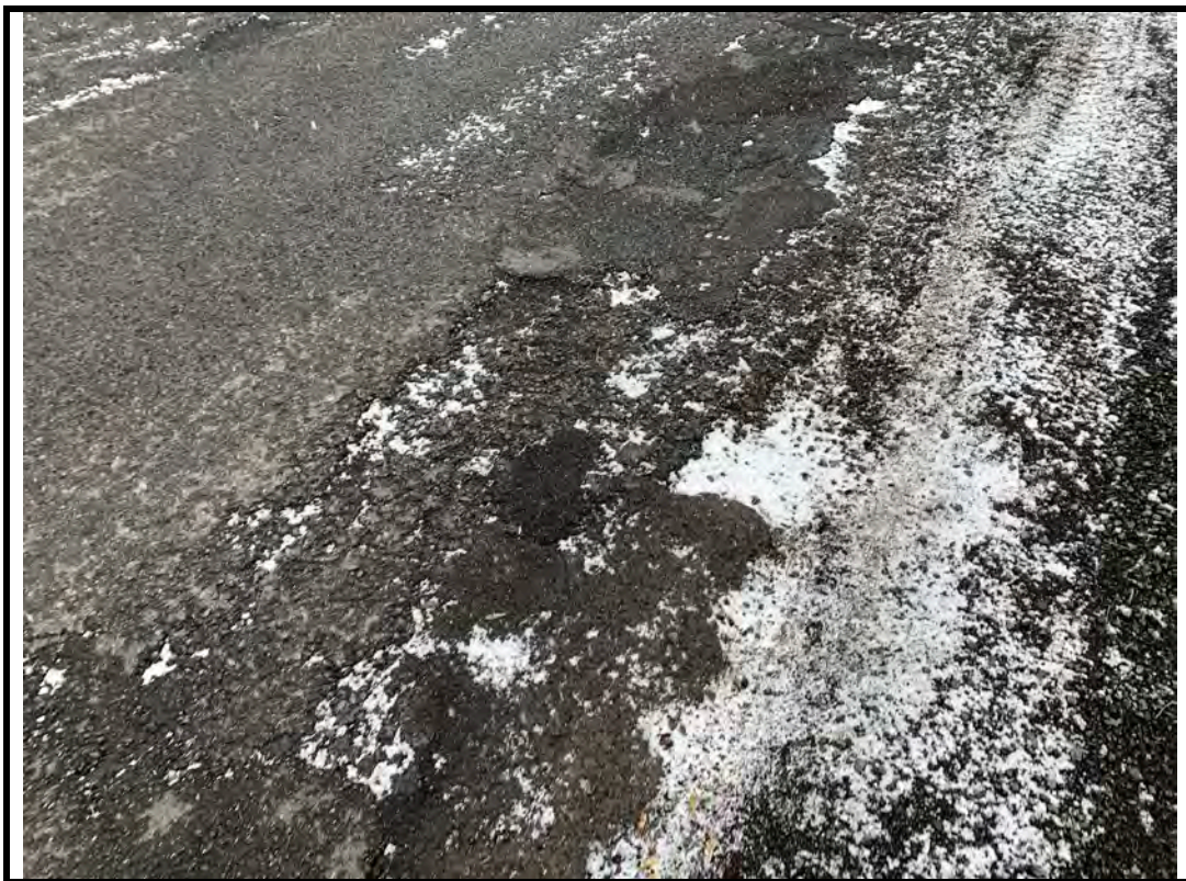
Photo 7 Potholes and patched potholes noted on south wearing surface
