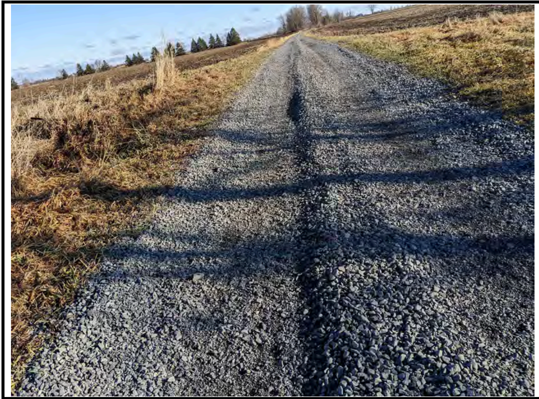
Photo 7 Severe settlement on east approach wearing surface
