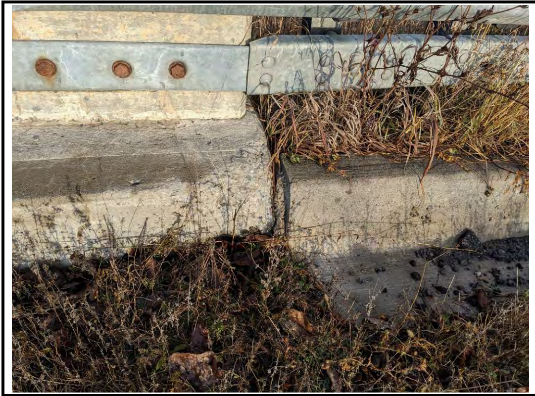
Photo 9 Spall on northeast barrier curb
