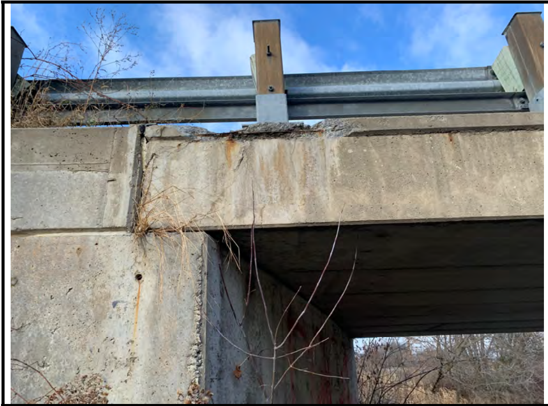
Photo 13 Spall with exposed corroded reinforcement at southeast corner
