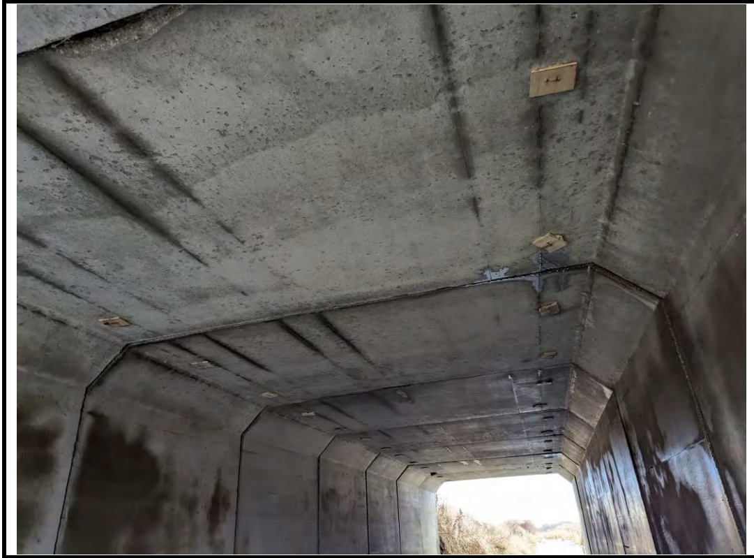
Photo 13 Leaking at second joint from East
