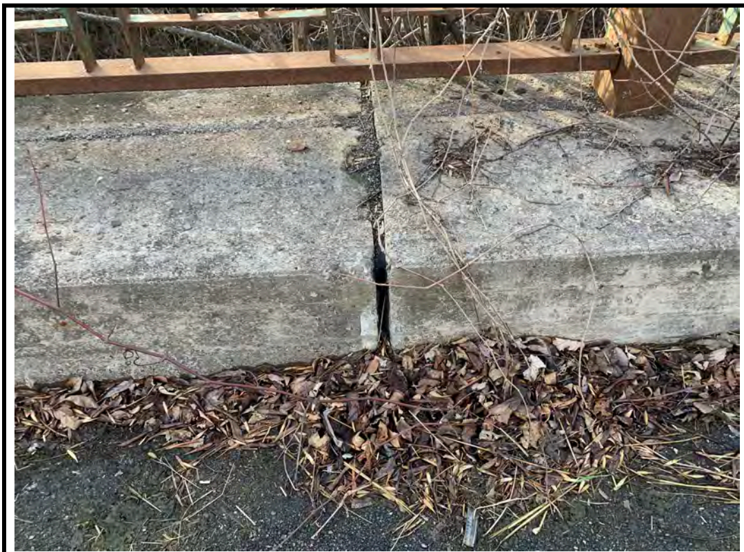
Photo 10 Scaling on top of west concrete curb
