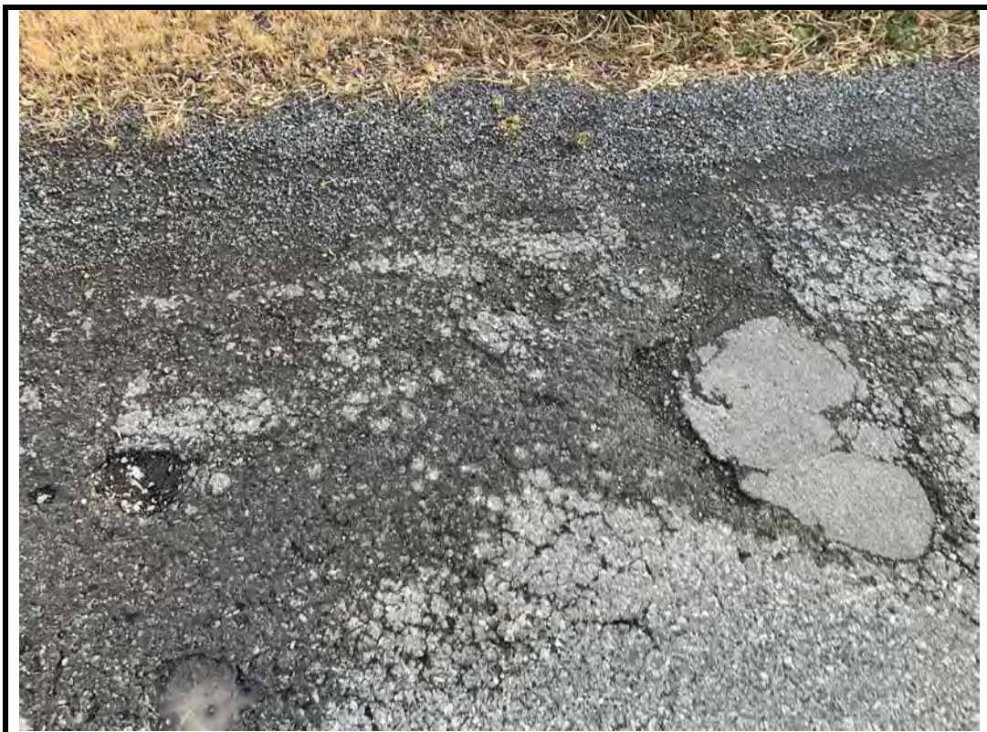
Photo 6 Potholes and alligator cracks on south edge of wearing surface
