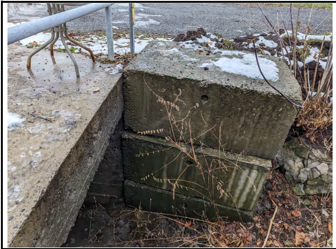
Photo 11 Scaling on SE concrete block retaining wall
