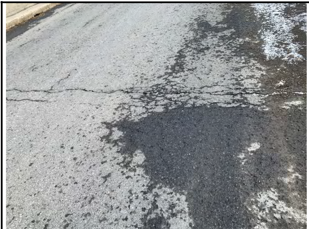
Photo 12 Wide crack at west end of deck
