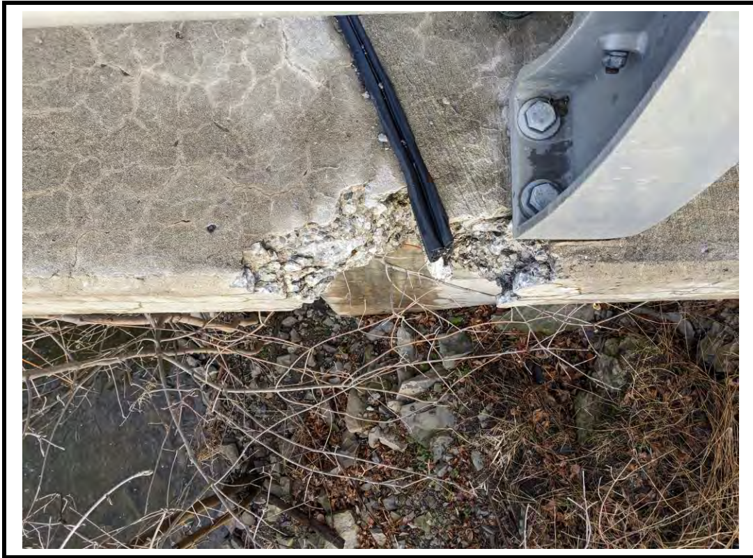
Photo 11 Spall at east joint and deck
