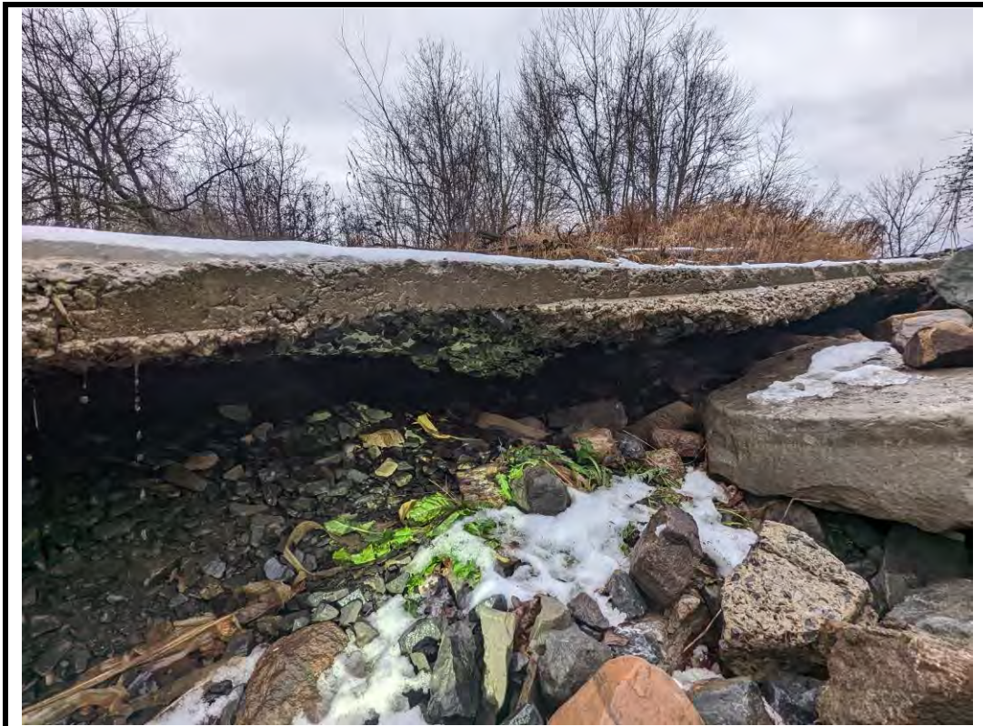
Photo 8 Severe undermining and loss of fill at North approach slab (2)
