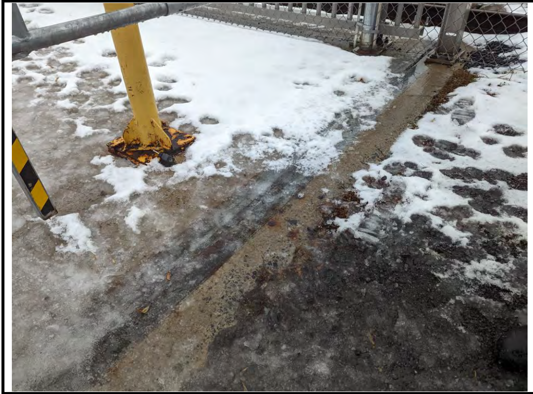
Photo 11 Abrasion at North end dam (Typical)
