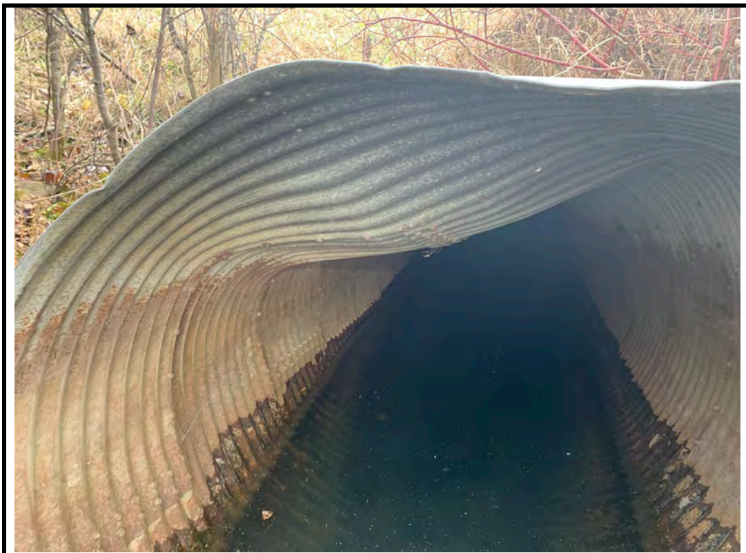
Photo 10 Large dents in east end of south barrel
