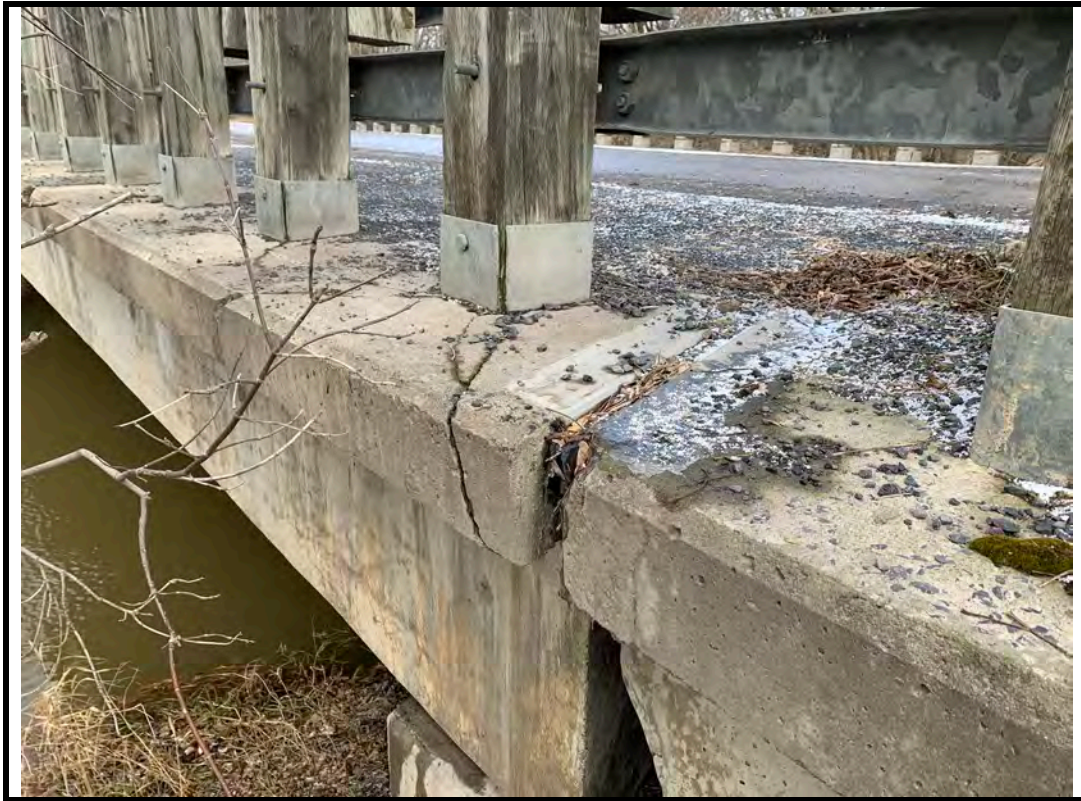
Photo 13 Crack at southwest corner of exterior soffit
