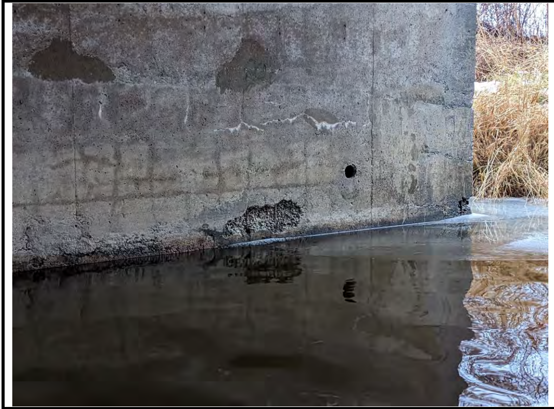
Photo 11 Spalls and honeycombing at springline along east abutment wall (typical)
