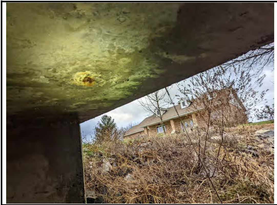
Photo 13 Small spall with ECR on the deck soffit
