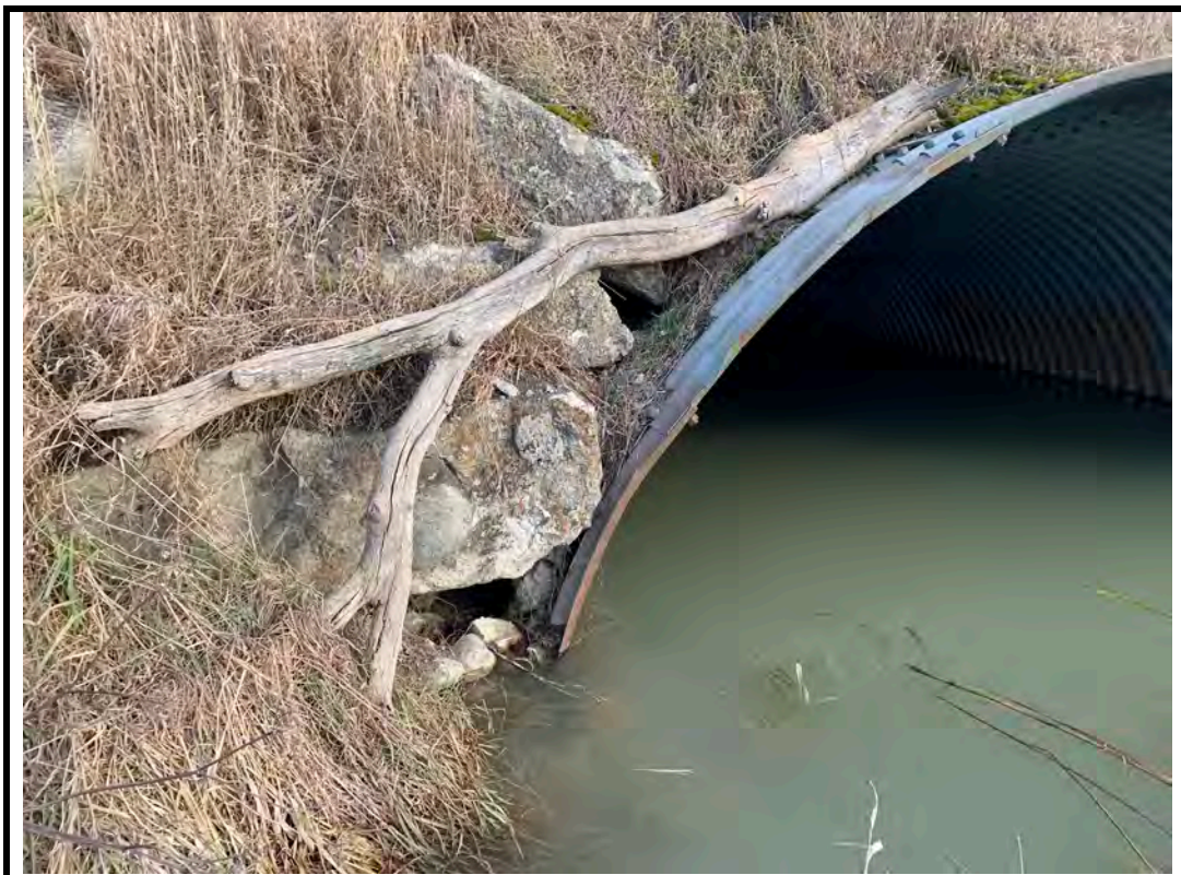
Photo 10 Some fill loss around barrel
