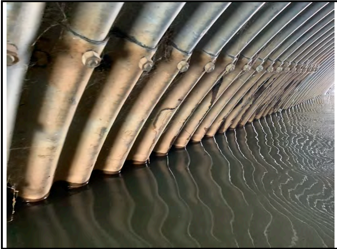
Photo 9 Light corrosion and evidence of leakage on barrel wall
