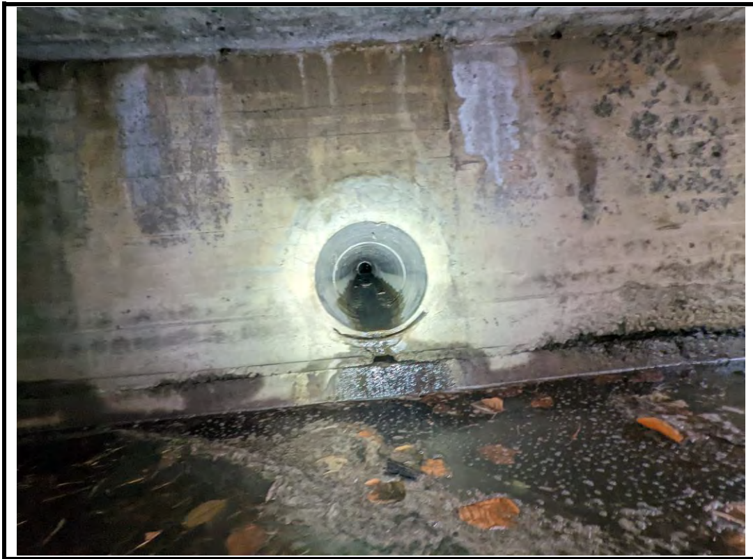
Photo 15 Pipe outlet in East culvert side wall
