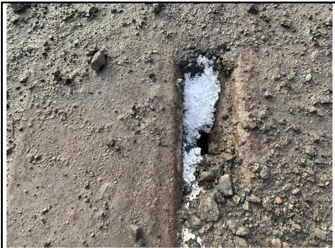
Photo 10 Damaged seal at north expansion joint
