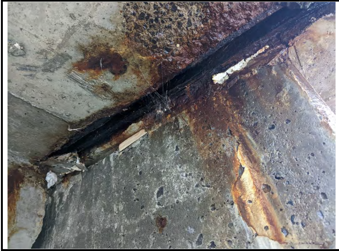
Photo 17 Evidence of failure at the south expansion joint with spalls and stains
