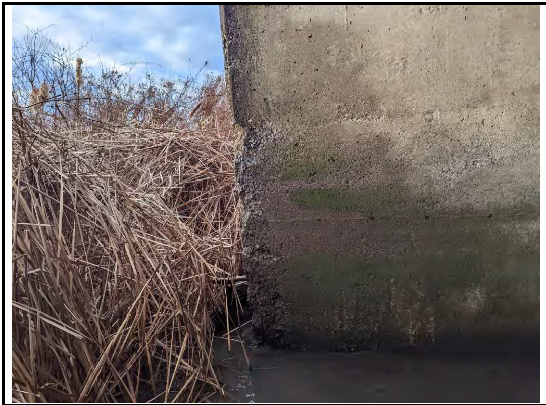
Photo 12 Spalls and honeycombing at the northwest of barrel.
