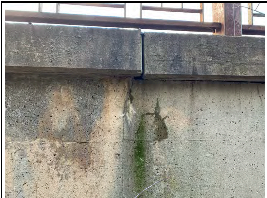
Photo 18 Medium cracks with efflorescence on southeast wingwall
