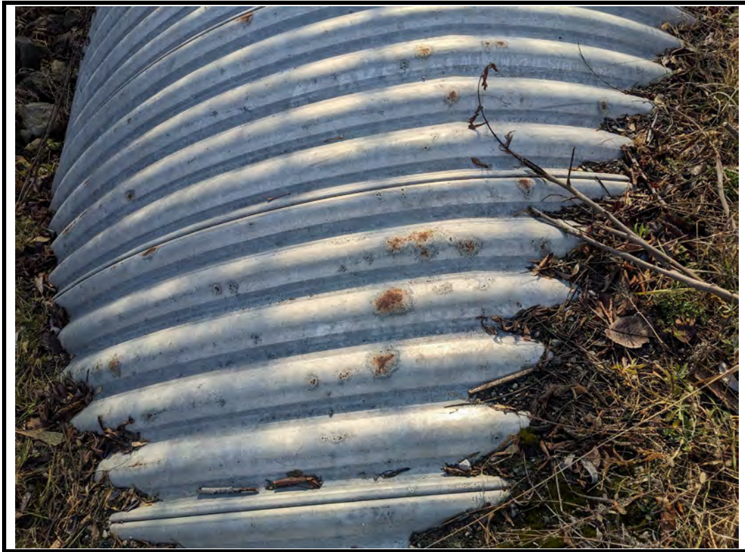
Photo 9 Localized rust spots on exterior of barrel at south end
