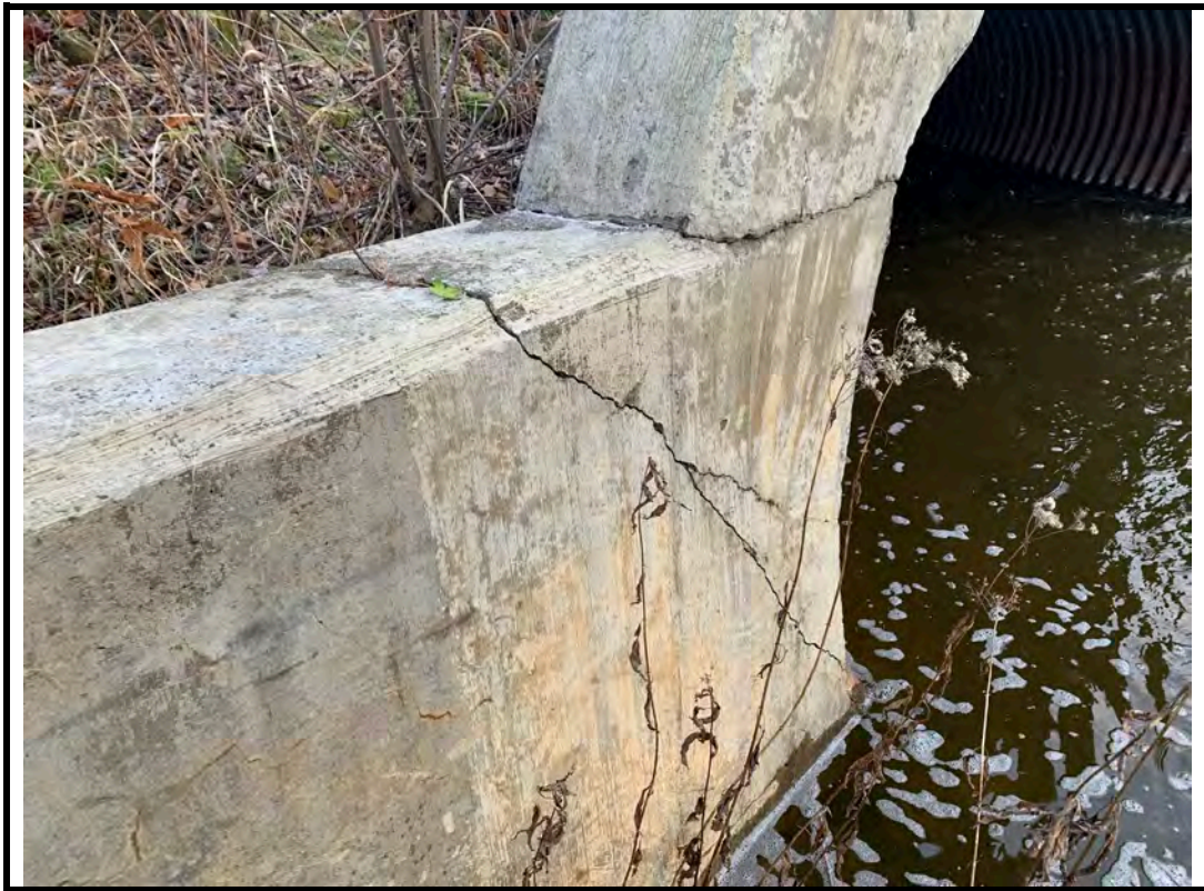
Photo 9 Wide crack at southwest corner of south concrete wall
