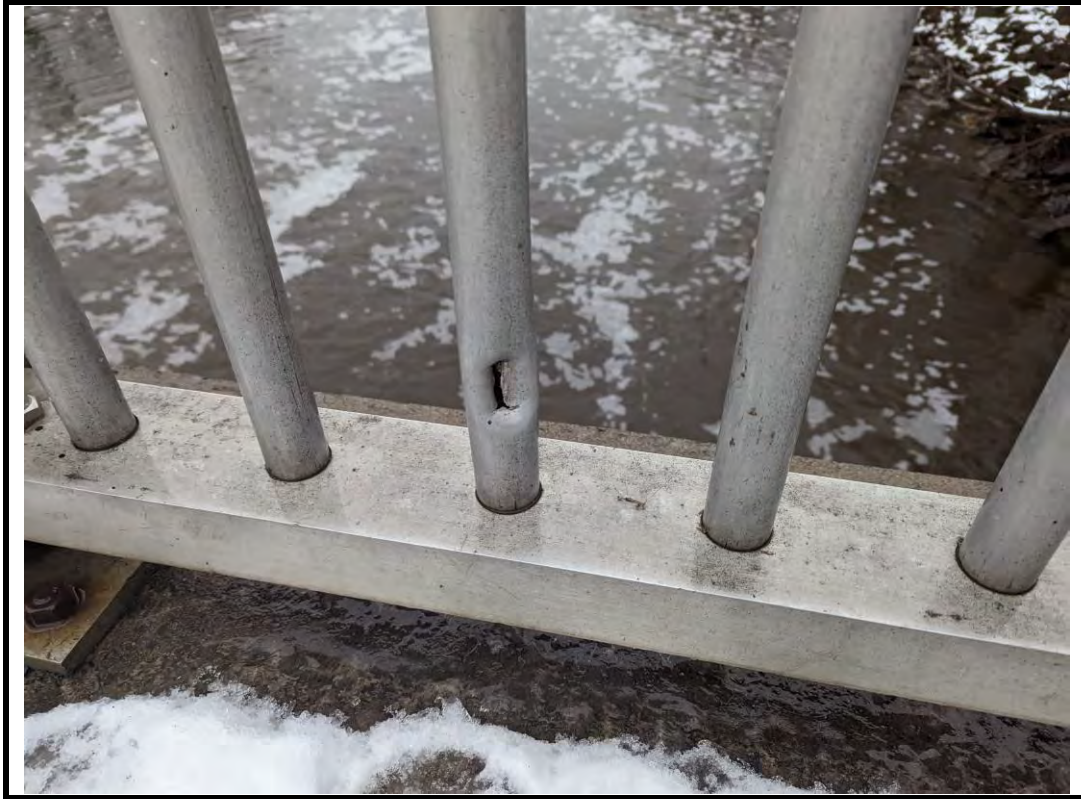
Photo 9 Perforation in deck barrier picket
