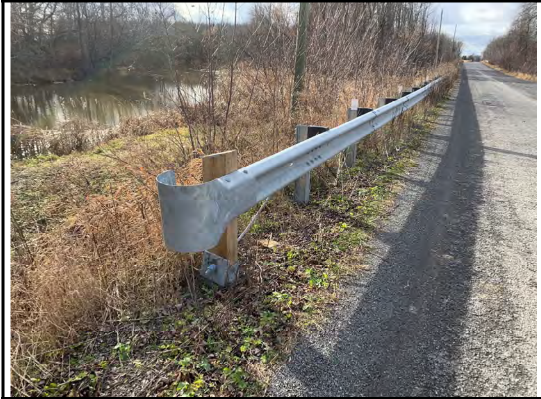
Photo 7 New end treatment at southeast corner
