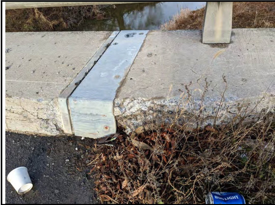
Photo 11 Spall at northeast barrier curb near joint
