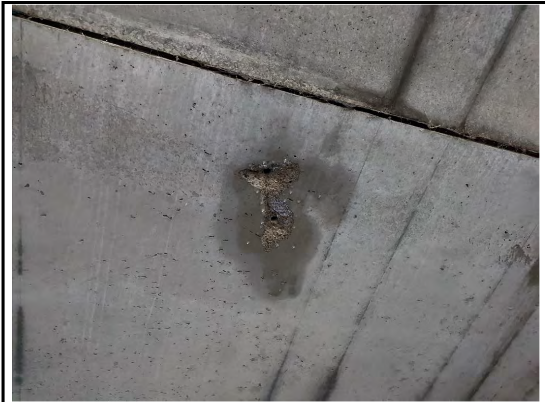
Photo 10 Spall with damp stain on north barrel soffit (typical)
