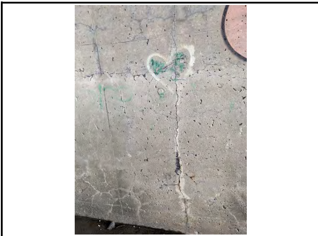
Photo 14 Wide vertical crack in east abutment wall with possible AAR
