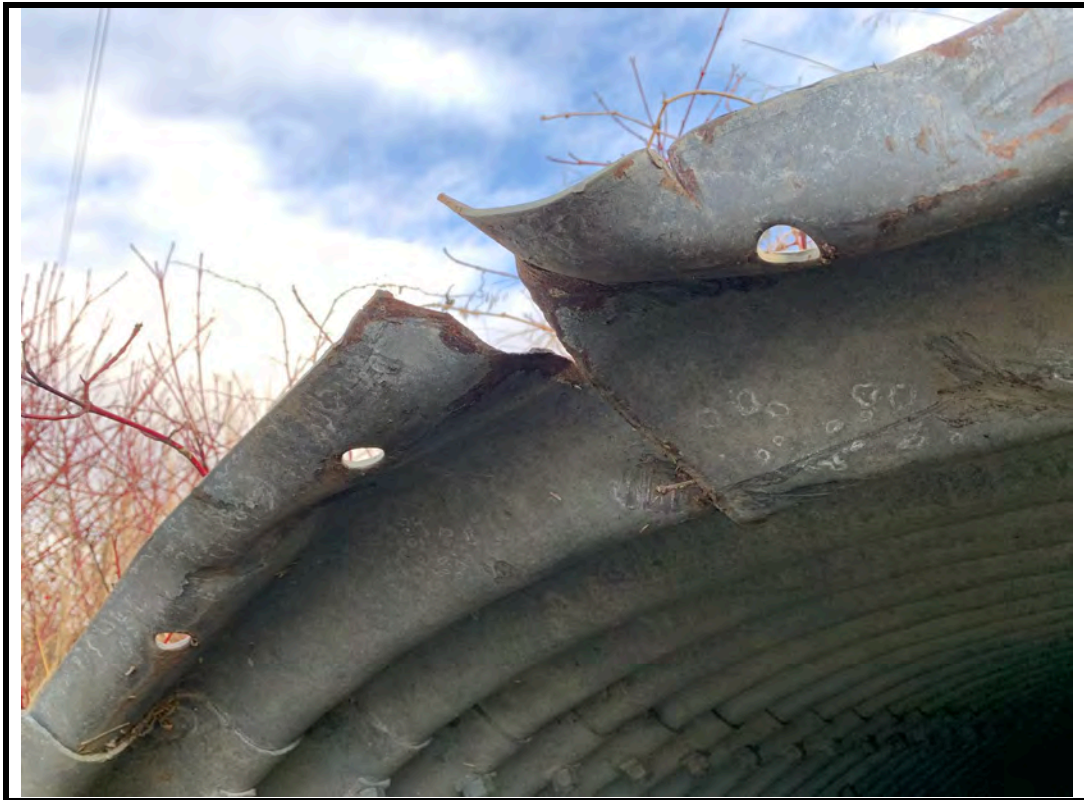
Photo 8 Perforations at north end of barrel
