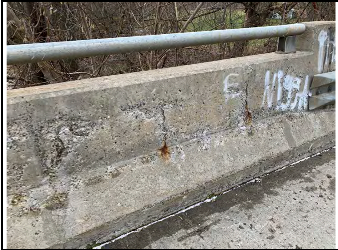
Photo 11 Spalls and disintegration noted on south end of east barrier wall
