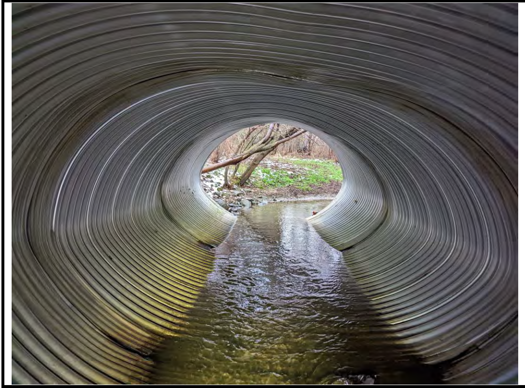
Photo 9 Deformation along top of pipe and light localized corrosion at joints
