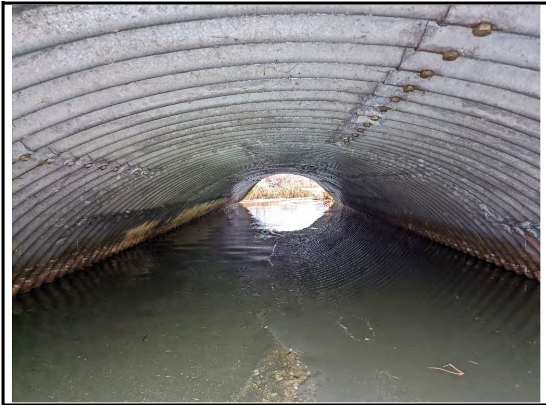
Photo 9 View through pipe arch barrel from the west
