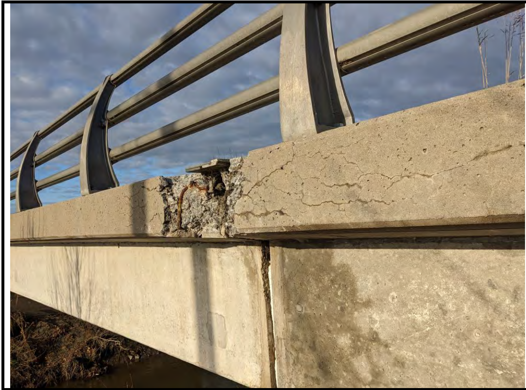
Photo 13 Spall at southeast joint and deck fascia
