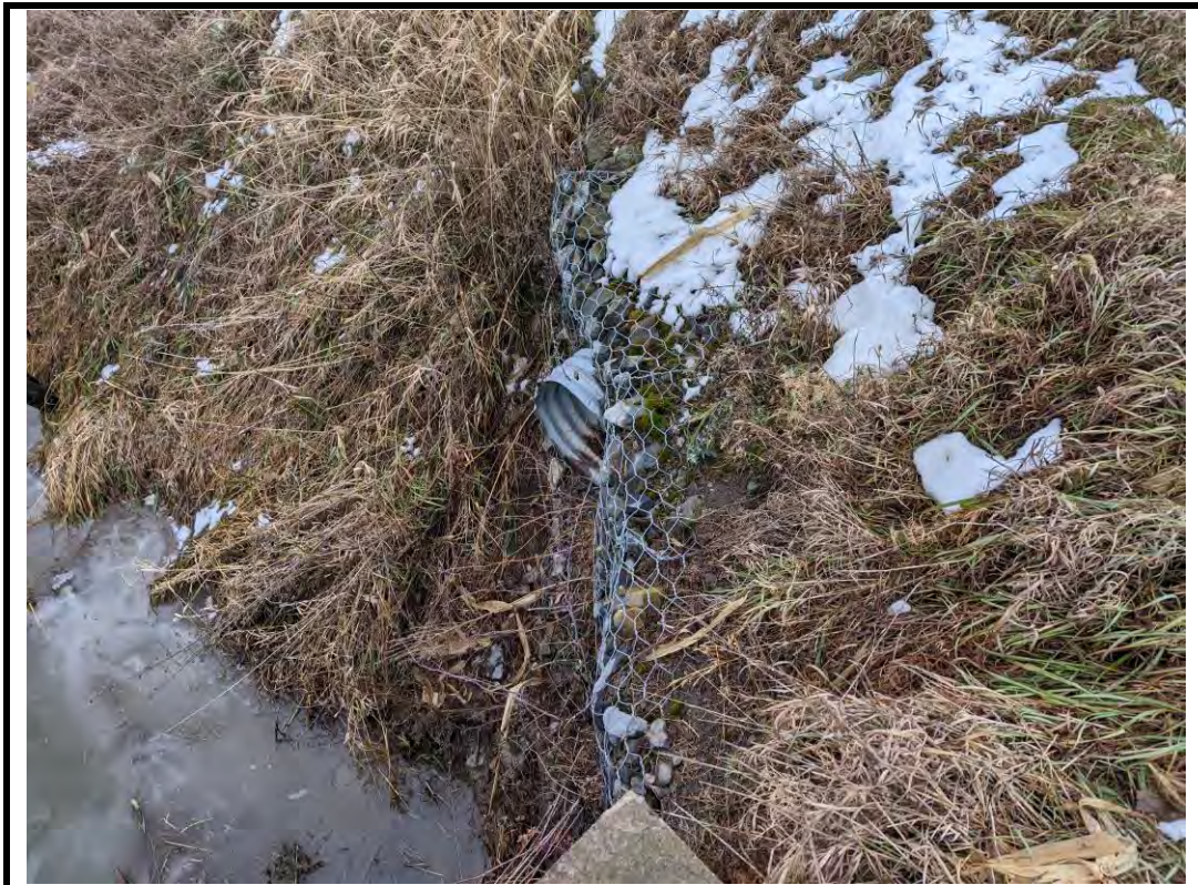
Photo 10 Southwest gabion wall leaning towards channel
