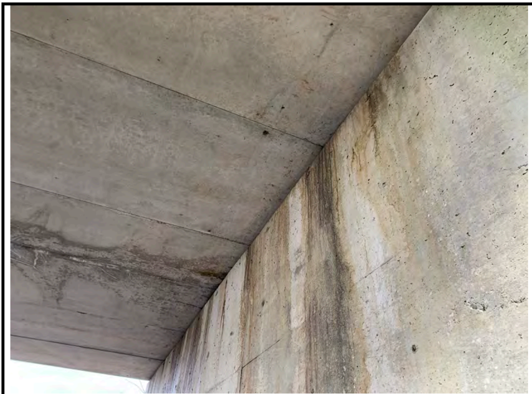
Photo 16 Staining at top of west abutment wall
