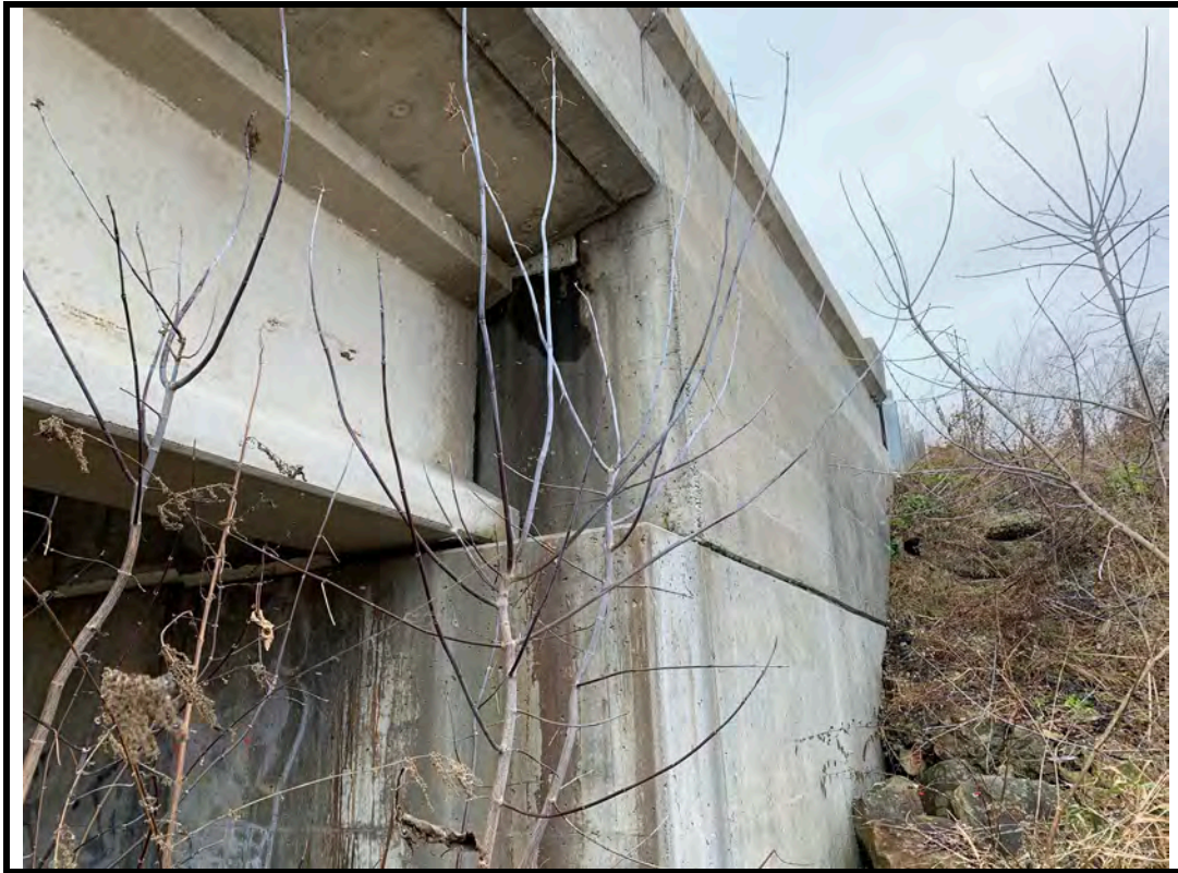
Photo 21 Damp stains and evidence of leaking seal on northeast corner of ballast wall
