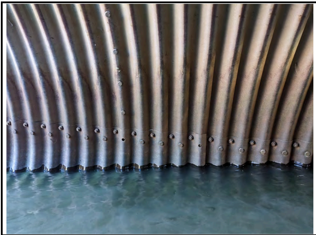
Photo 9 Light corrosion and missing bolt on east barrel wall
