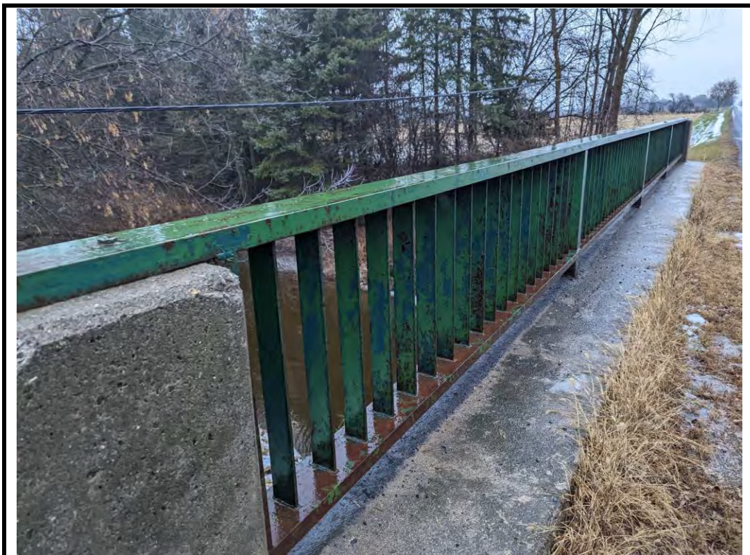
Photo 8 Corrosion and coating failure at north barrier railing (typical)
