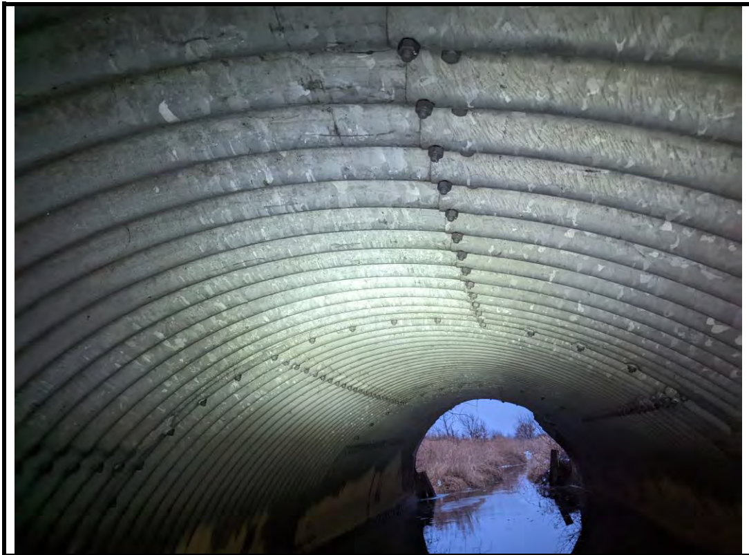
Photo 8 Sagging in pipe arch below roadway
