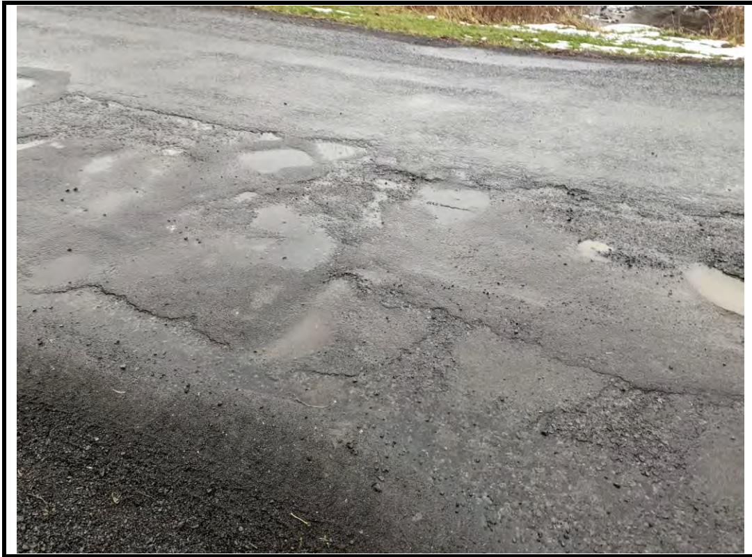
Photo 7 Roadway depression above structure, potholes, and raveling
