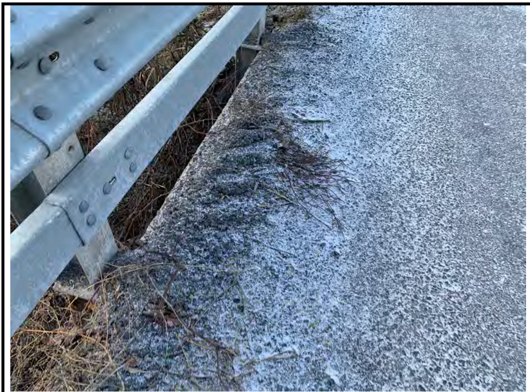
Photo 8 Vegetation growth at edges of roadway
