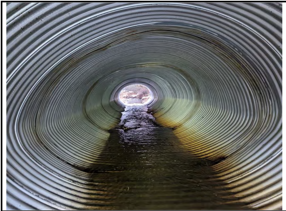
Photo 12 Corrosion along bottom of pipe and at joints
