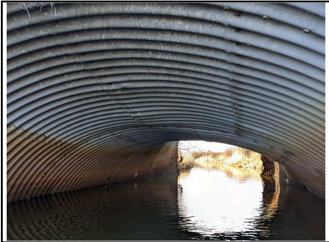
Photo 10 Severe sag in middle of barrel
