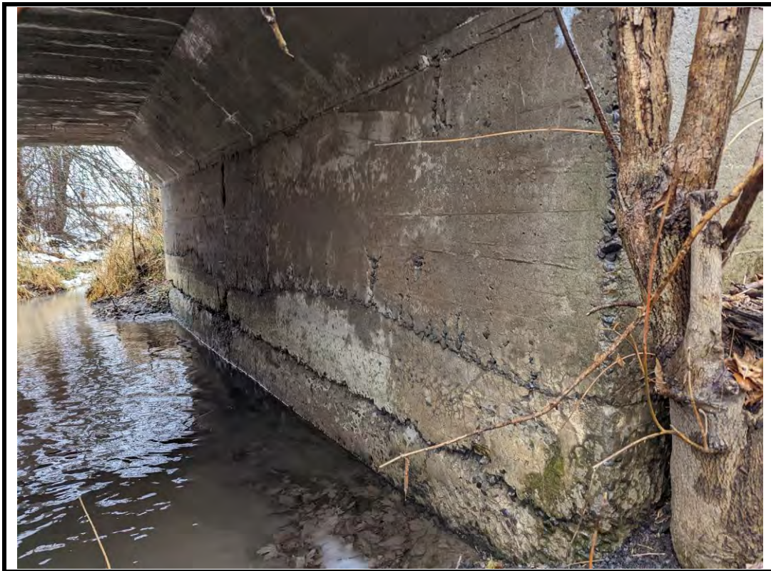
Photo 12 Severe scour/deterioration along barrel walls (typical)
