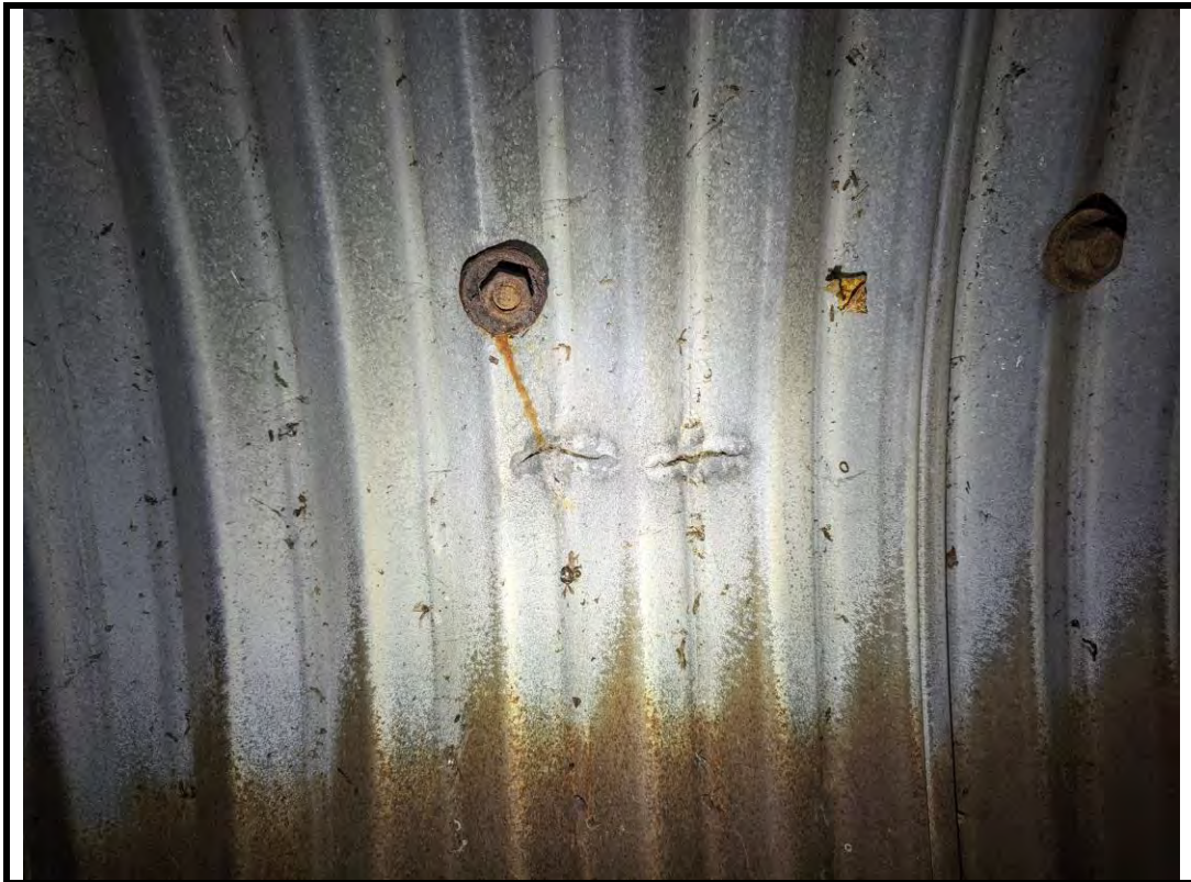
Photo 10 Perforations on barrel wall
