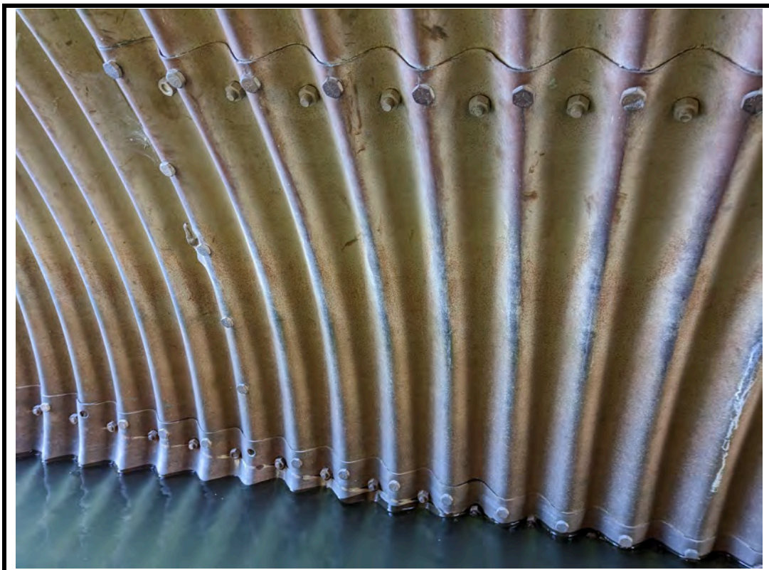
Photo 10 Cracks at bolt line at barrel wall
