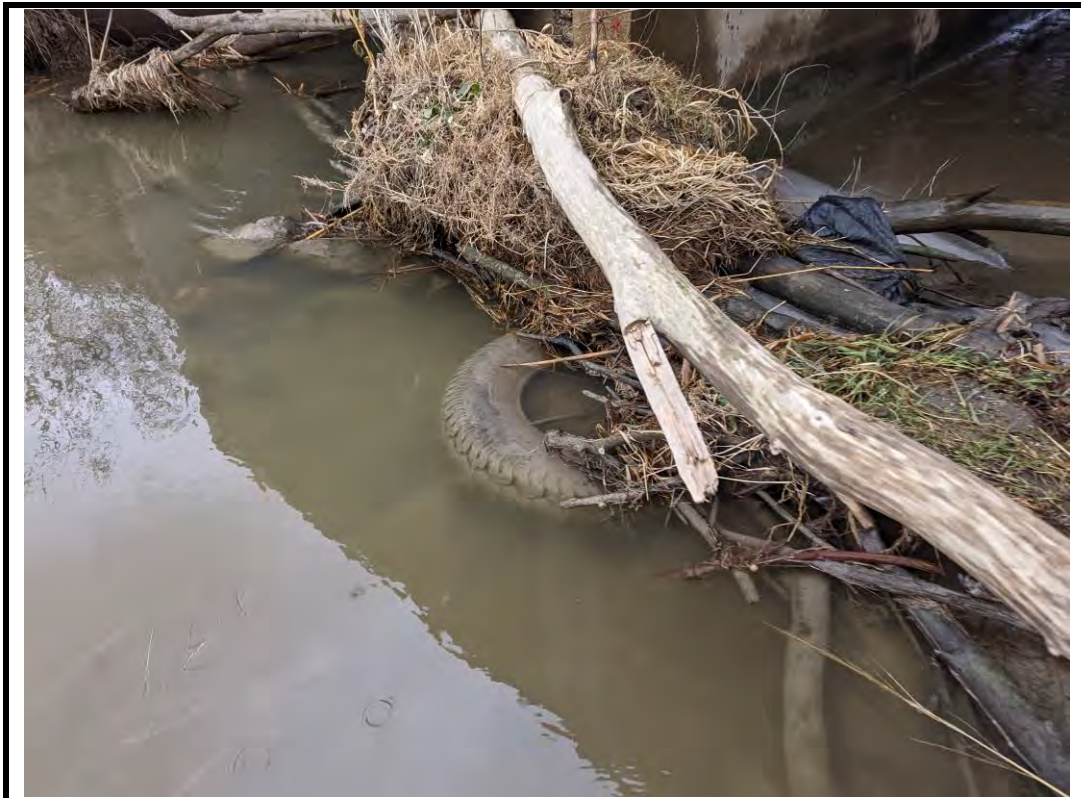
Photo 14 Heavy/Large obstructions at culvert inlet
