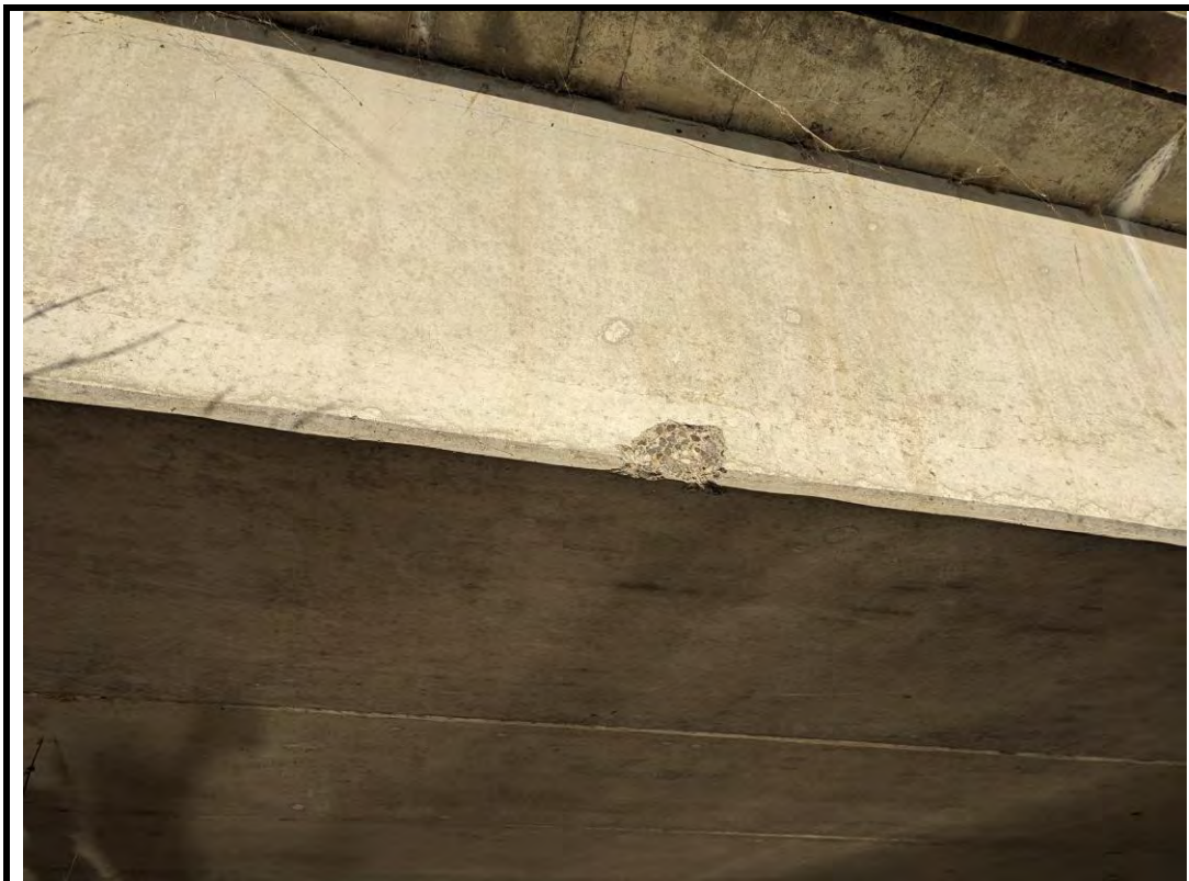
Photo 16 Small spall on south box girder side (named as soffit in report)
