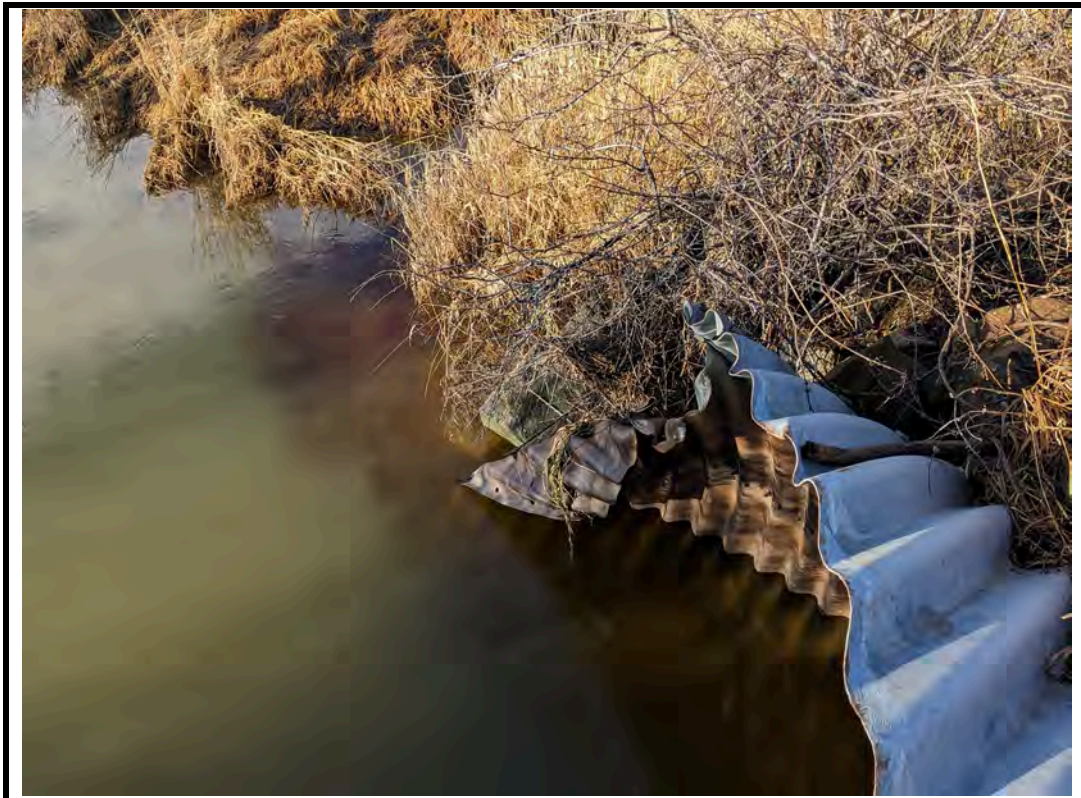
Photo 8 Deformation at northwest corner of structure
