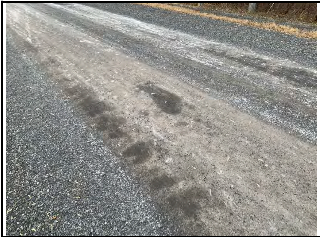
Photo 7 Moderate tire rutting on east wearing surface
