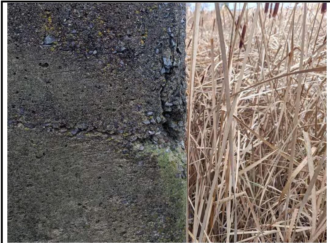
Photo 10 Spall/honeycombing at southeast of barrel
