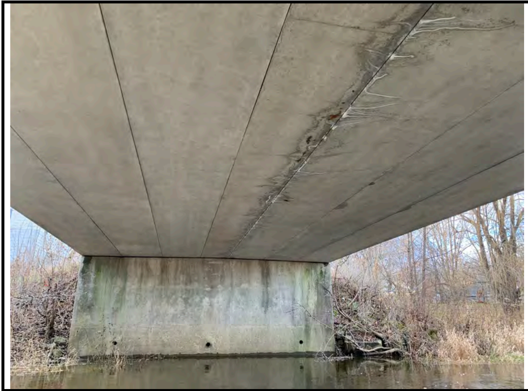
Photo 11 Efflorescence and evidence of leakage between box girders
