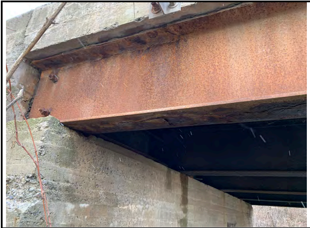
Photo 14 Flaking on bottom flange of exterior girder
