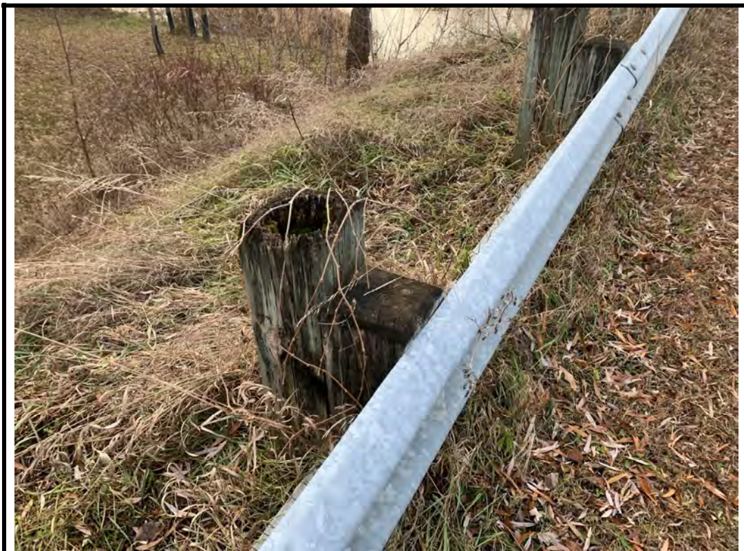
Photo 8 Severe rot on timber posts at southeast approach barrier
