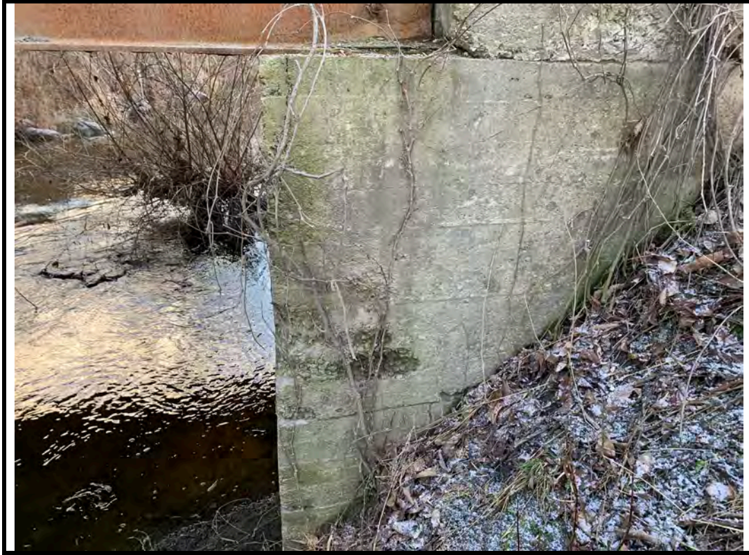
Photo 17 Severe honeycombing on northwest wingwall
