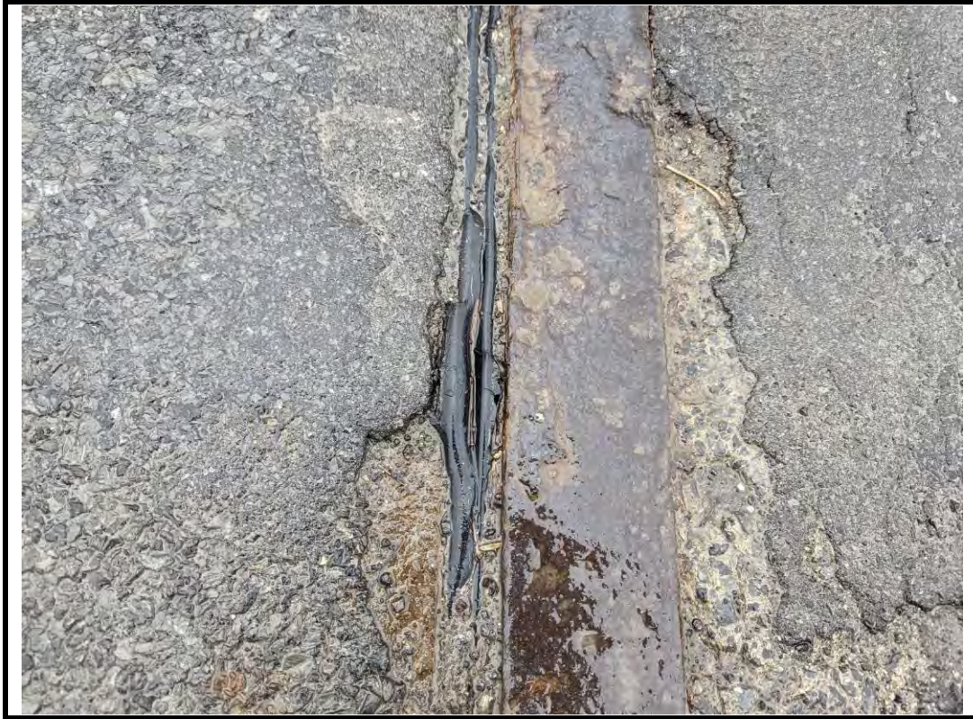
Photo 11 Rust, abrasion on armouring (typ.). Debris and failing deck seal at North
