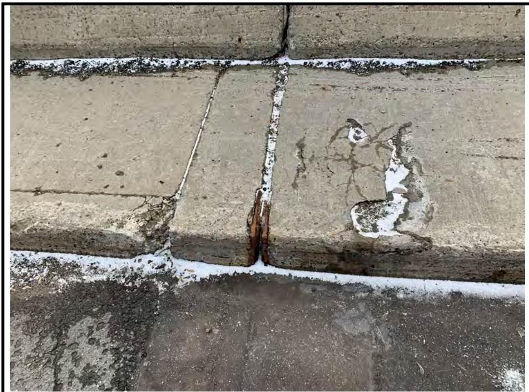
Photo 10 Spall on top face of concrete sidewalk
