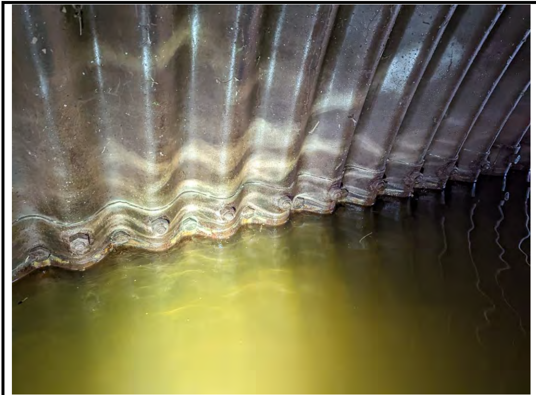
Photo 8 Section crack/splitting along boltline at East barrel wall, with coating loss
