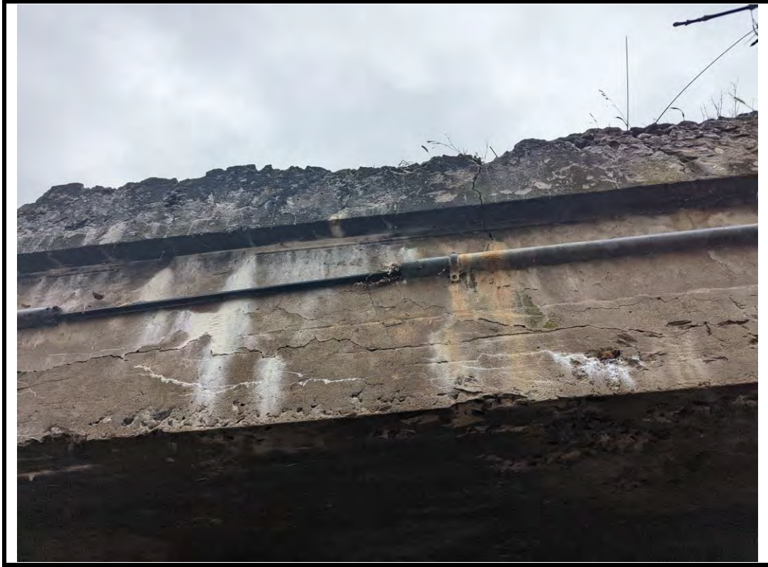
Photo 9 Cracks and efflorescence at north barrel, with spalls along deck
