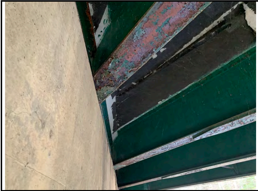
Photo 15 Corrosion and coating failure on north end of interior girder
