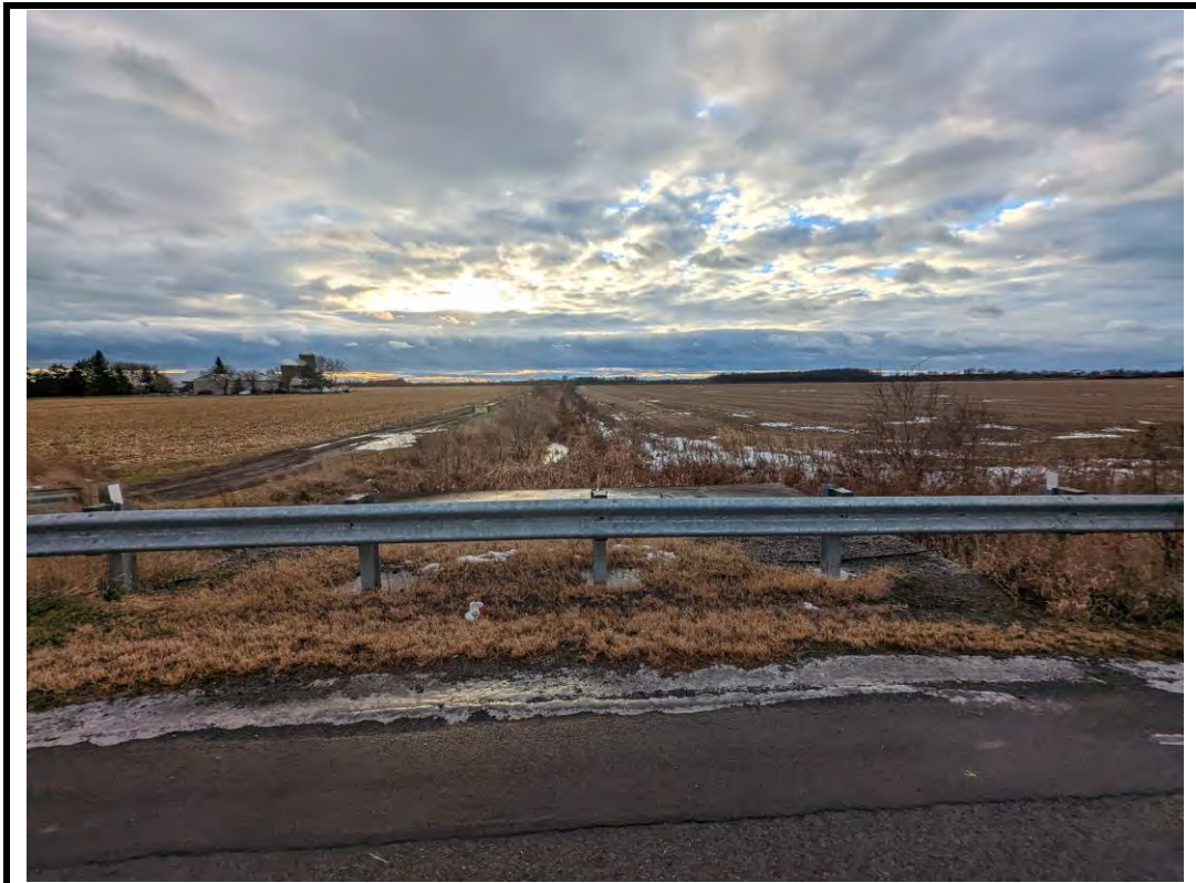
Photo 8 Ponding at barrier posts above structure
