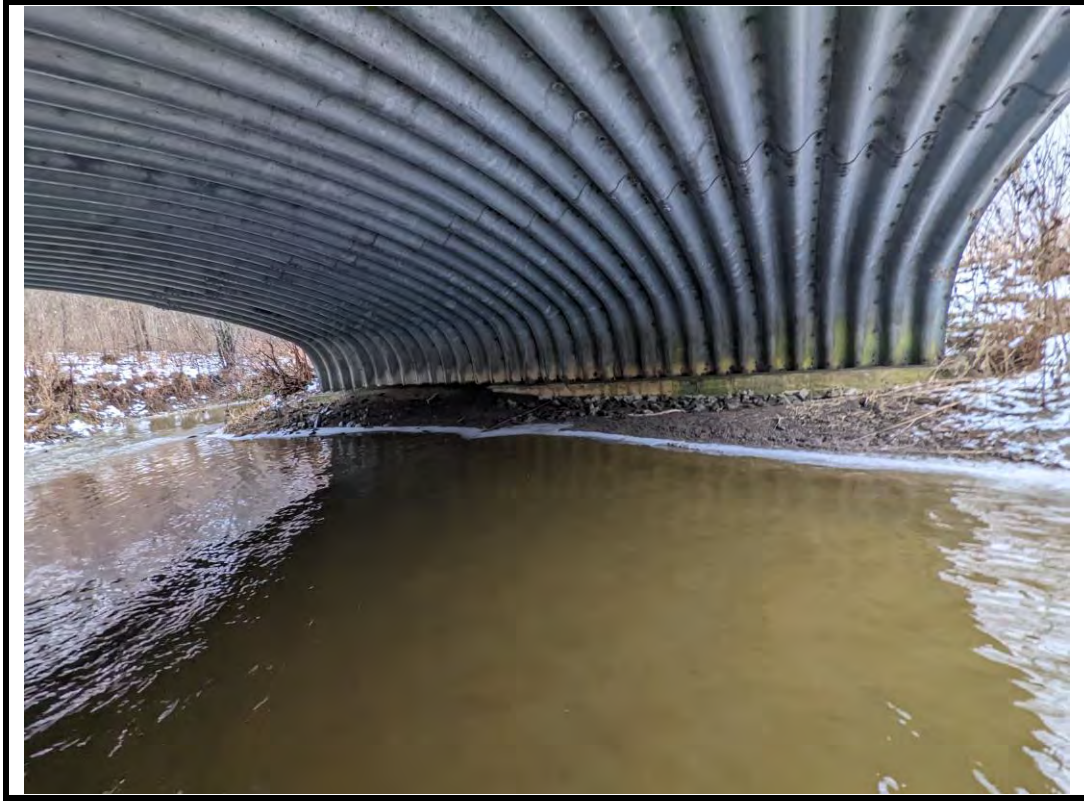
Photo 11 Sediment buildup within culvert along stream bed
