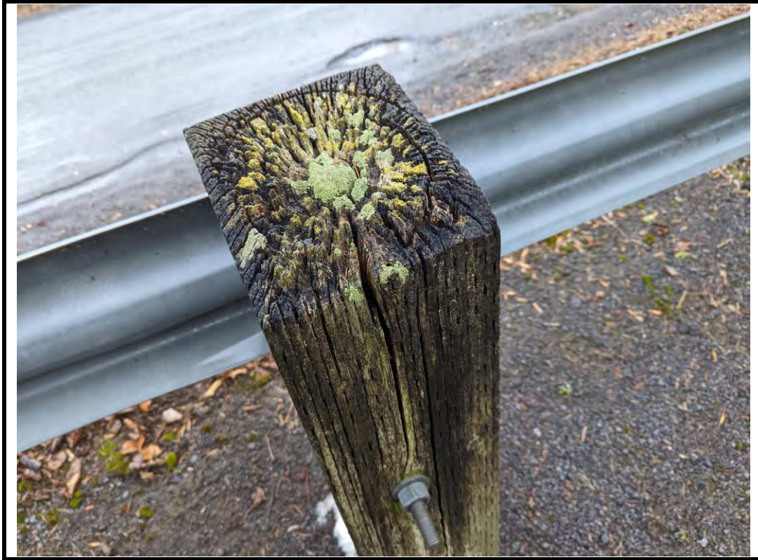
Photo 13 Rot, checks and splits at southwest approach barrier post (typ.)
