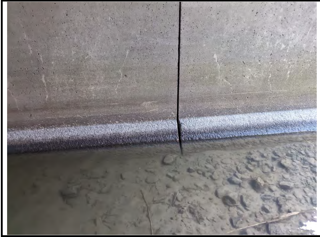
Photo 7 Light scaling along bottom haunches of culvert (typical)
