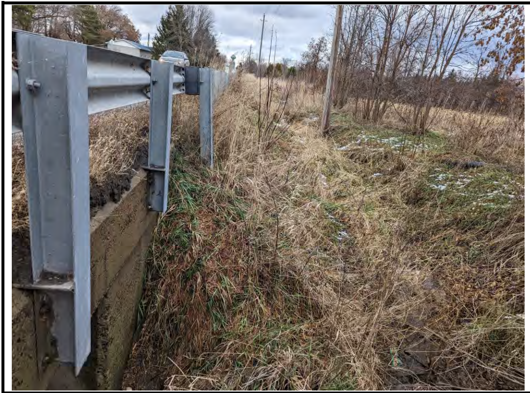
Photo 11 Disconnected/rotated barrier post and loss of fill at the southeast
