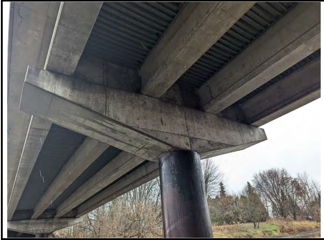
Photo 15 South pier cap, bridge soffit, and girders
