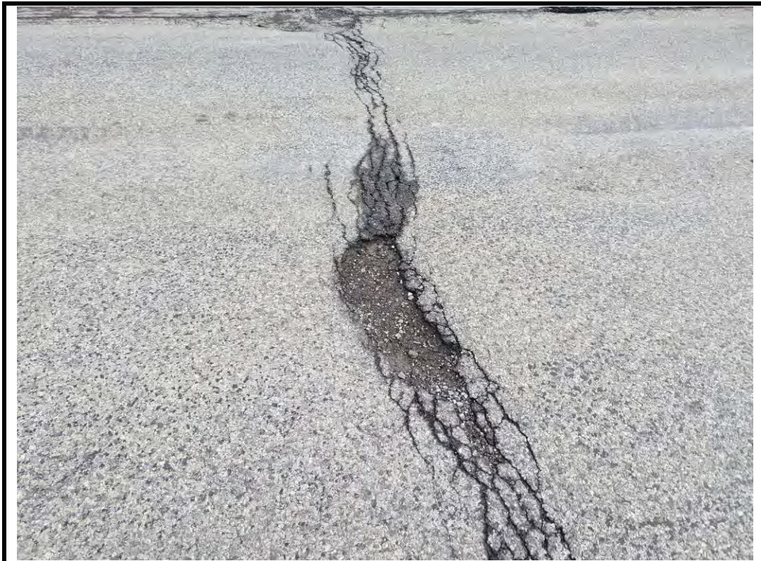
Photo 8 Medium pothole and transverse alligator cracks in approach wearing surface
