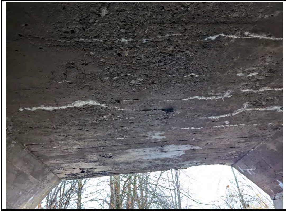
Photo 11 Efflorescence and scaling on barrel soffit (typ.)
