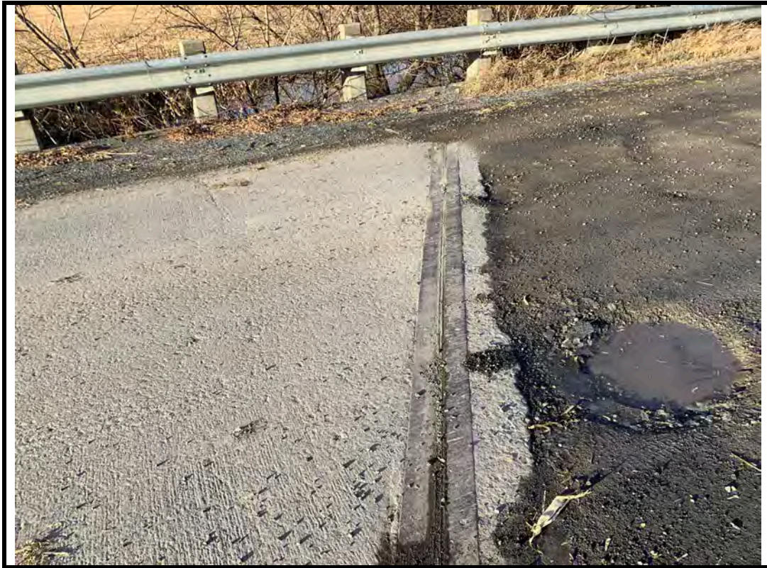
Photo 9 Abrasions noted on strip seal on east expansion joint
