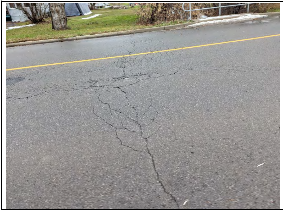
Photo 9 Map cracking on west approach wearing surface
