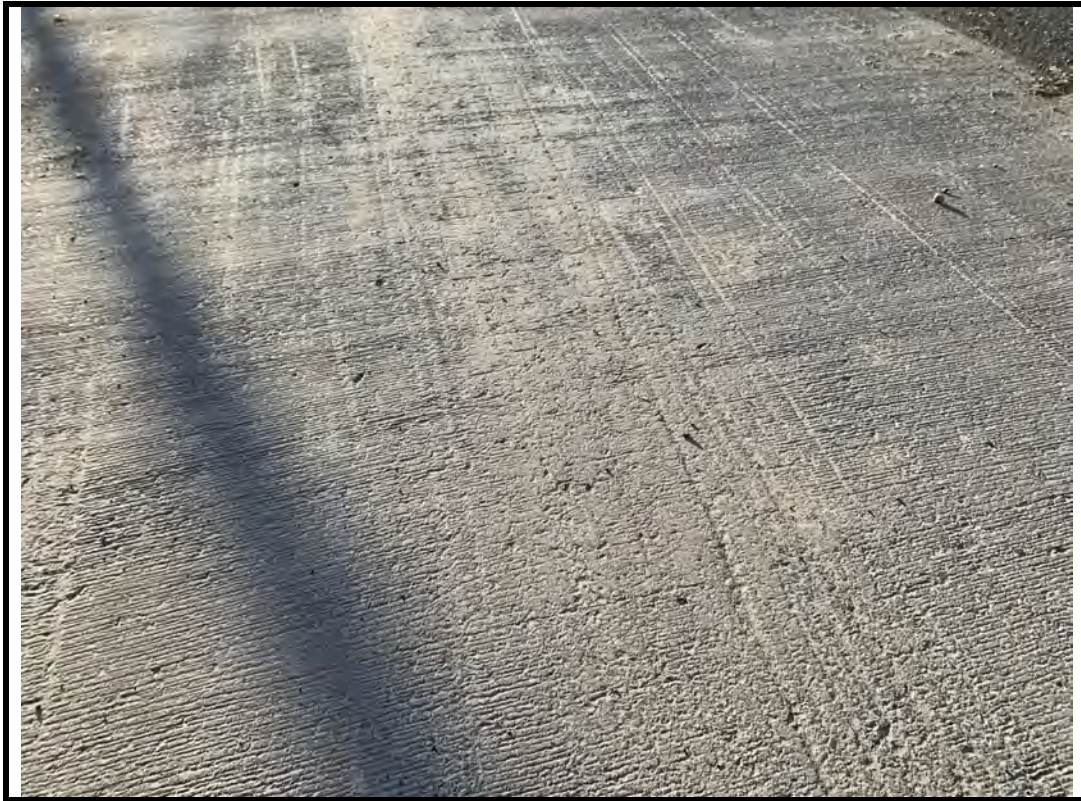
Photo 11 Abrasions and scaling on exposed concrete deck top.
