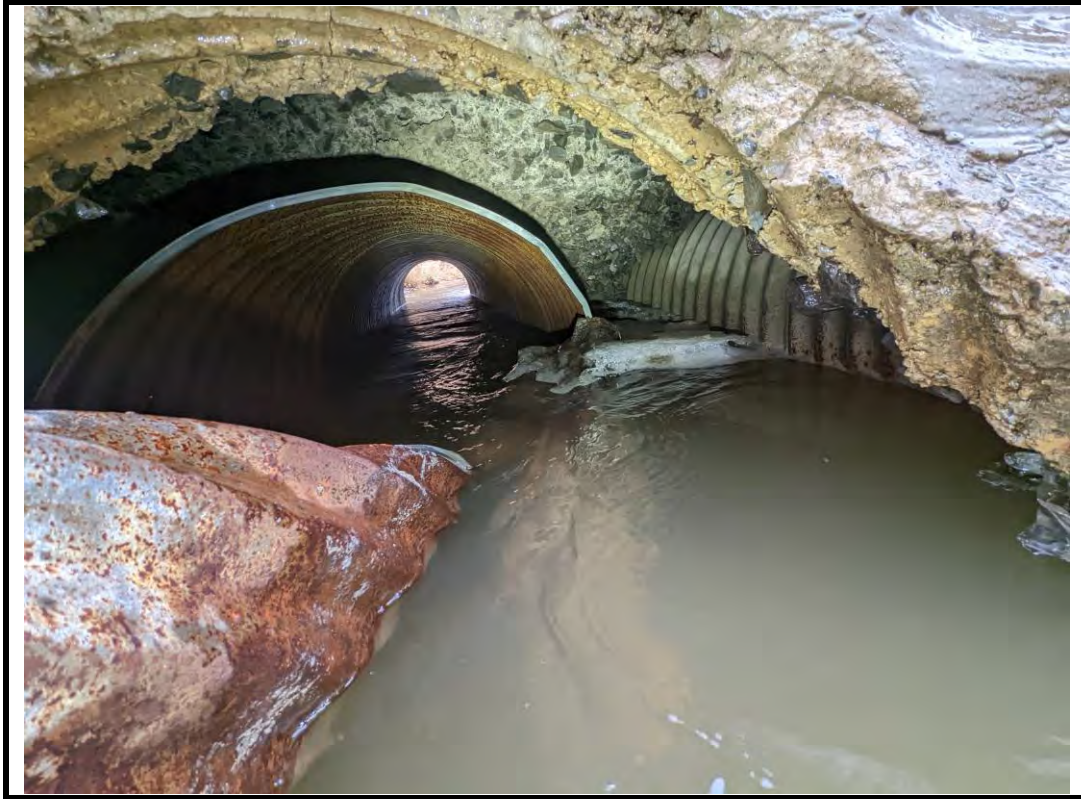
Photo 11 Separation of barrels and voids in slab around barrels on west side
