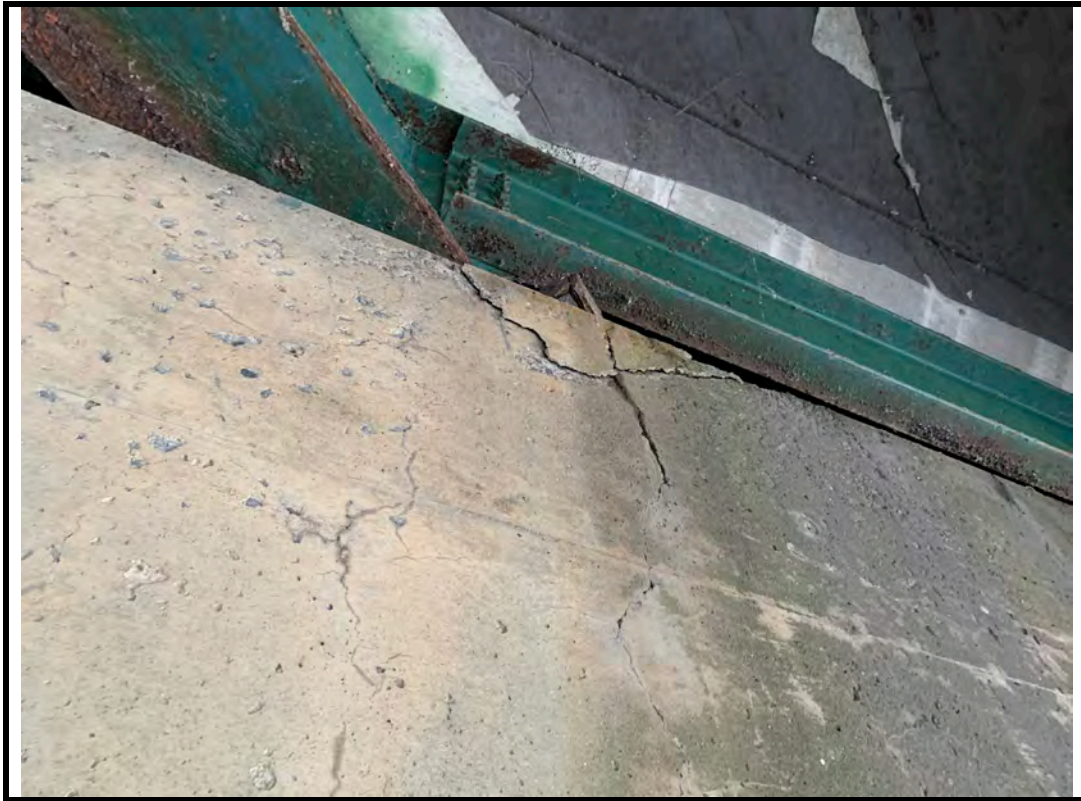
Photo 19 Delamination on south abutment wall below girder
