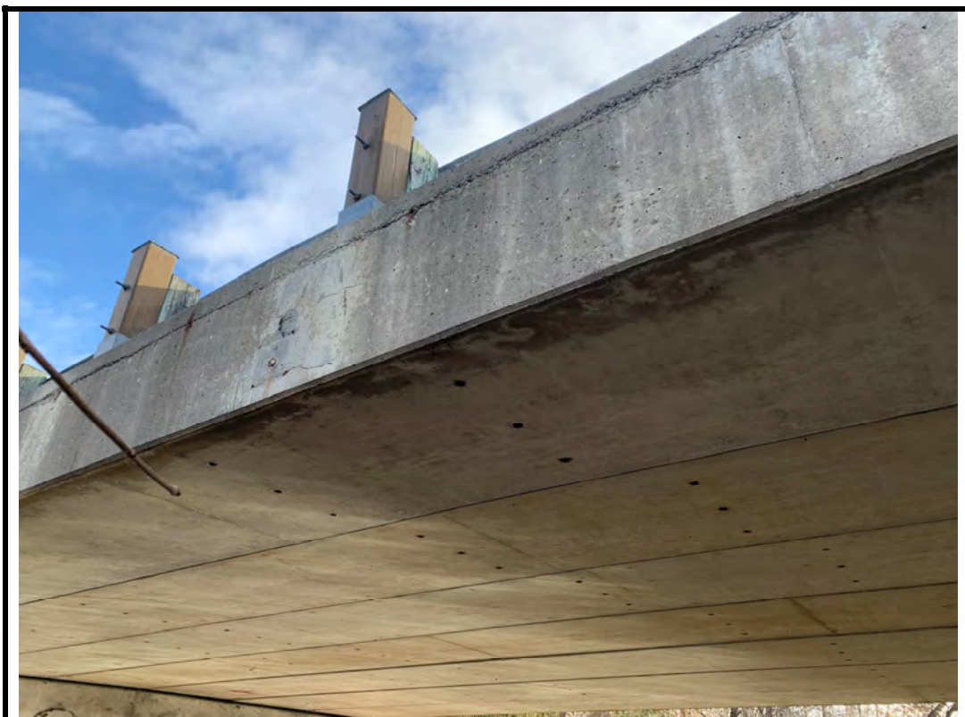
Photo 14 Staining at edges of underside of structure
