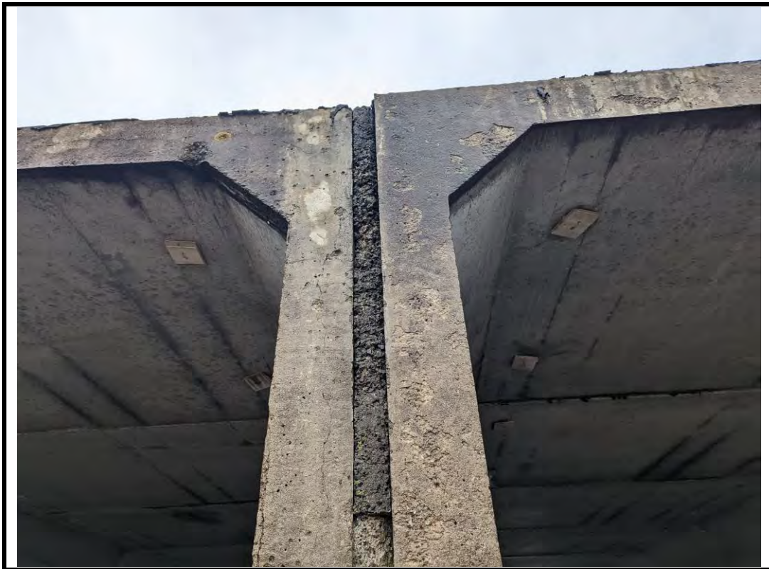
Photo 12 Scaling and cracks at west barrel ends (typical)
