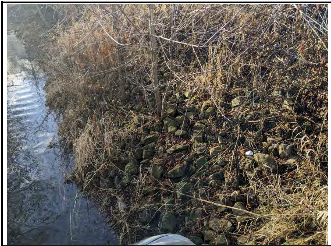
Photo 12 Rip rap slope protection at southwest embankment
