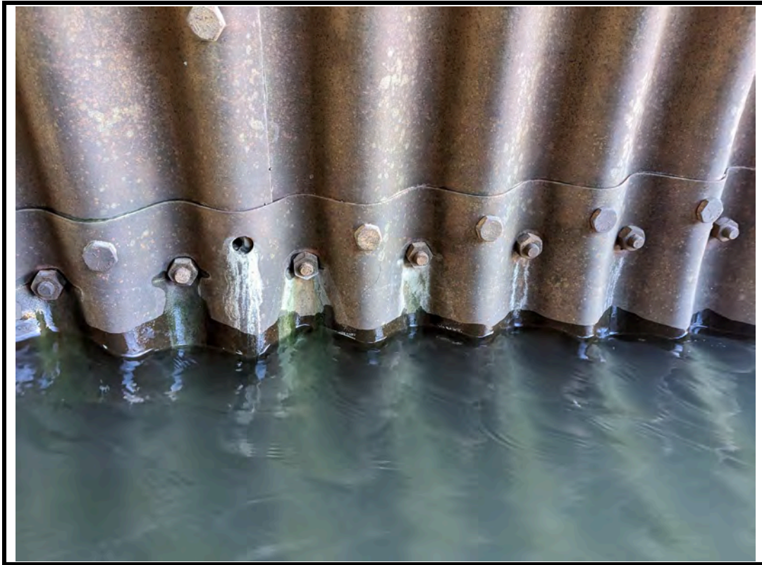
Photo 11 Evidence of leakage and efflorescence at bolt line on west barrel wall
