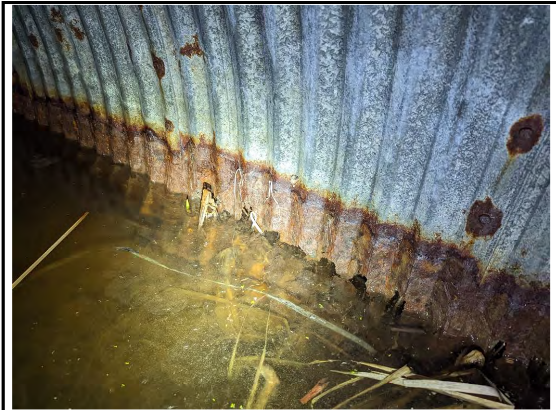
Photo 8 Severe corrosion and perforation at waterline within South barrel (typ.)
