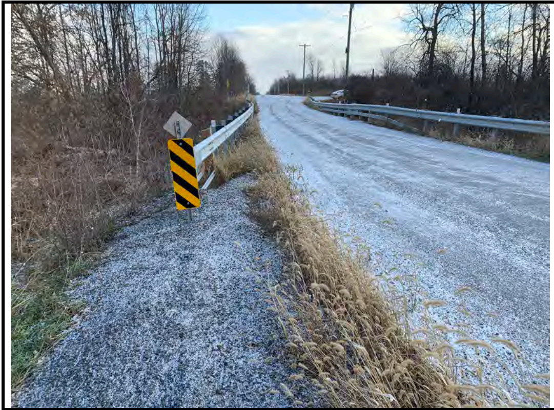
Photo 7 Typical view of approach barrier end treatment, northwest corner shown
