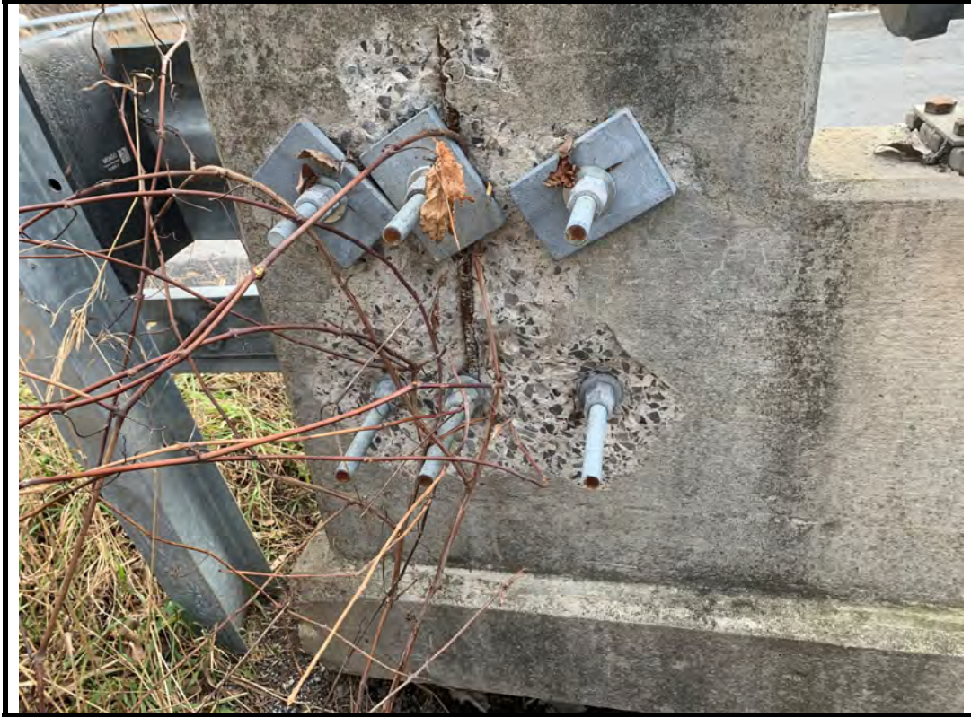
Photo 11 Spall on exterior of southwest end of barrier wall
