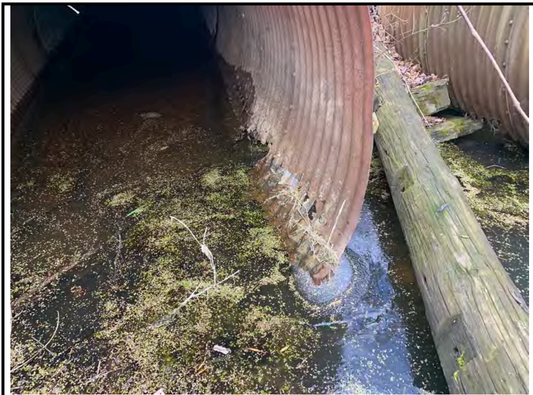
Photo 8 Severe corrosion and perforations in south barrel
