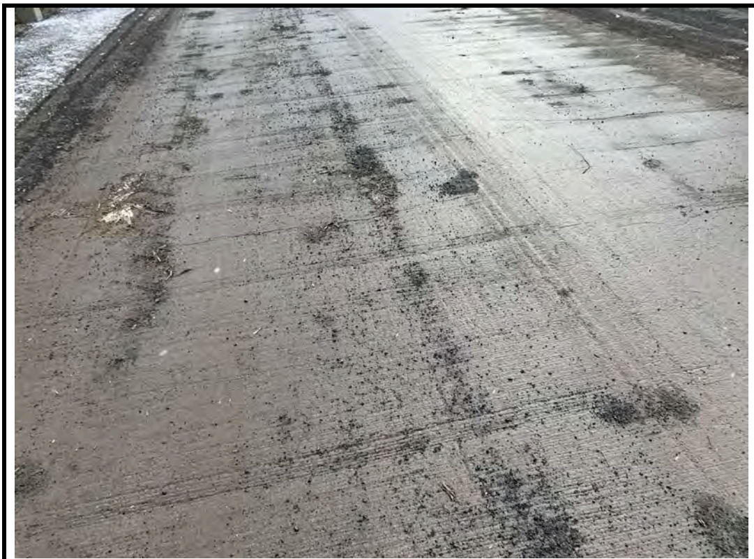
Photo 12 Wide transverse cracks and abrasions on deck top
