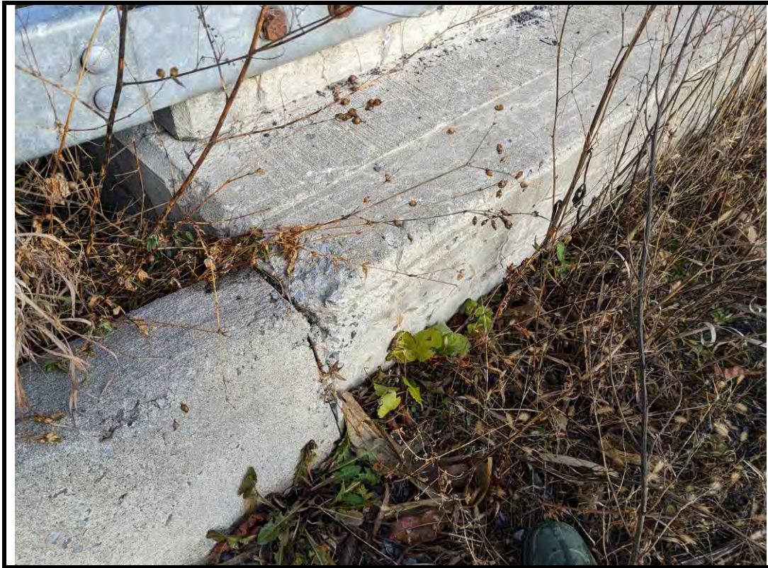
Photo 9 Spall on northwest barrier curb at transition
