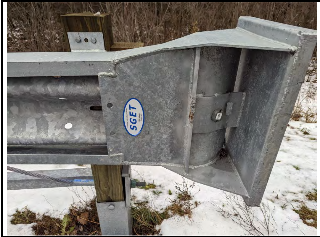
Photo 7 New approach guide rail and end treatments above structure (typ.)
