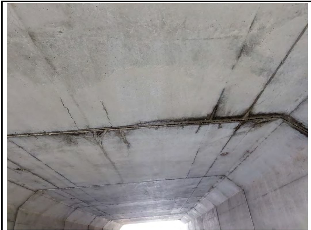
Photo 8 Leaking at second joint from the south
