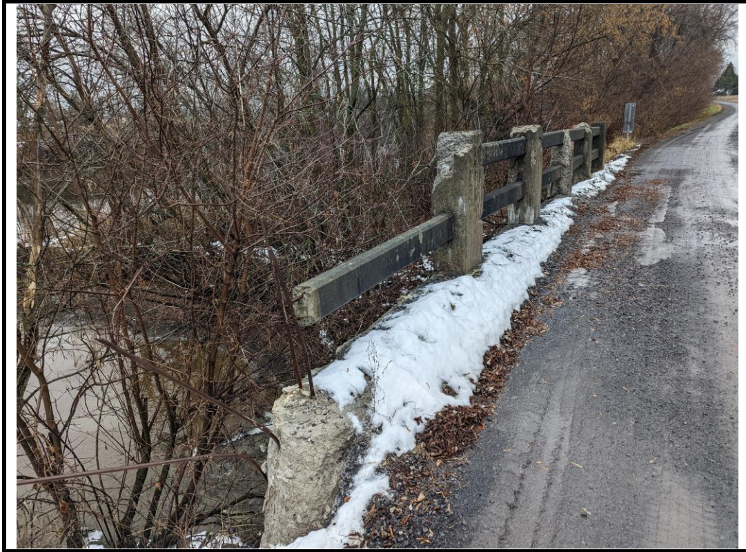
Photo 7 Deflection, section loss, spalls, ECR, and disintegration on north barrier (typ.)
