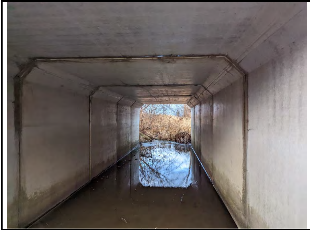
Photo 9 View through barrel and leaking at segment joints
