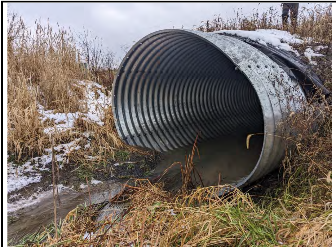
Photo 8 South culvert barrel end and encroachment of washout (inlet)
