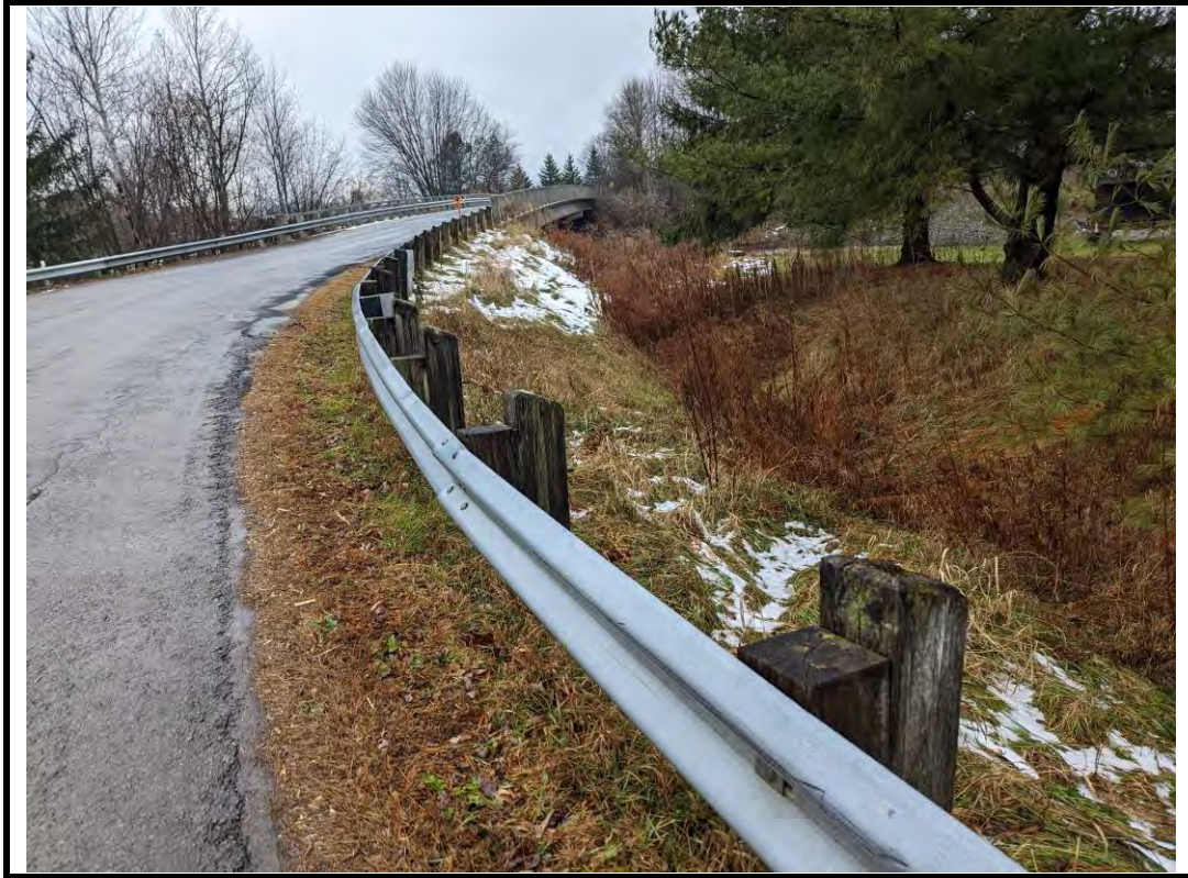
Photo 7 Abrasion and deformation on southeast approach barrier (typ.)
