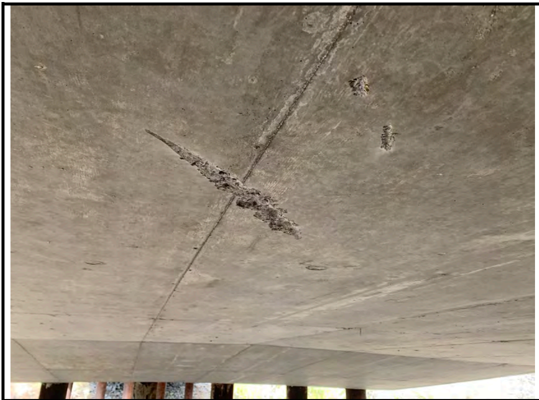
Photo 16 Small spall on south side of interior soffit
