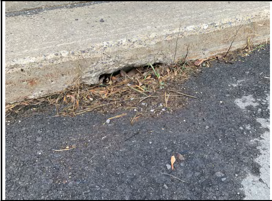
Photo 13 Debris blocking deck drain
