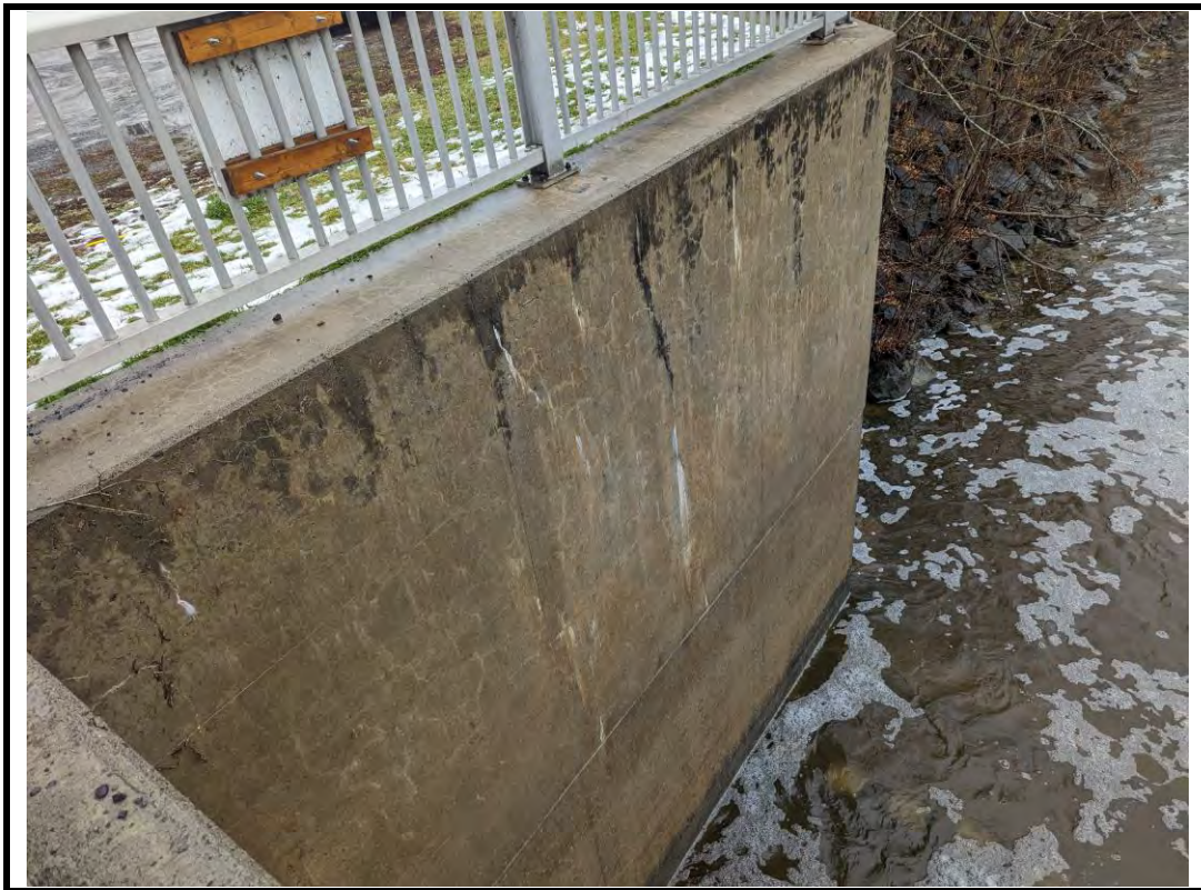
Photo 12 Map cracking on wingwalls (typical)
