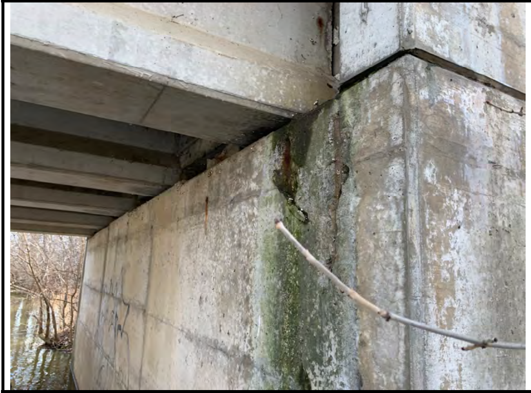
Photo 19 Staining and delamination on north end of east abutment wall
