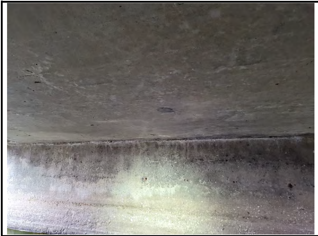
Photo 15 Scaling, wet stains, and light scour on abutment walls
