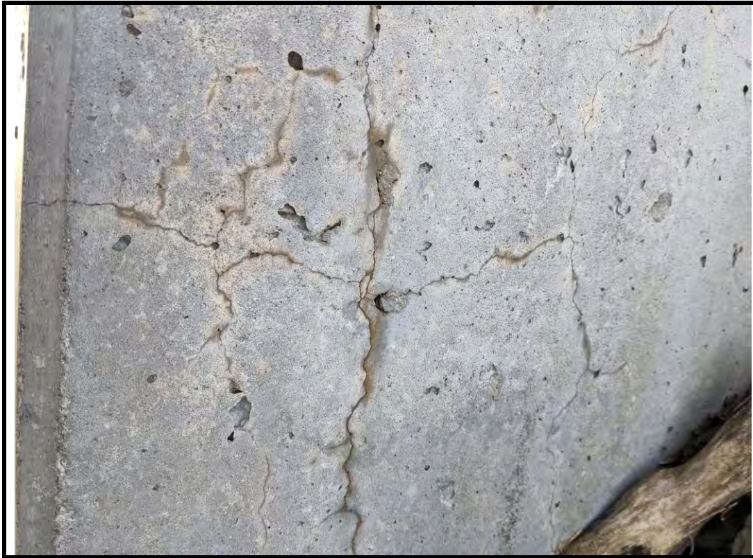
Photo 17 Cracks in northwest abutment wall
