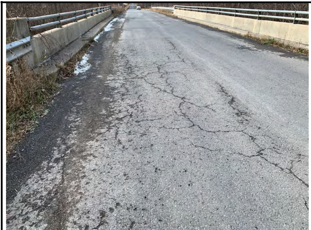
Photo 8 Medium pattern cracks on east approach wearing surface
