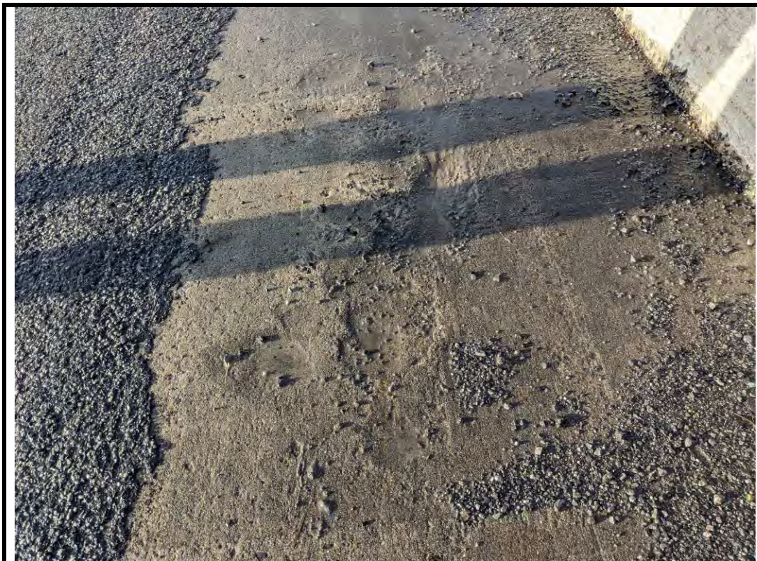
Photo 14 Exposed concrete deck top beside surface treatment
