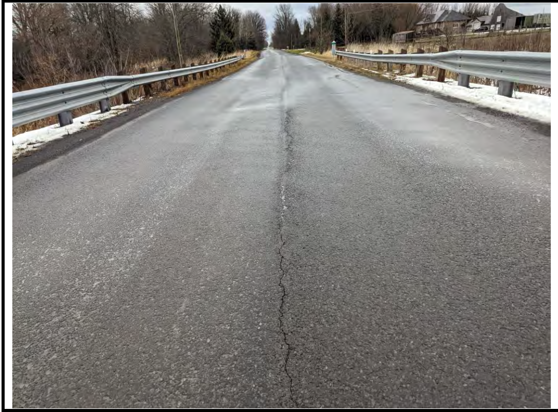
Photo 9 Medium longitudinal crack and raveling in asphalt wearing surface
