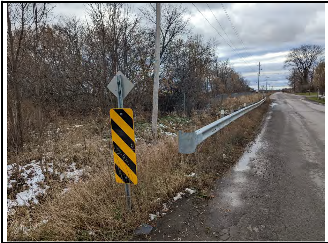
Photo 7 Structure and approach barrier and end treatment (typical)
