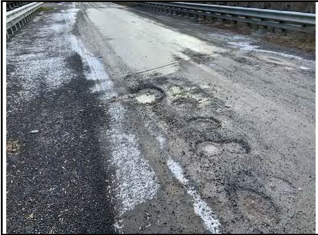
Photo 9 Large potholes on north approach
