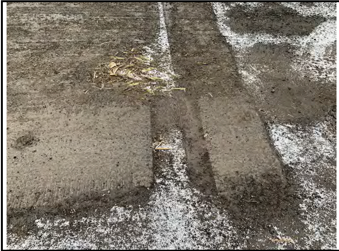
Photo 9 North expansion joint covered by debris
