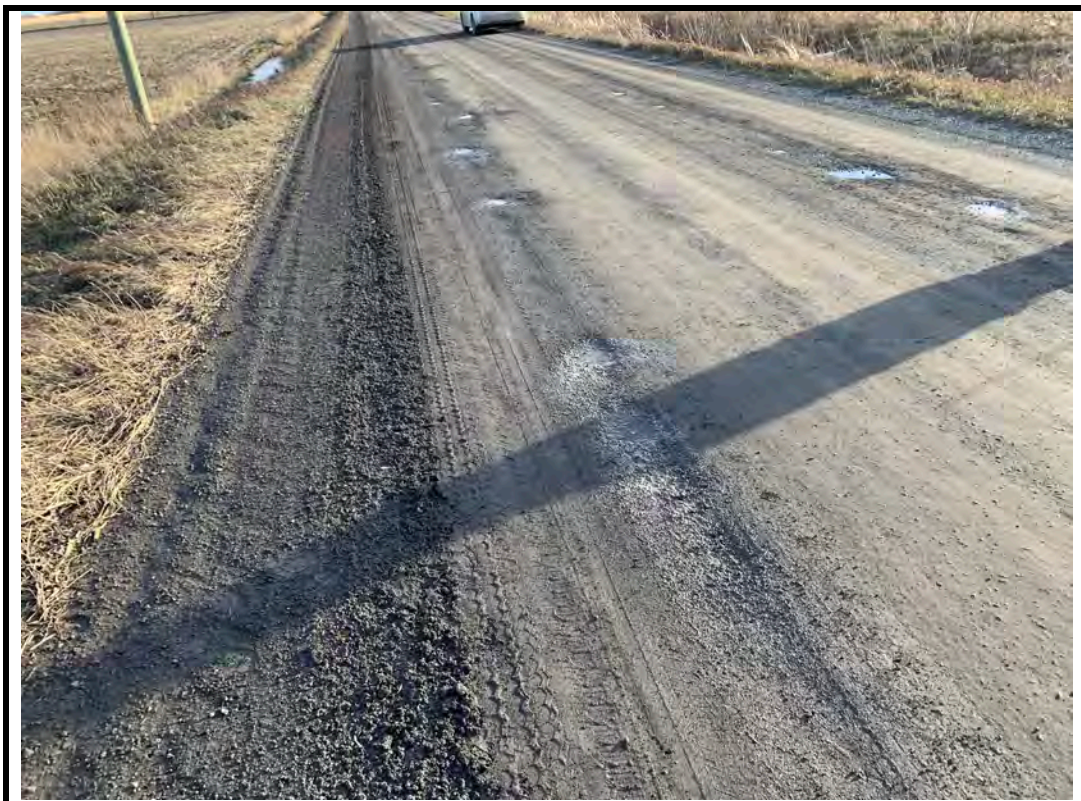
Photo 6 Potholes forming on south wearing surface
