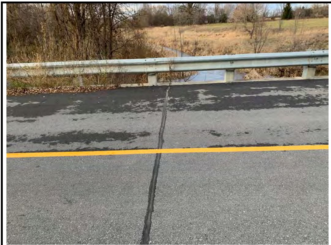
Photo 10 New asphalt at west end of deck wearing surface
