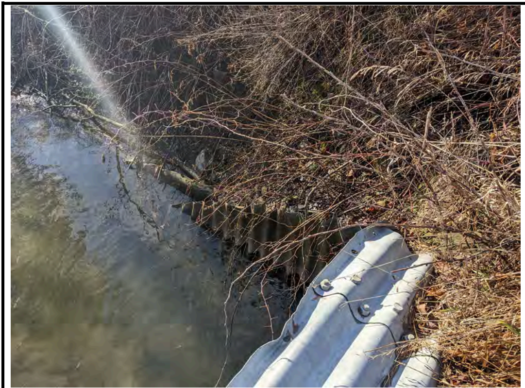
Photo 12 Erosion and washout noted on southwest embankment
