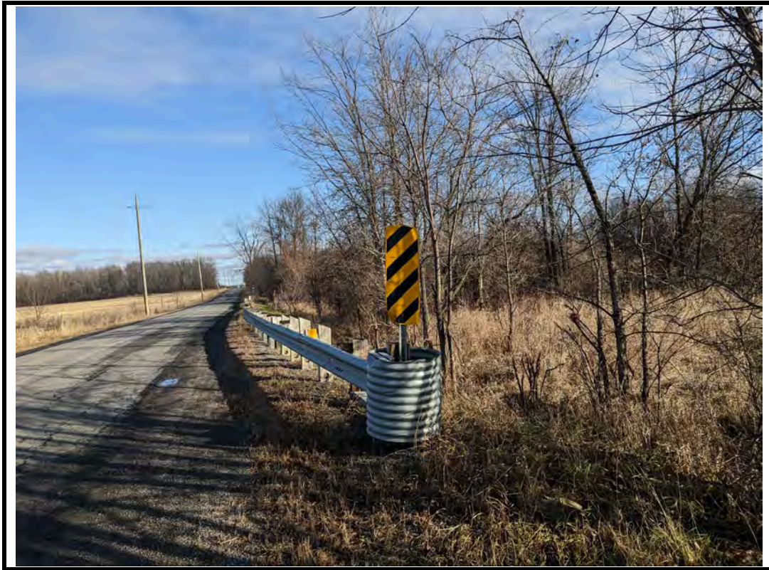
Photo 7 Eccentric end loader at southwest corner of approach
