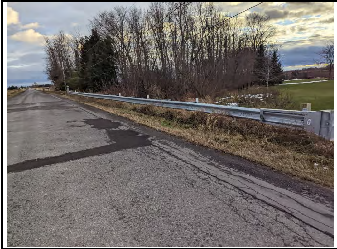
Photo 7 Longitudinal alligator cracks, with patches and raveling on wearing surface
