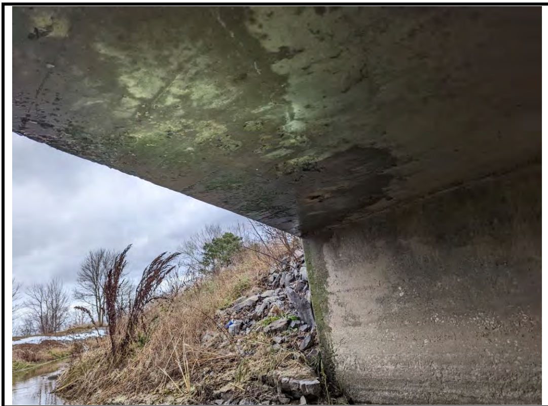
Photo 14 Scaling and wet stains on deck soffit
