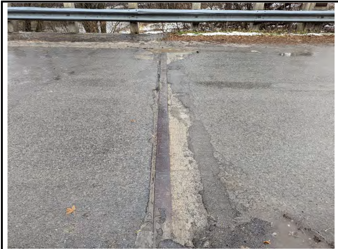
Photo 10 Partially covered expansion joint at north (typ.)
