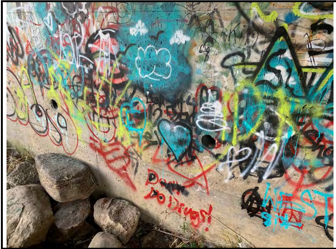
Photo 19 Scaling and graffiti around drains on abutment wall
