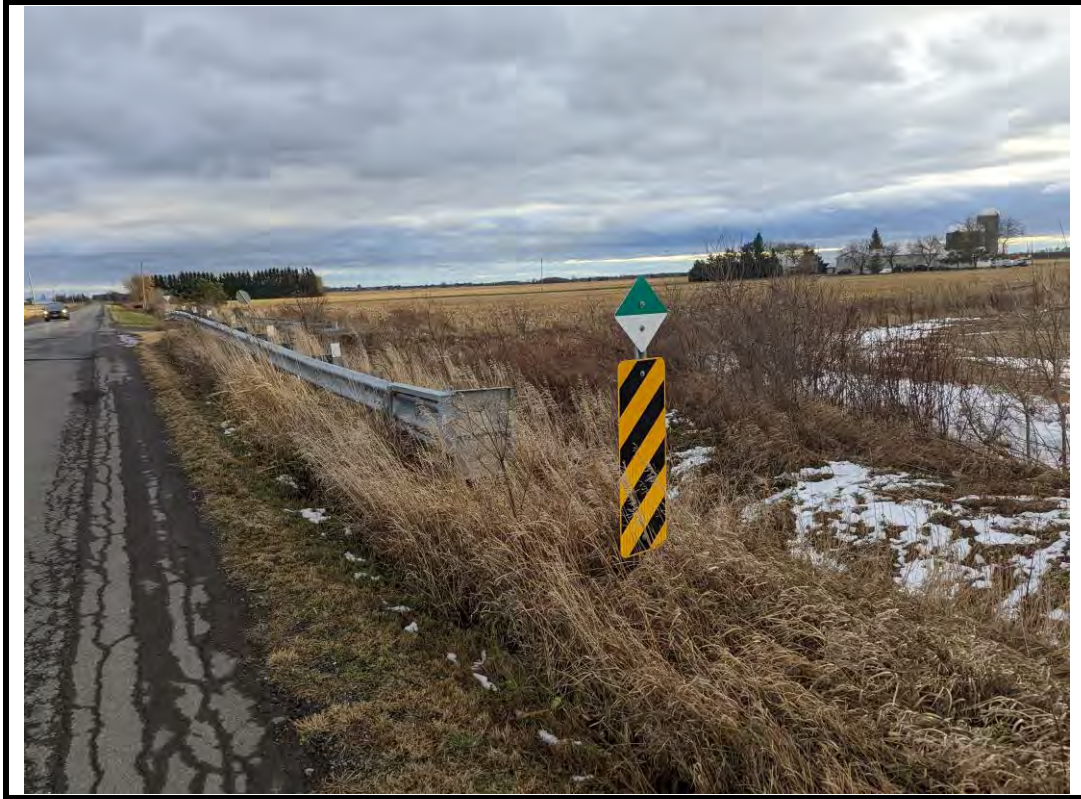
Photo 7 Replaced barrier and end-treatment (typical)
