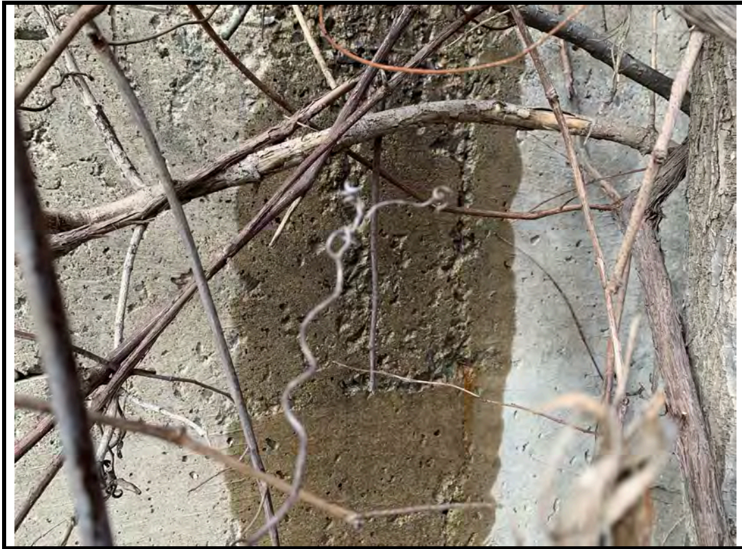
Photo 15 Scaling on north abutment wall
