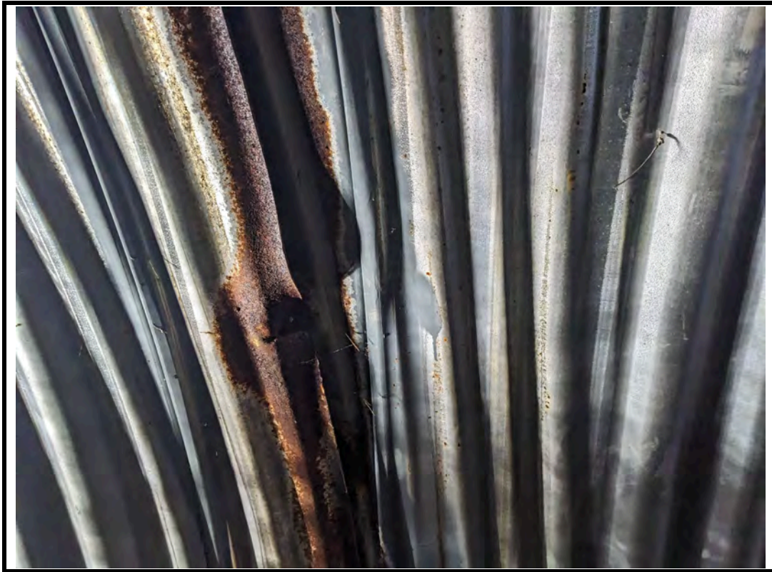
Photo 11 Minor separation at plate connection at south end of barrel
