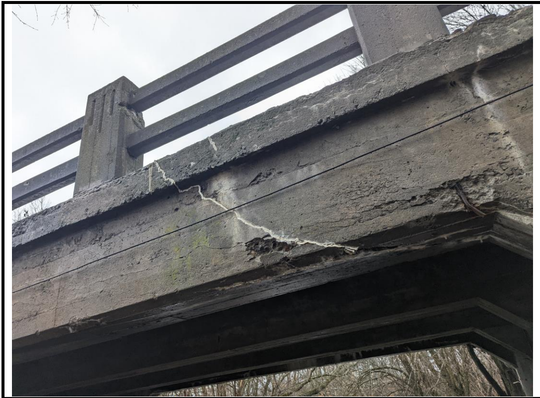
Photo 14 Cracks, scaling, spalls, and ECR on South fascia (typ.)
