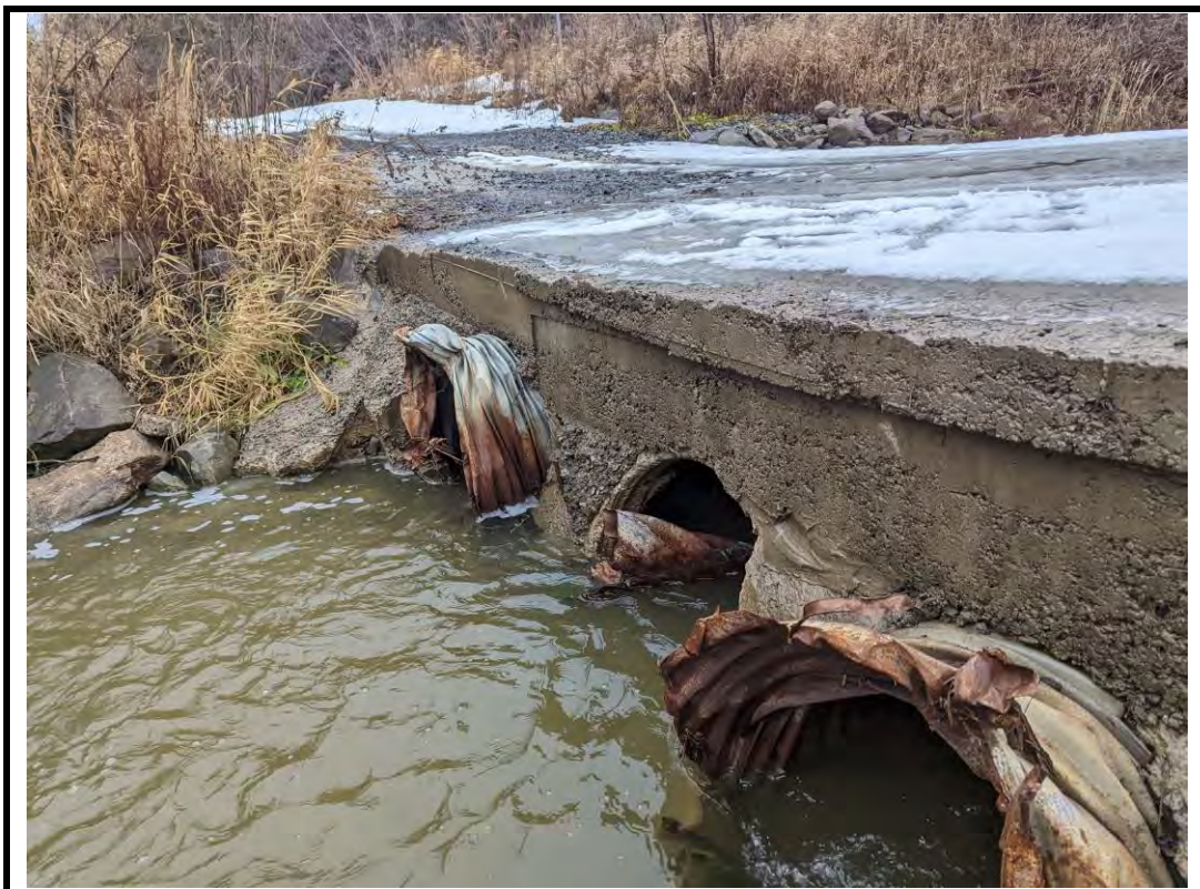
Photo 10 Severe deformations on west ends of barrels, and scaling on concrete deck
