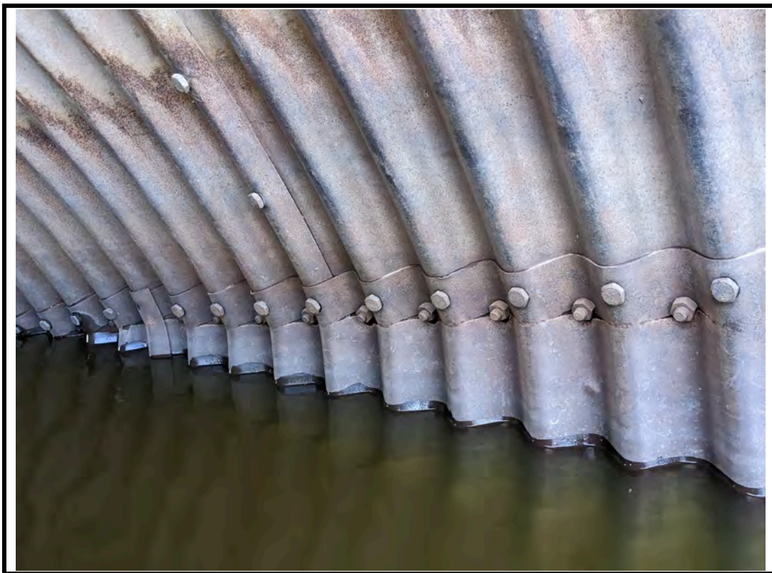
Photo 11 Wide horizontal cracks at bolt line at northeast corner of barrel
