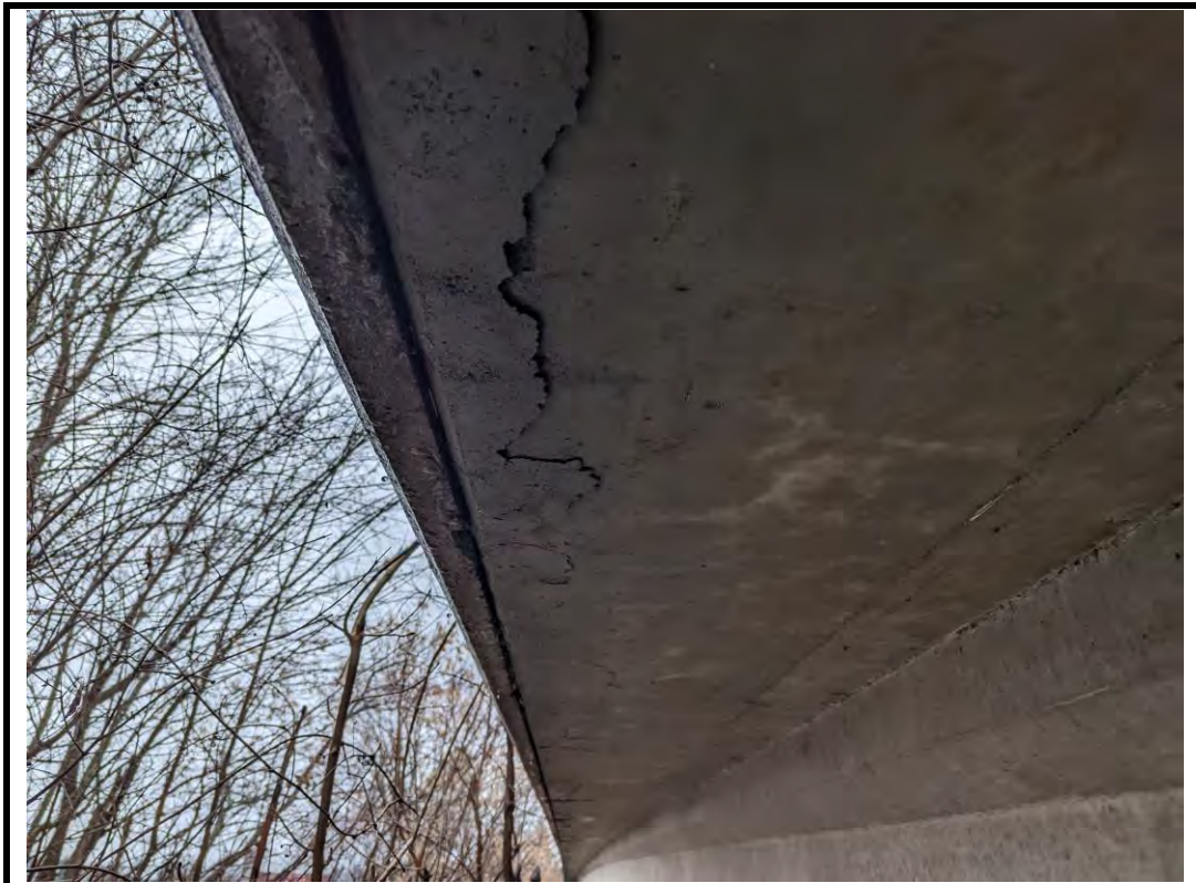
Photo 14 Delamination along west soffit overhang (typ.)
