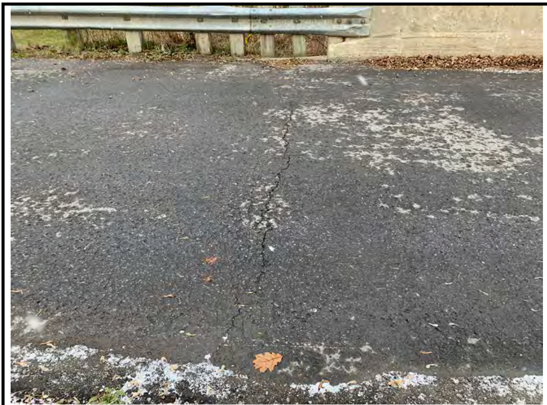
Photo 8 Wide crack on south approach wearing surface
