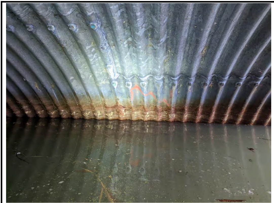
Photo 12 Corrosion on pipe arch walls (typ.)
