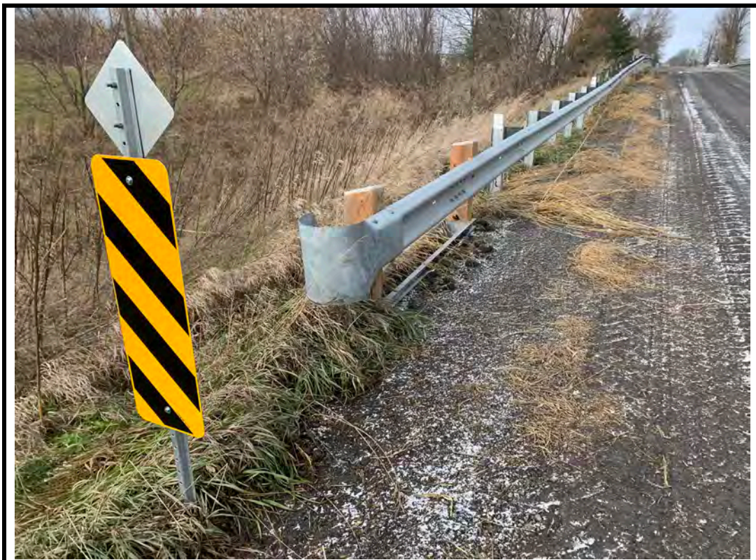
Photo 8 New end treatment at southwest corner
