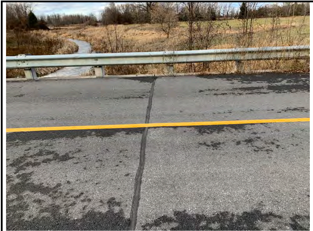
Photo 8 Seal at east end of structure
