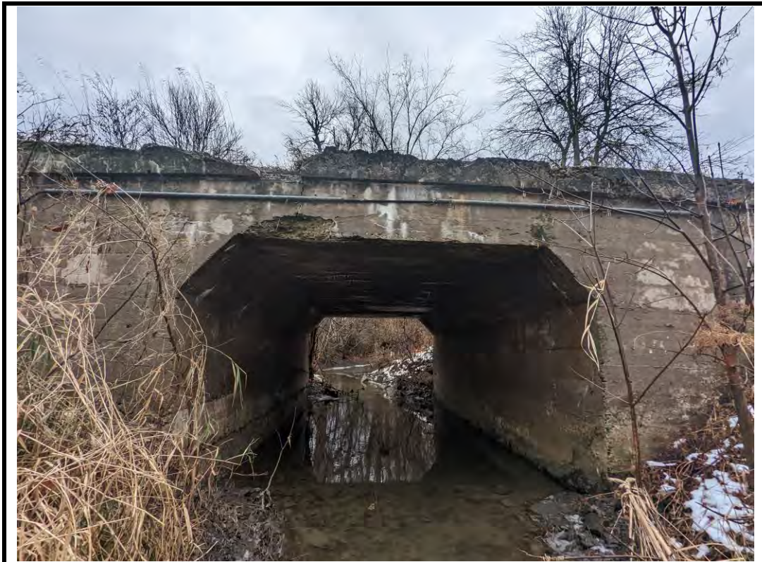
Photo 8 Spalling, honeycombing, and efflorescence at north end of barrel (Typ.)
