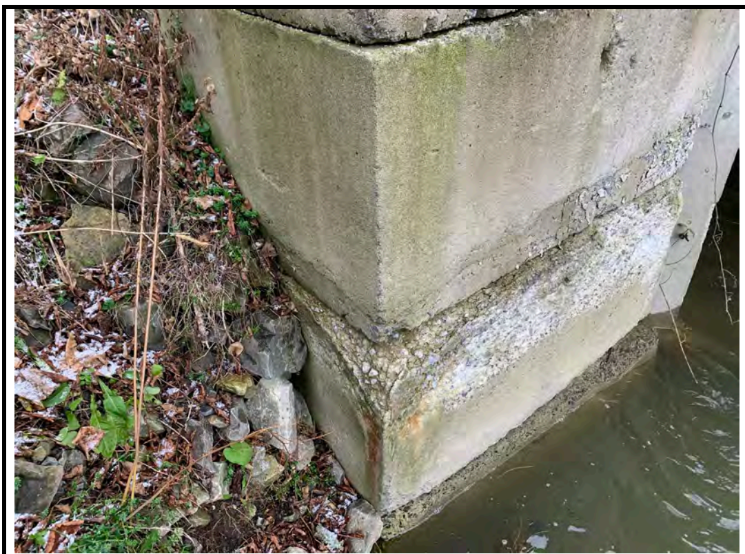
Photo 8 Disintegration on southeast block wall
