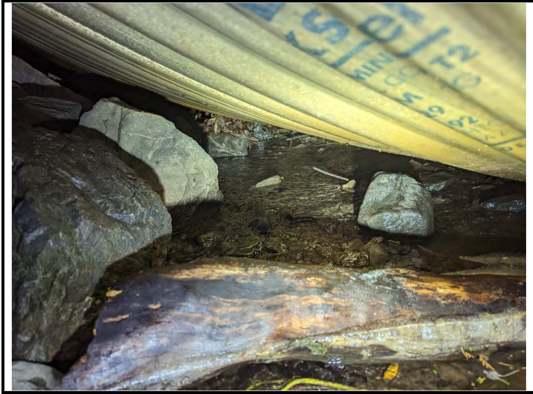
Photo 11 Undermining below south pipe segment
