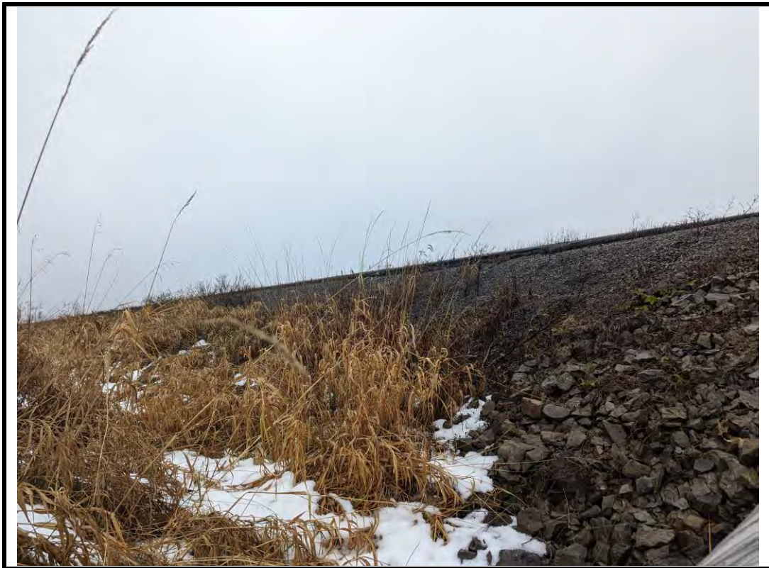
Photo 12 Light loss of Rip Rap at southwest embankment
