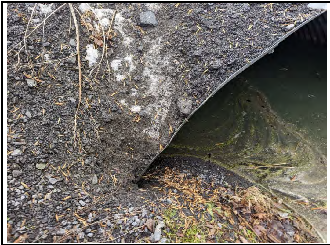
Photo 11 Erosion and encroachment into barrel at the northwest
