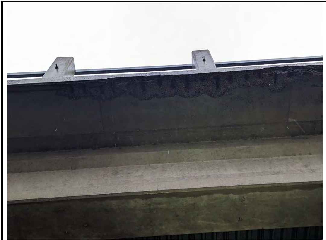
Photo 20 Spalls and ECR at northeast overhang (typ.)
