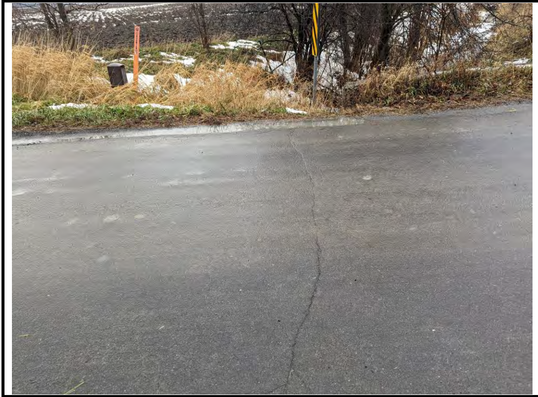
Photo 7 Transverse crack in asphalt approach wearing surface above structure
