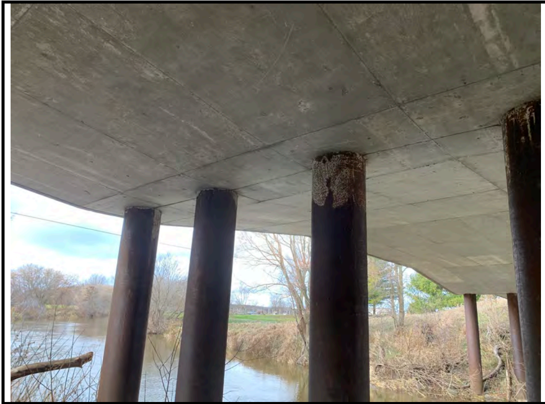
Photo 21 Staining on top of pier shafts
