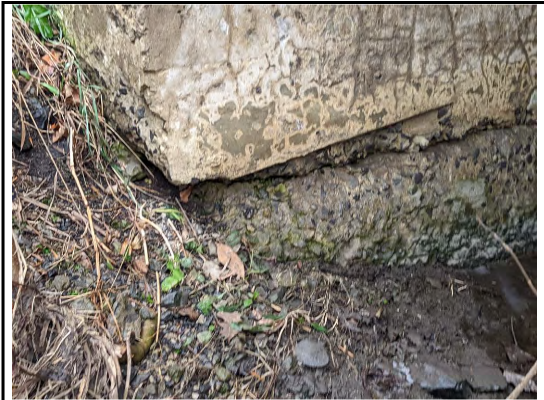
Photo 10 Scour/ severe scaling along concrete barrel walls (typ.)
