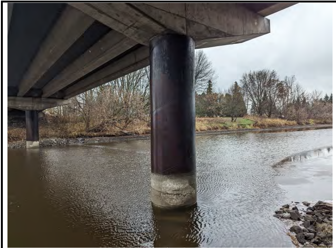
Photo 16 Steel frame pier shaft at South end of bridge
