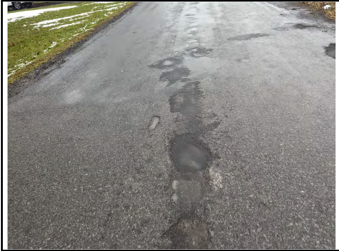
Photo 7 Small potholes forming on asphalt wearing surface above structure
