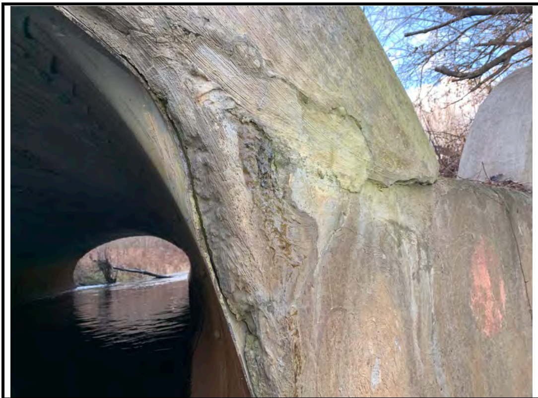
Photo 10 Spall on north concrete wall
