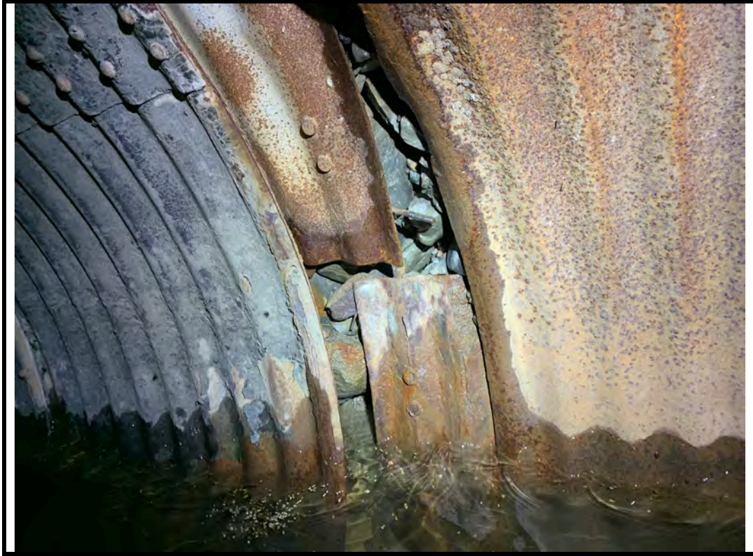
Photo 13 Separation of seam in north barrel
