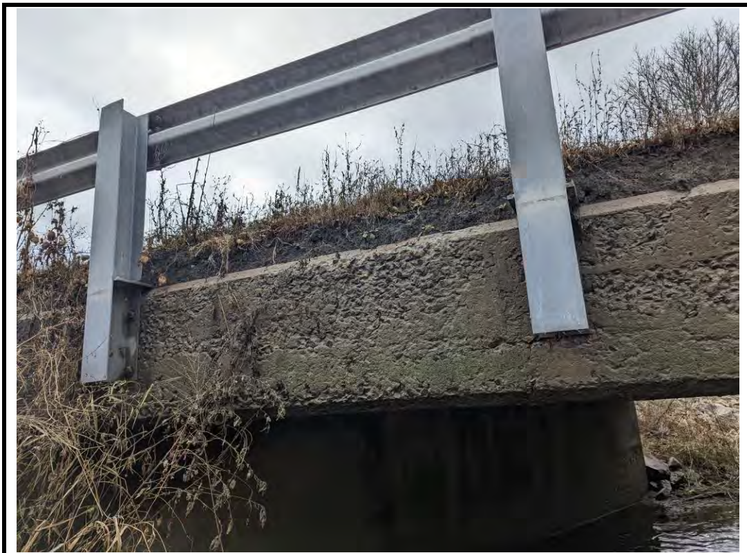
Photo 12 Scaling on deck soffit exterior/fascia (typ.)
