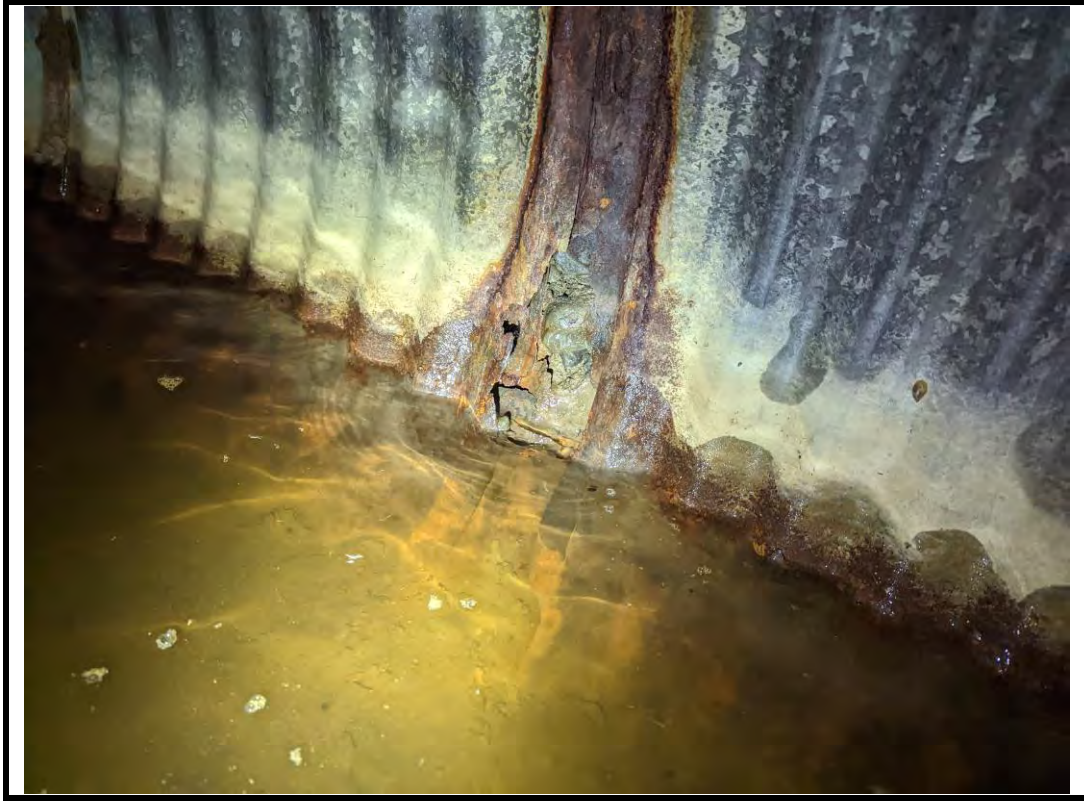
Photo 9 Perforation, corrosion, and sedimentation at midspan of South barrel
