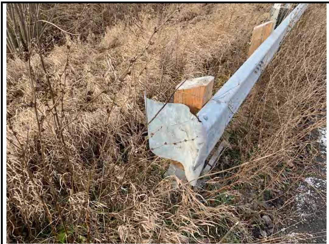
Photo 8 Collision damage at southwest end treatment
