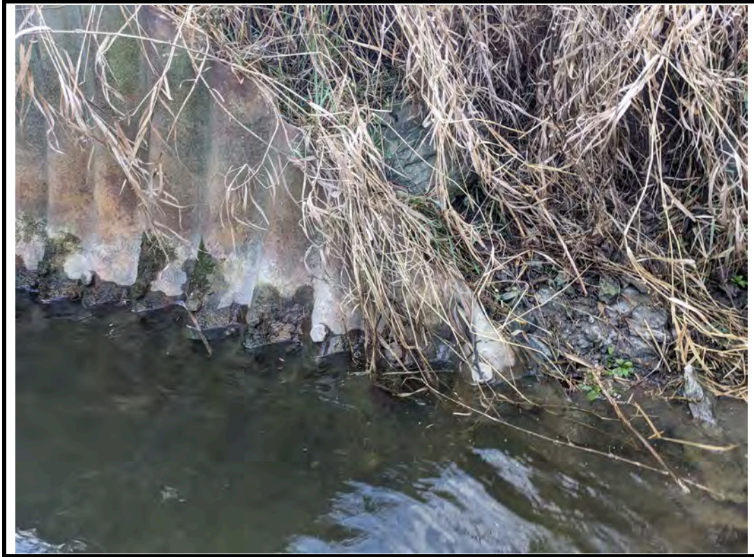
Photo 11 Erosion at northwest embankment
