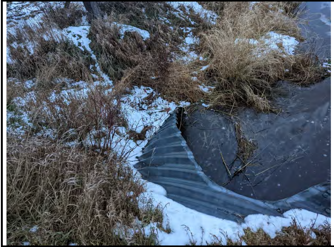
Photo 9 Loss of Rip-Rap at embankments (Typical)
