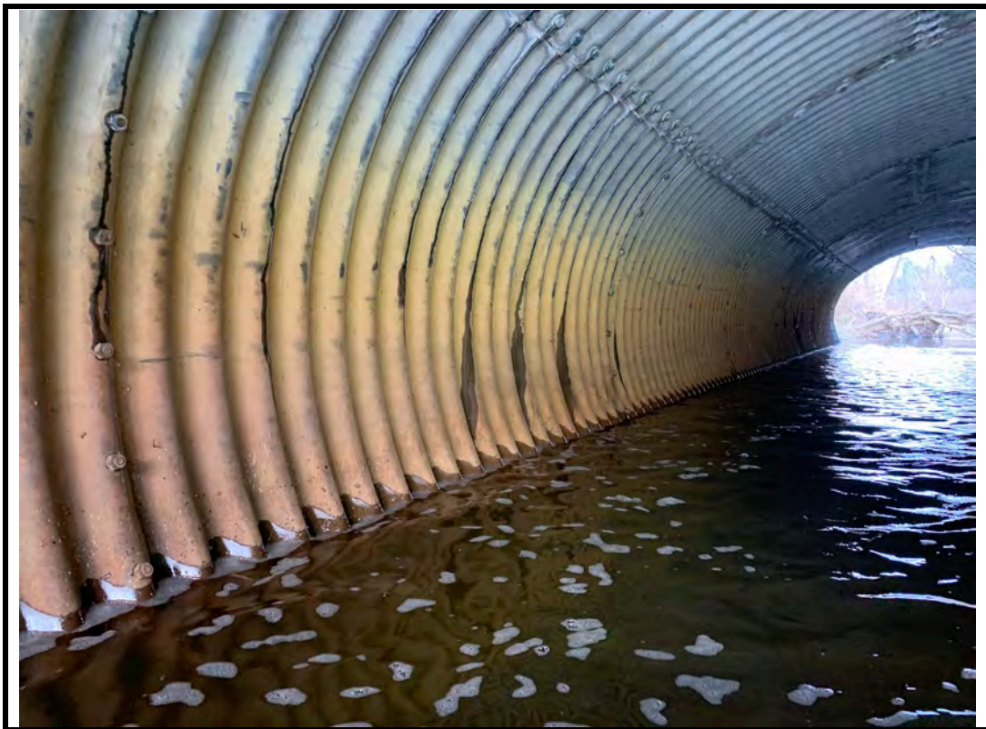
Photo 12 Wet areas and evidence of leaking in west barrel
