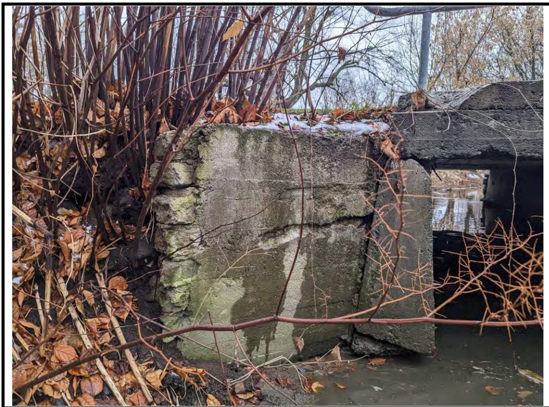
Photo 10 Scaling, degradation, and spalls on SW concrete retaining wall
