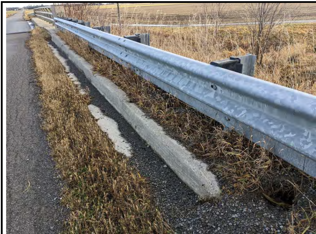
Photo 8 Vegetation and aggradation at southwest approach (typical)
