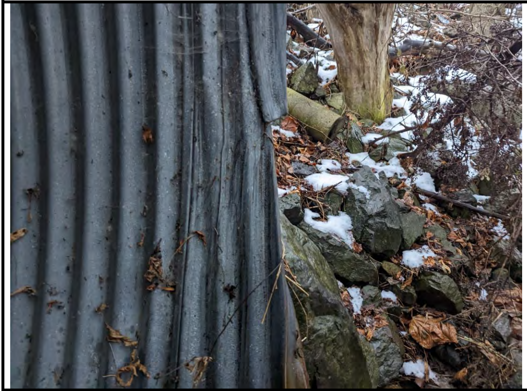
Photo 9 Light deformation at east barrel end
