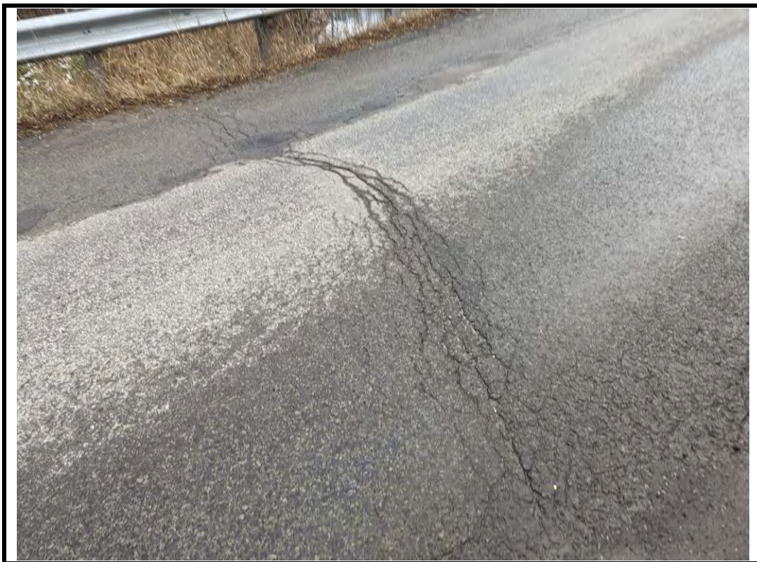
Photo 8 Transverse cracks, patched potholes, and raveling on wearing surface
