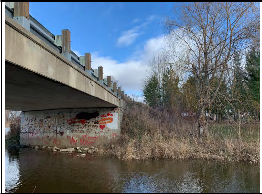
Photo 19 Moderate erosion at southeast embankment
