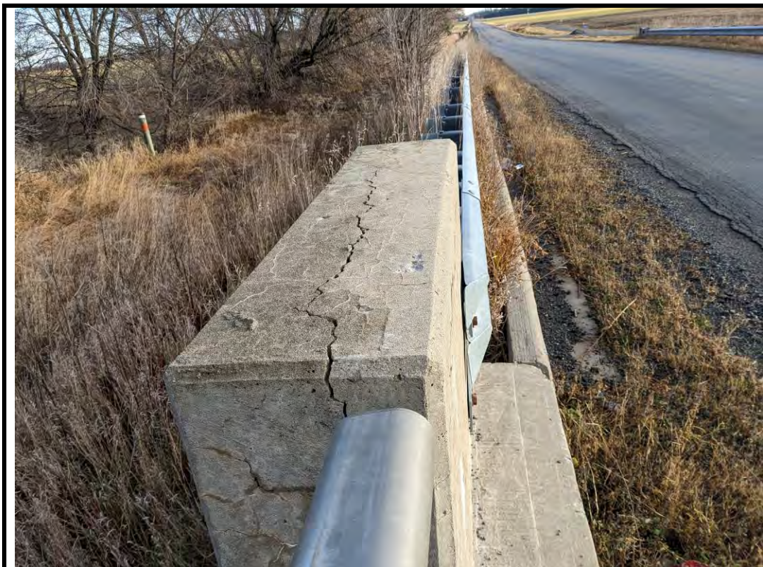
Photo 12 Wide crack at northeast barrier end wall
