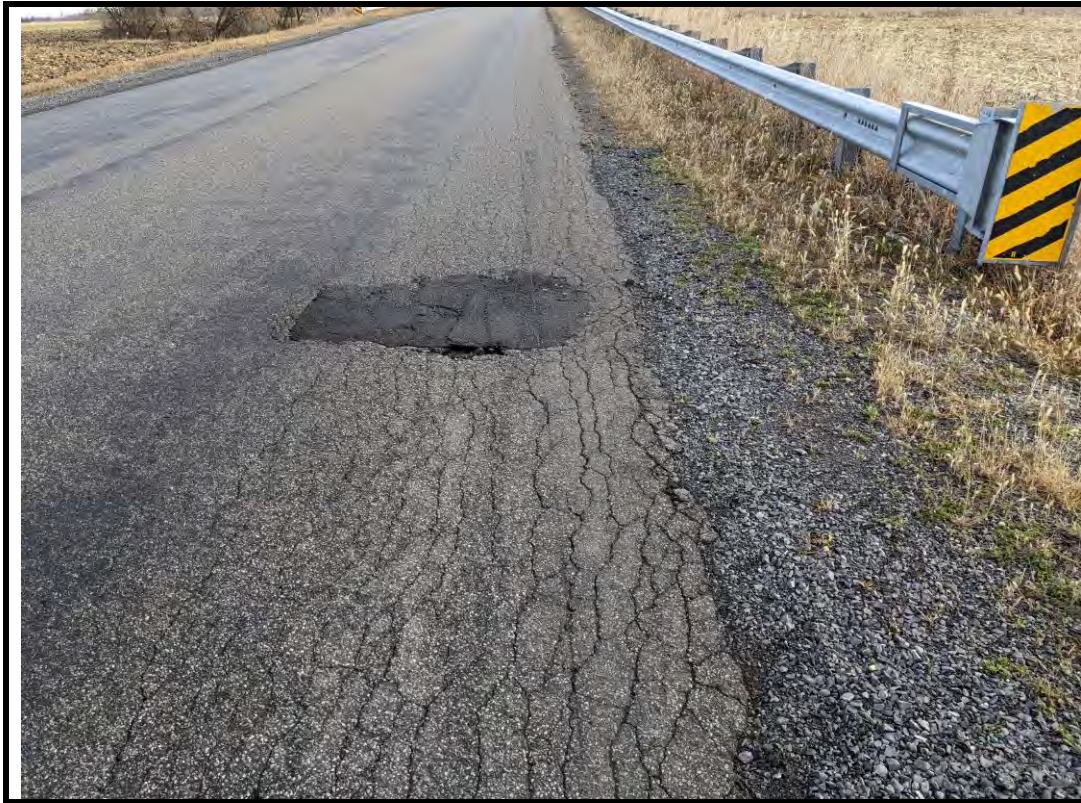
Photo 7 Pothole, patch, and crack at southwest approach wearing surface
