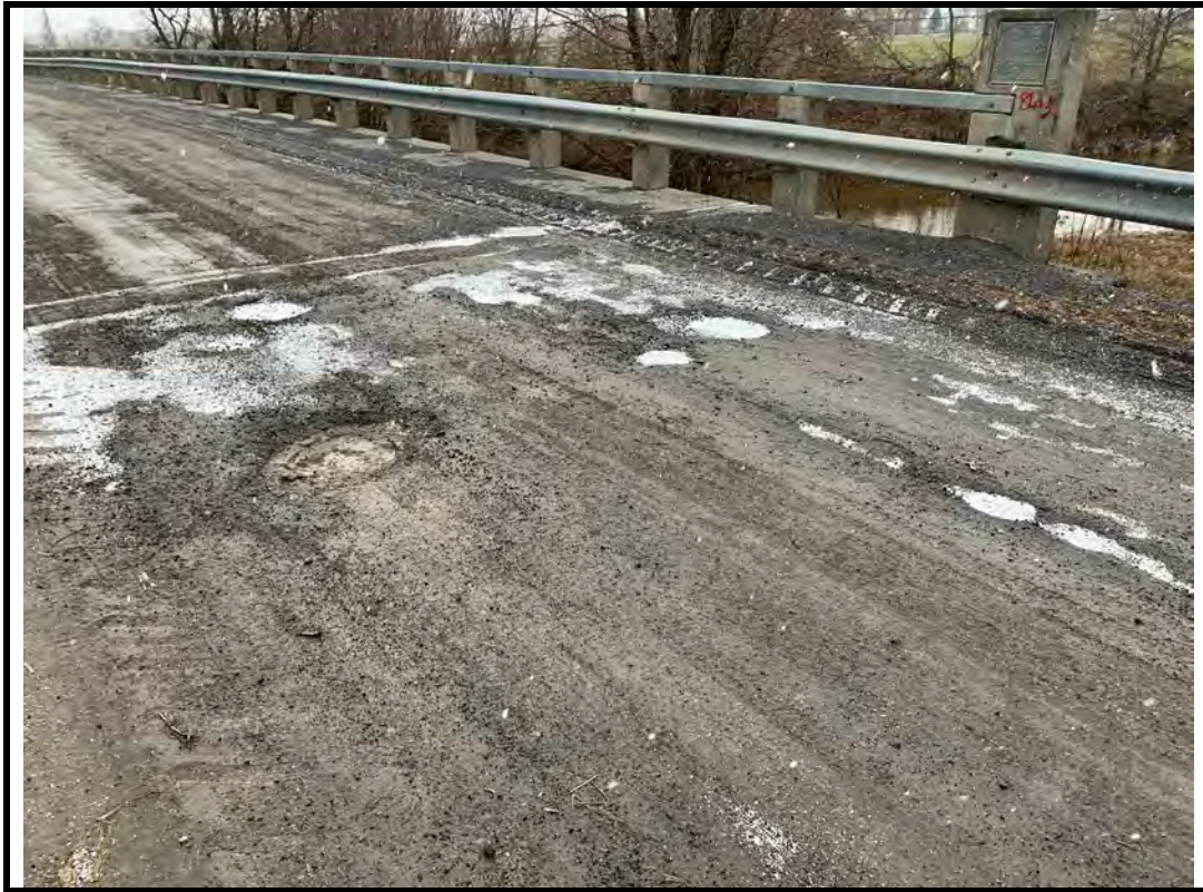
Photo 7 Settlement and large potholes on north wearing surface
