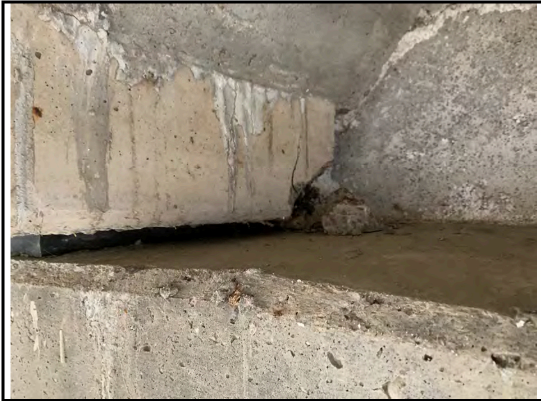
Photo 15 Spall at east end of interior girder
