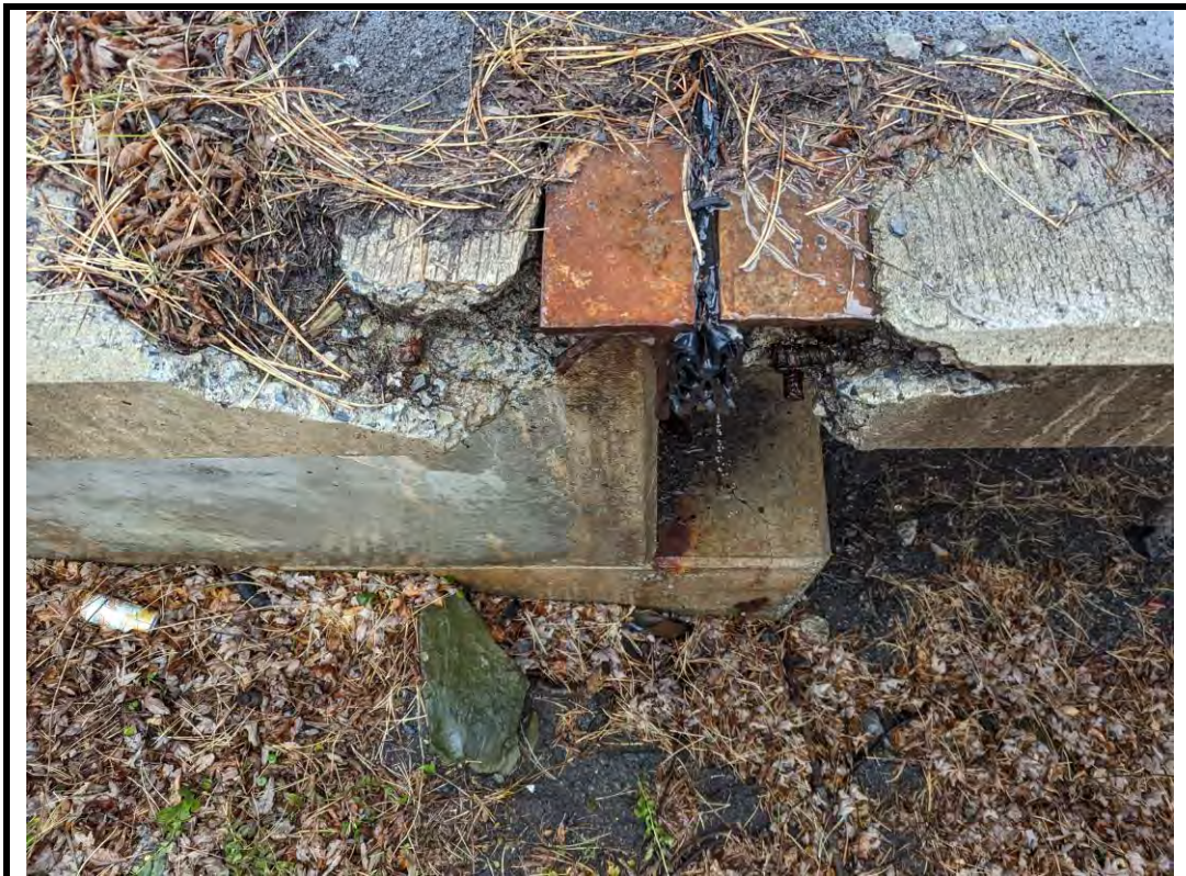
Photo 12 Spalls on deck fascia/soffit at north expansion joint, with squished seal
