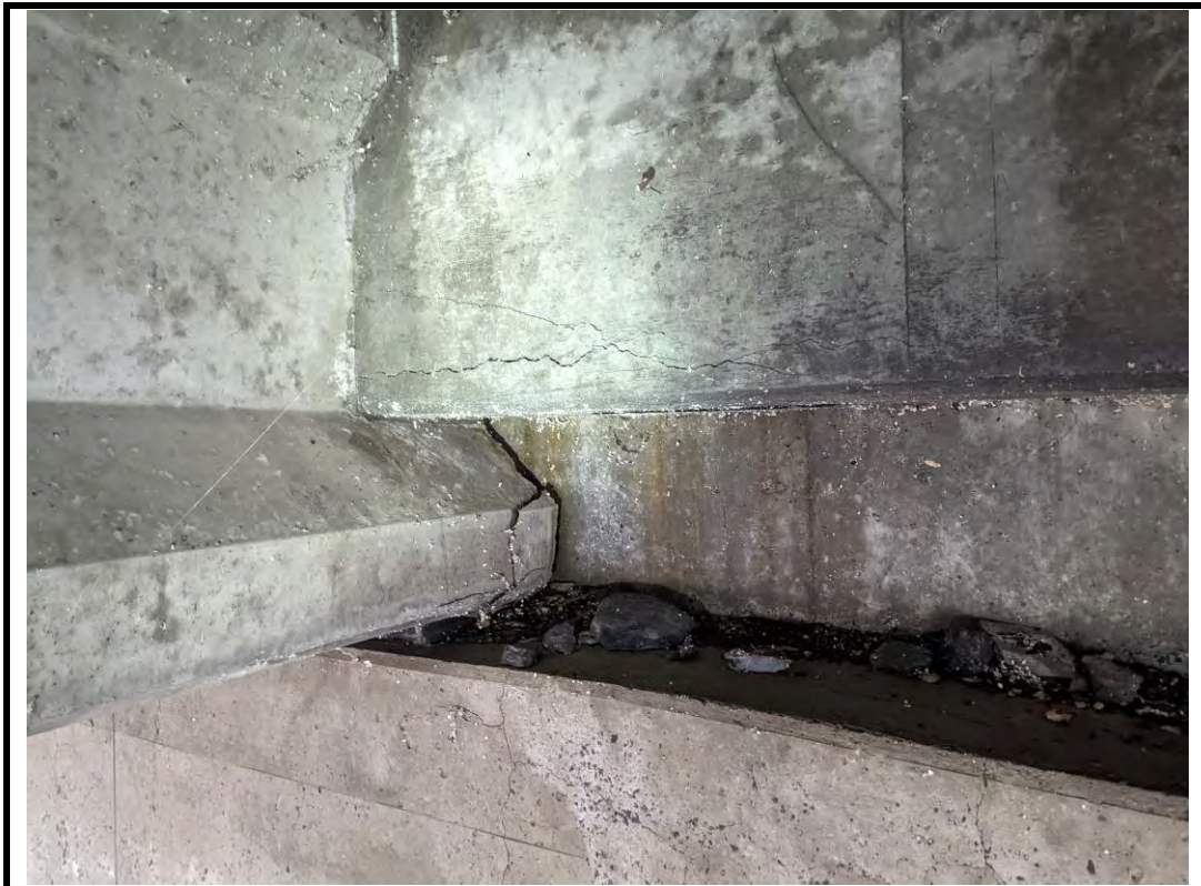
Photo 18 Cracks and delamination in south concrete girders and diaphragms
