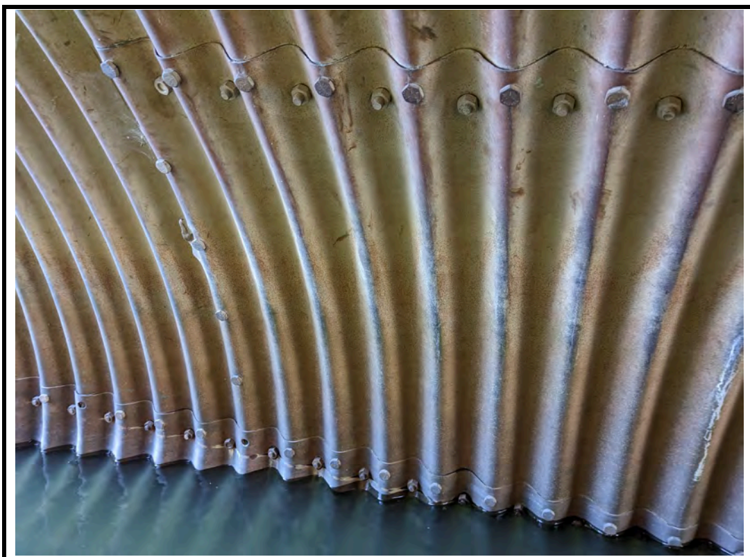
Photo 10 Cracks at bolt line at barrel wall
