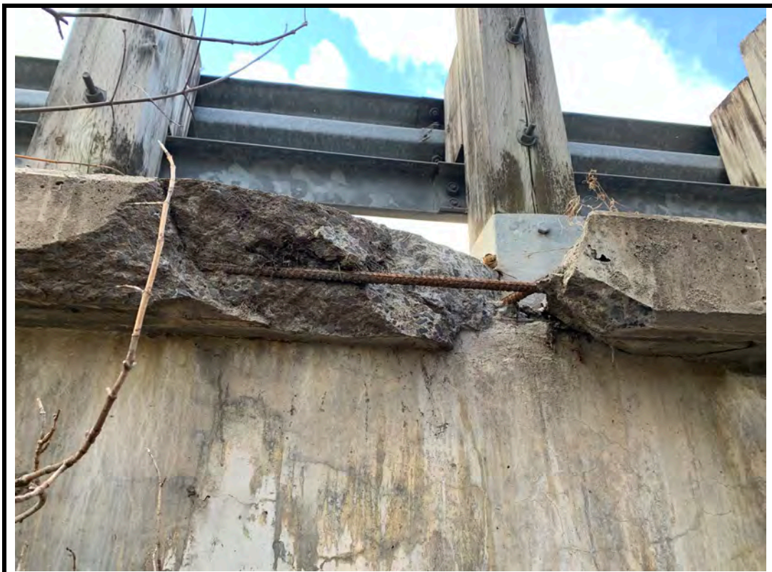
Photo 14 Spall with exposed corroded reinforcement on east fascia
