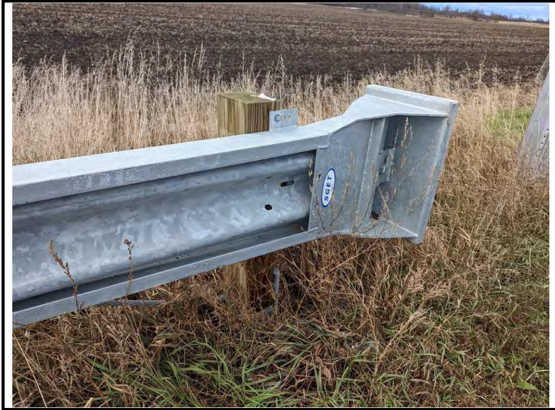
Photo 7 Recently installed guide rail and end-treatments
