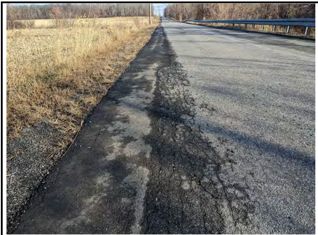
Photo 8 Edge cracking on northwest edge of approach
