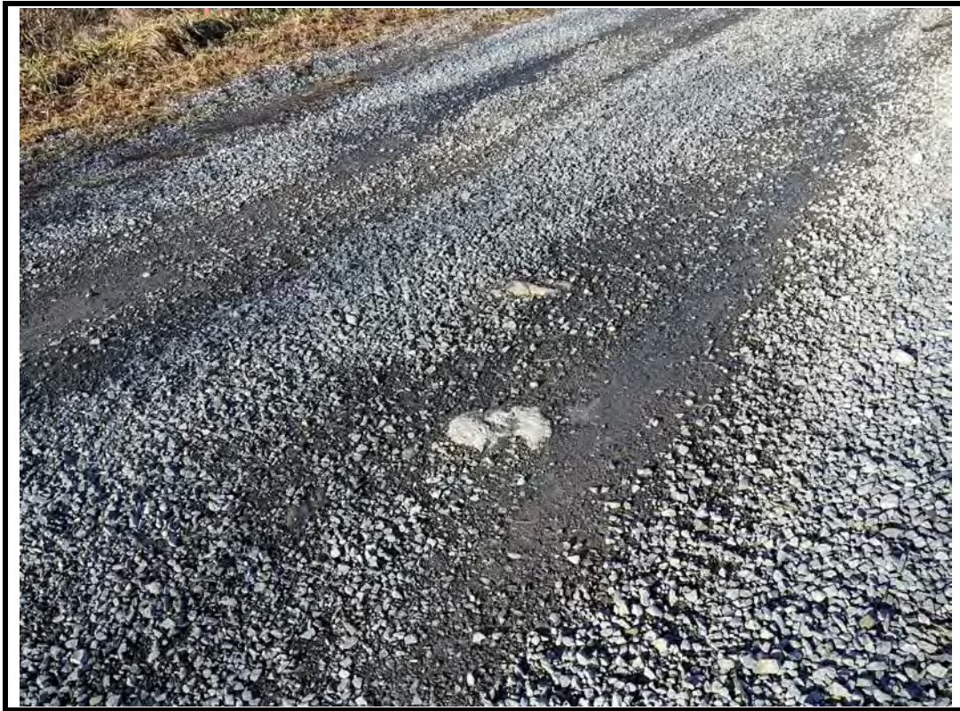
Photo 7 Tire rutting and potholes on south approach wearing surface
