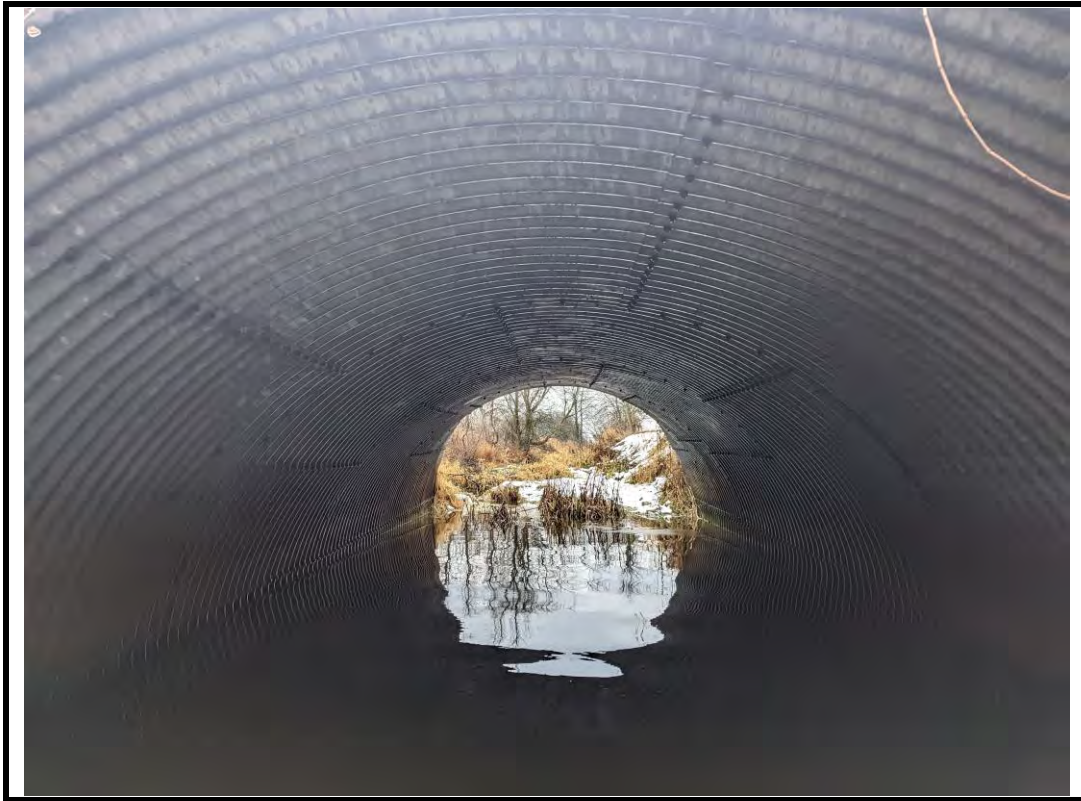
Photo 7 View of culvert sag from the North side
