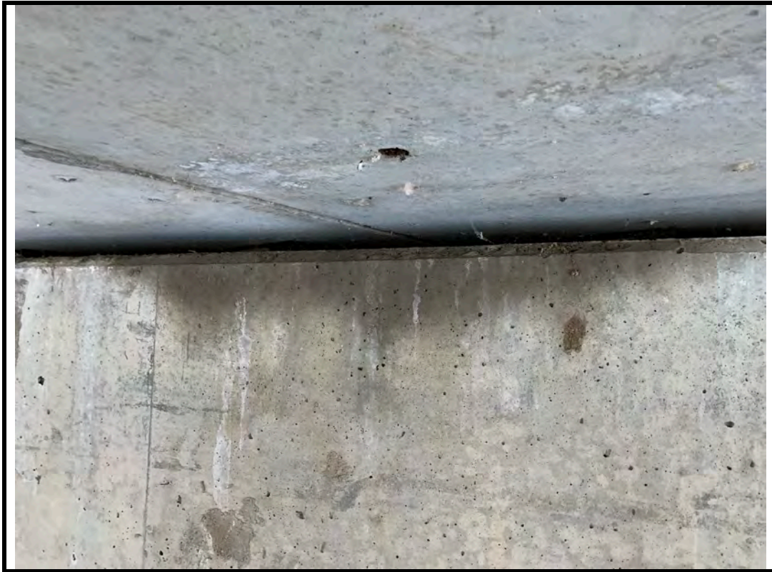
Photo 17 Damp staining and evidence of leakage on south abutment wall
