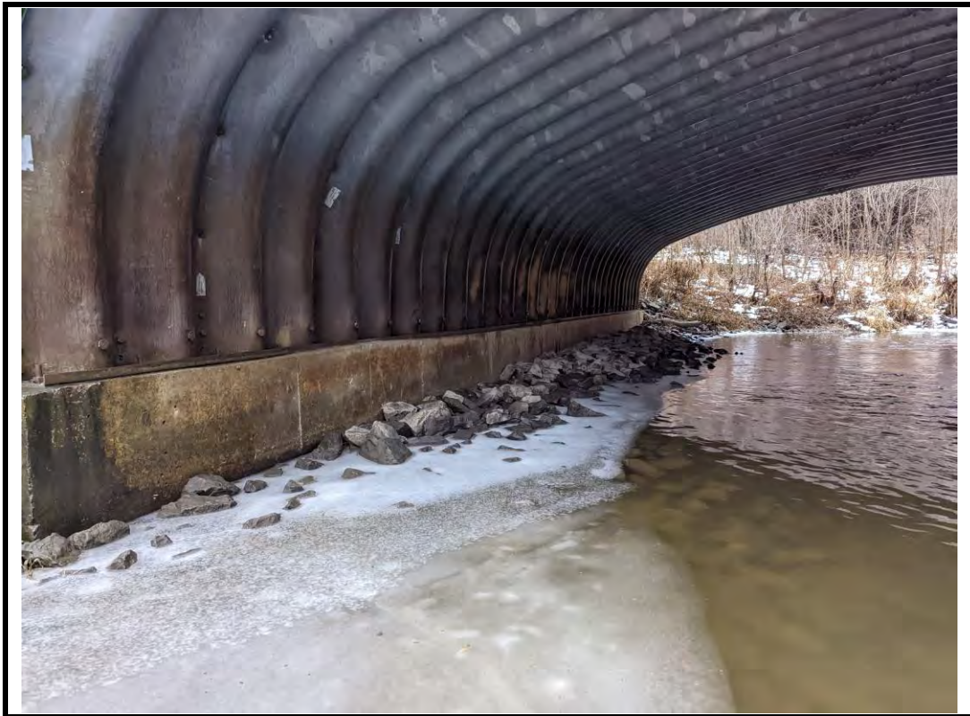
Photo 10 Coating failure within culvert along east strip footing
