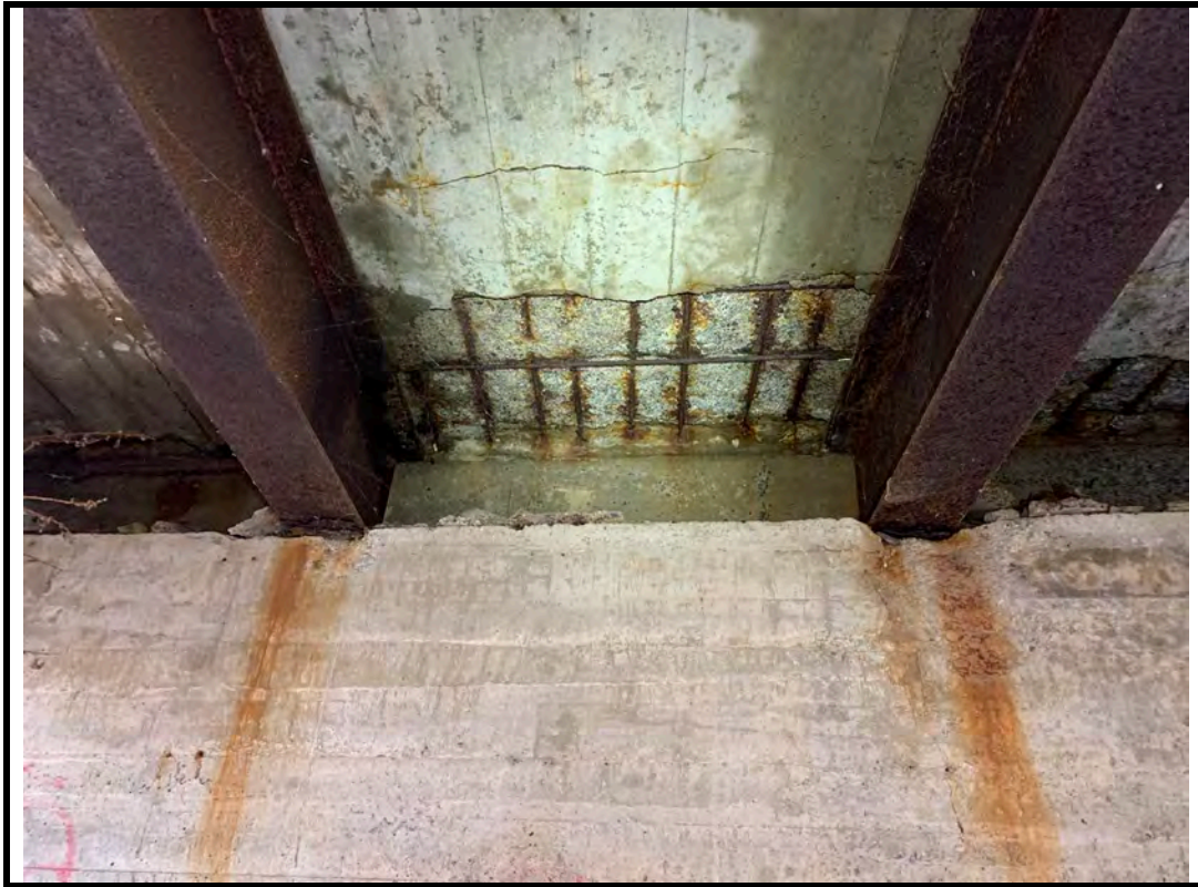
Photo 11 Large spall with ECR at west end of soffit
