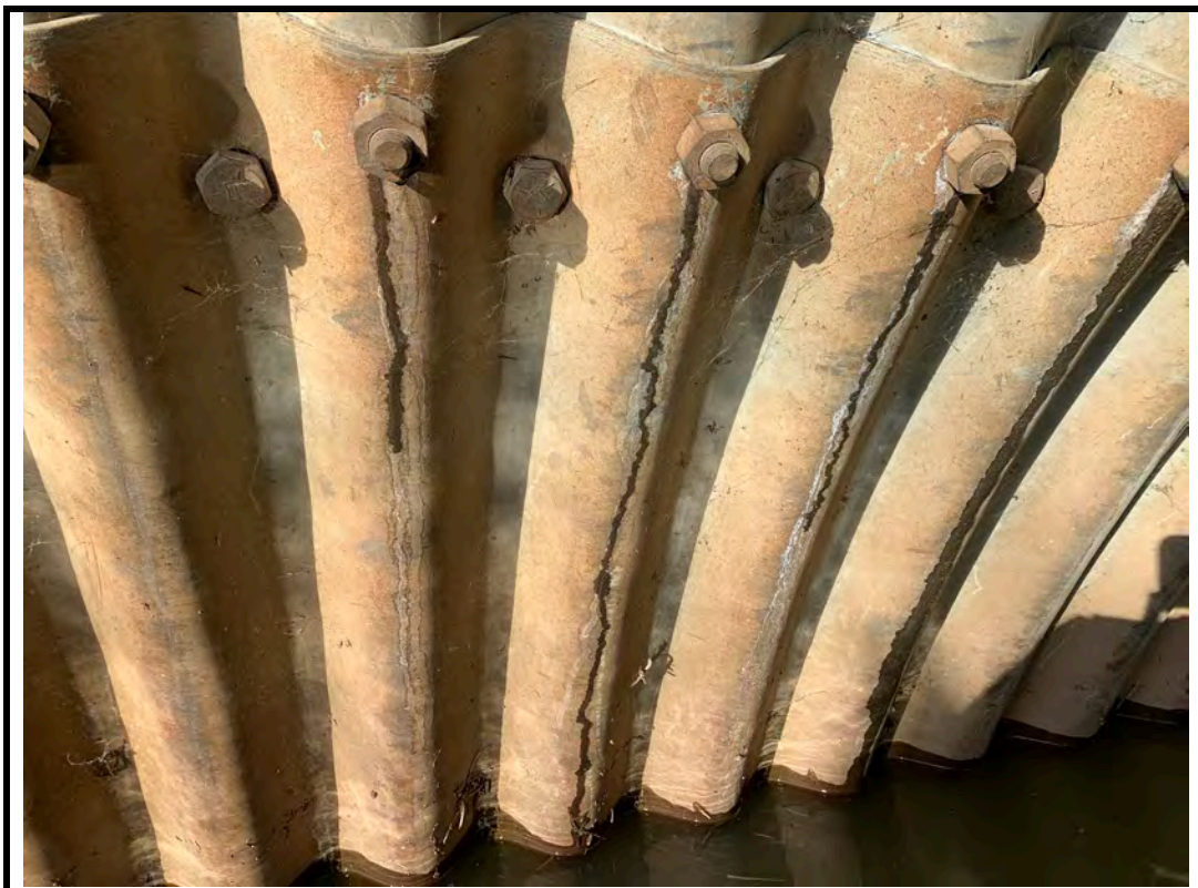
Photo 8 Evidence of leakage from bolt lines at northwest corner of barrel
