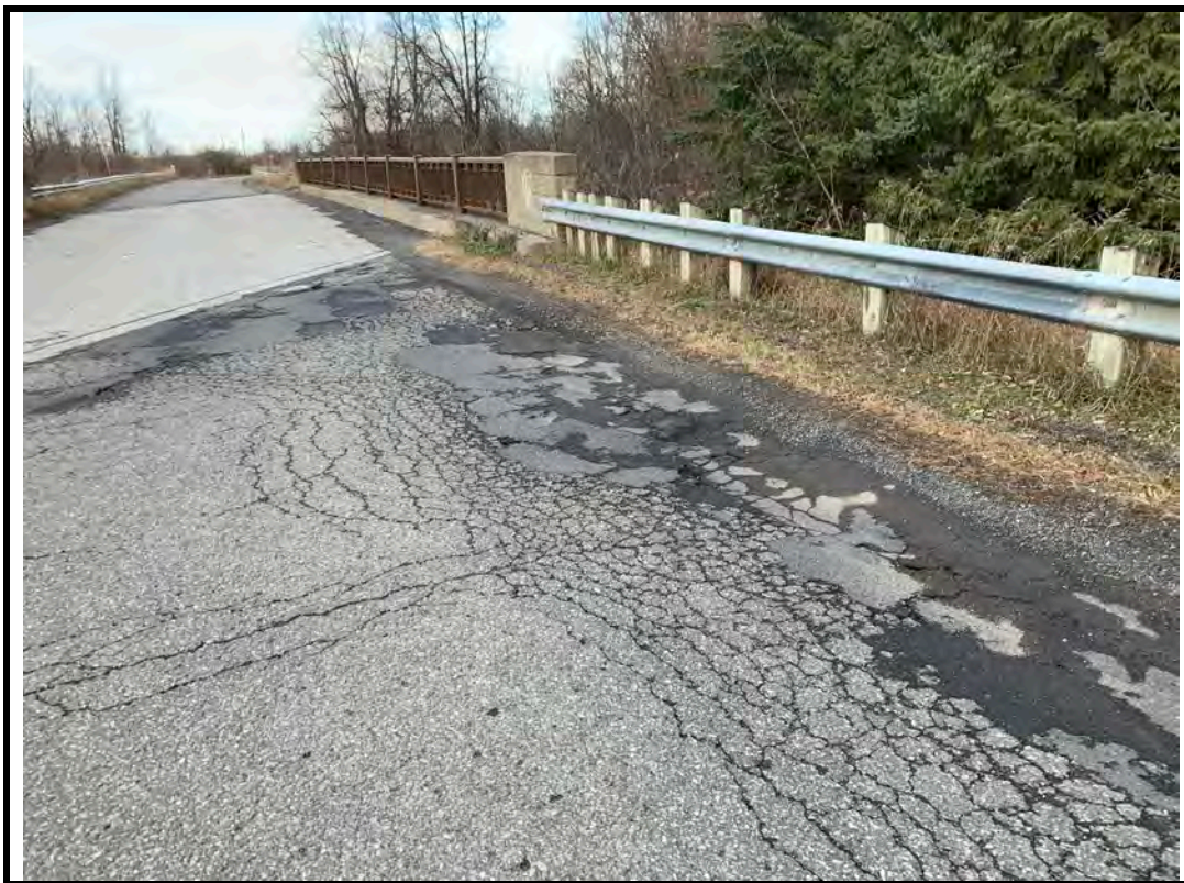
Photo 7 Wide pattern cracks, potholes and asphalt patches on north approach
