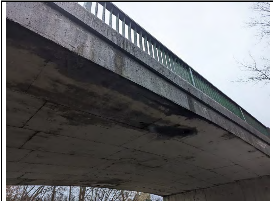
Photo 10 Wet areas around drain downspouts on soffit
