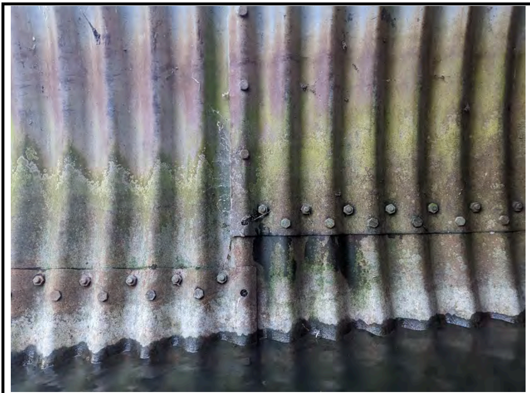
Photo 10 Leaking and missing bolts at plate connections
