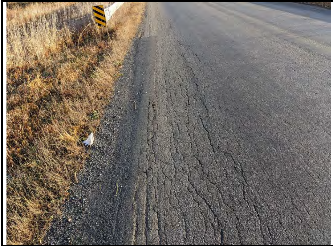
Photo 7 Alligator cracking in west approach wearing surface
