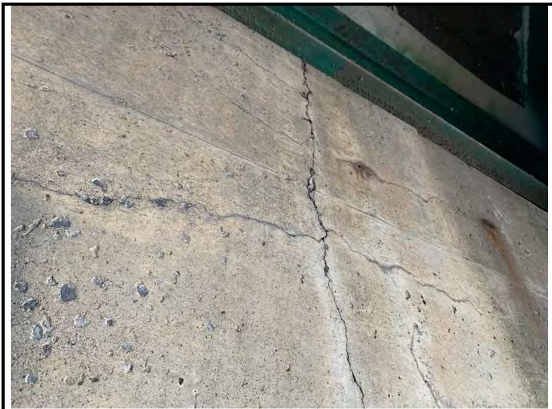
Photo 22 Wide vertical crack on south abutment wall
