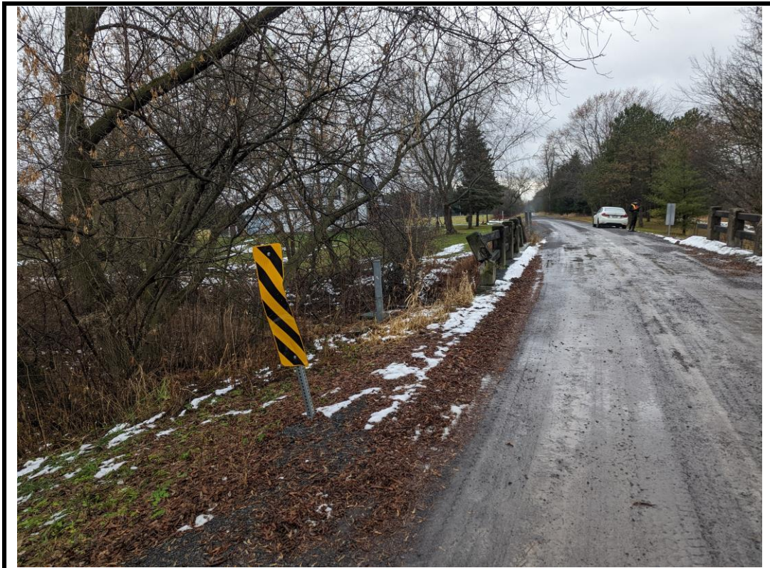
Photo 8 Deformed hazard sign at southeast
