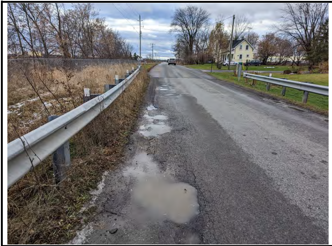
Photo 9 Potholes, ponding, and cracks in asphalt wearing surface
