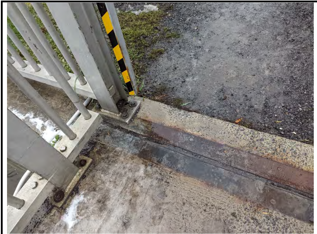
Photo 10 Corrosion and debris at South deck joint (typical)
