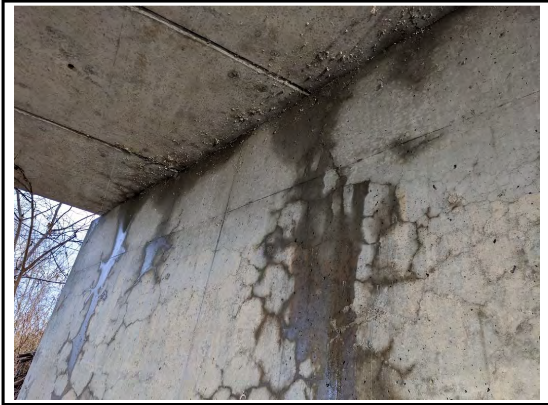
Photo 15 Evidence of joint failure at east abutment wall
