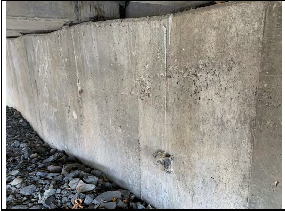
Photo 19 Localized moderate honeycombing on east abutment wall
