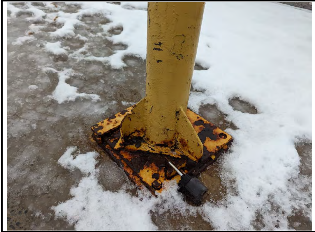
Photo 7 Corrosion and missing bolts at south bollard base (typical)
