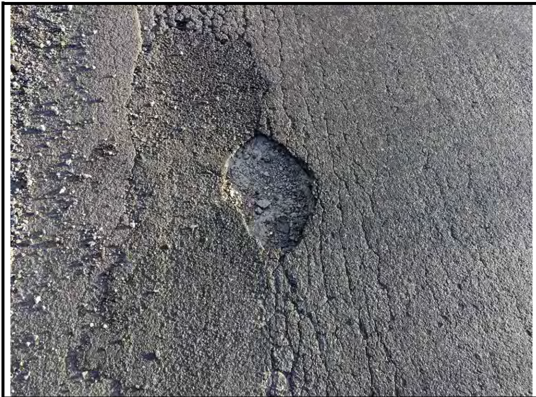
Photo 8 Pothole in west approach
