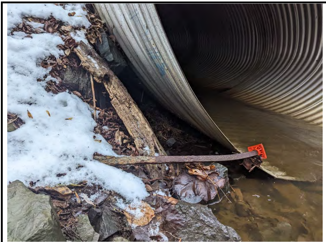
Photo 8 Typical scour / undermining of culvert (North inlet shown)
