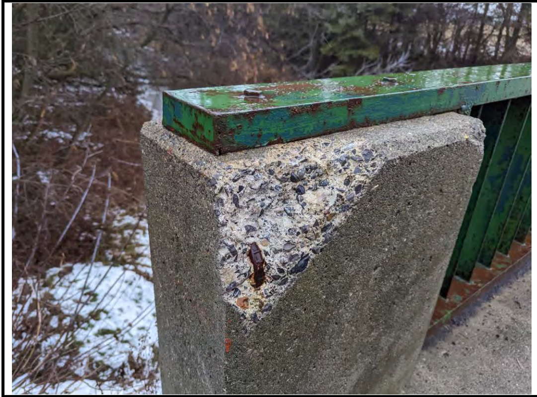
Photo 7 Spall at Northwest barrier end wall with ECR
