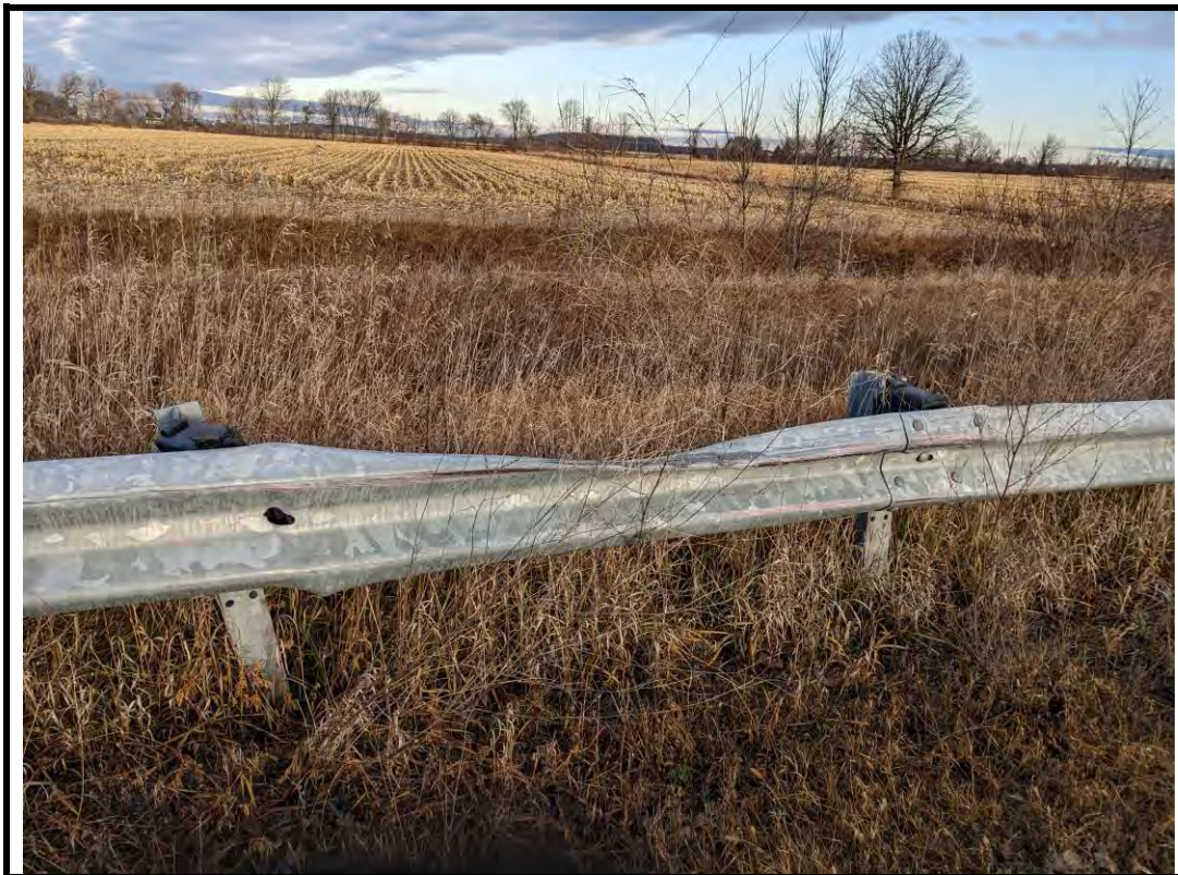
Photo 10 Impact damage at northeast approach barrier
