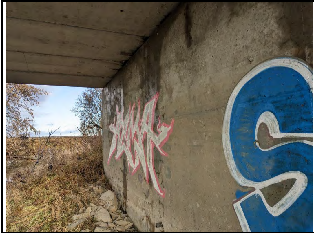
Photo 15 Evidence of leaking and joint failure at east abutment wall
