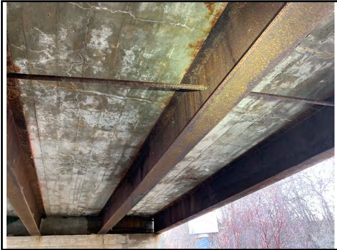
Photo 15 Corrosion on steel tie diaphragm
