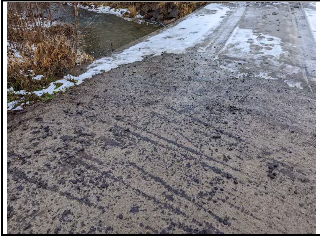
Photo 13 Scaling along top of exposed concrete deck
