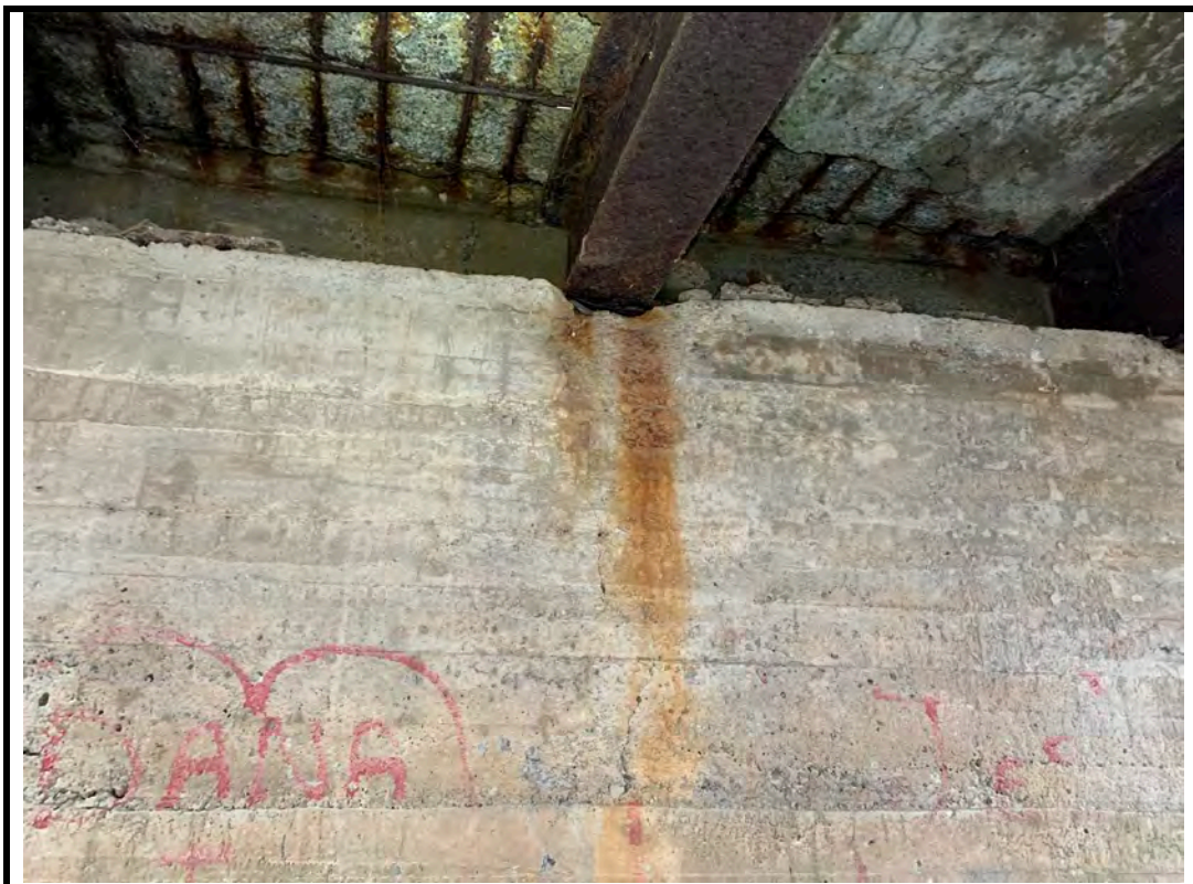
Photo 16 Spall and wide vertical crack below girder on west abutment wall
