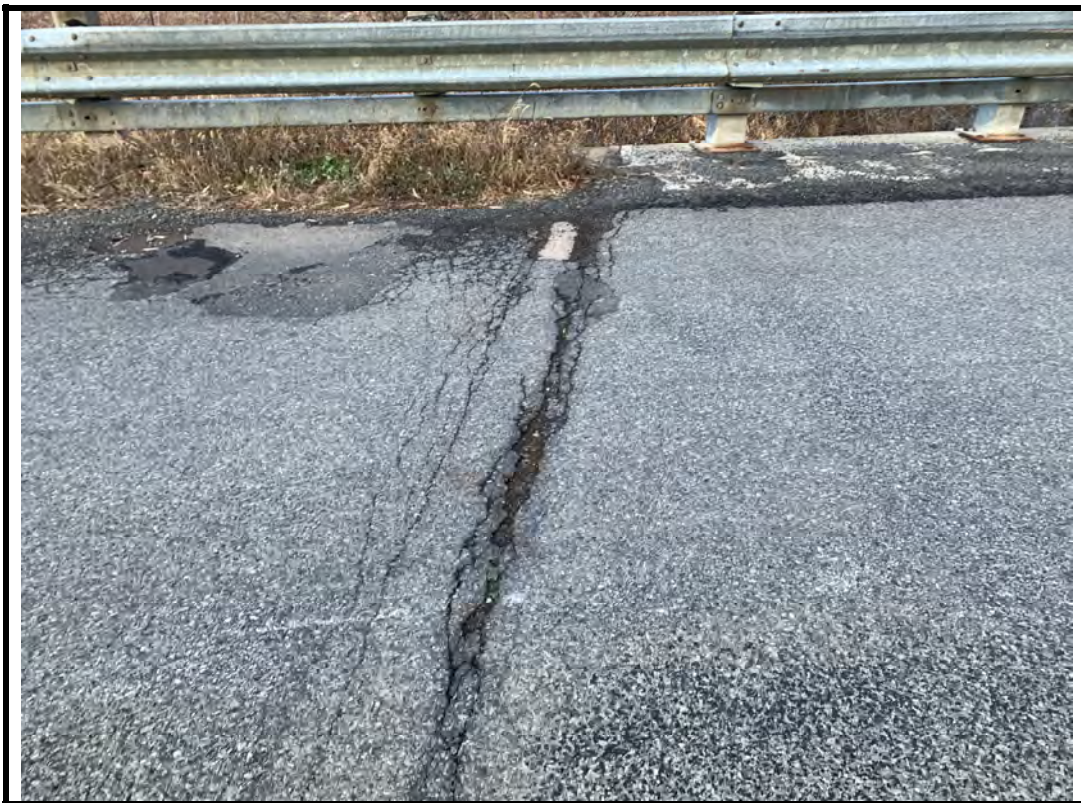
Photo 12 Wide crack and small potholes at west end of deck, at joint location
