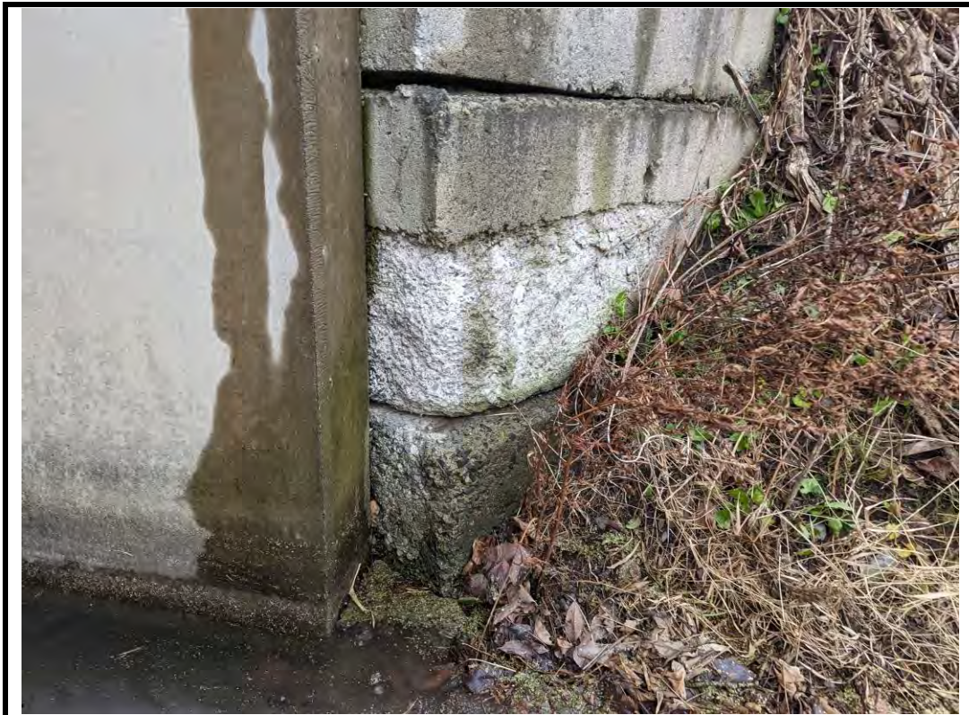
Photo 10 Scaling/disintegration on northeast retaining wall
