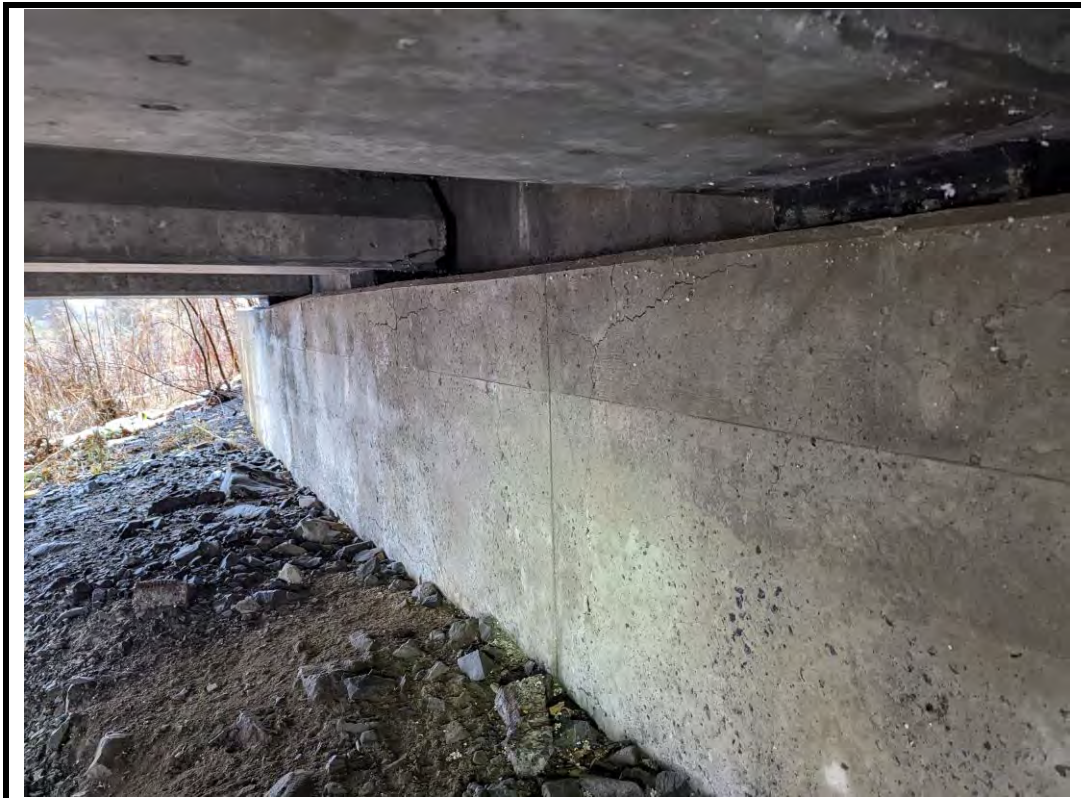
Photo 22 Cracks on South abutment wall.
