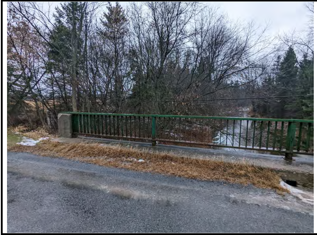
Photo 9 Vegetation along north edge of asphalt over deck (typical)
