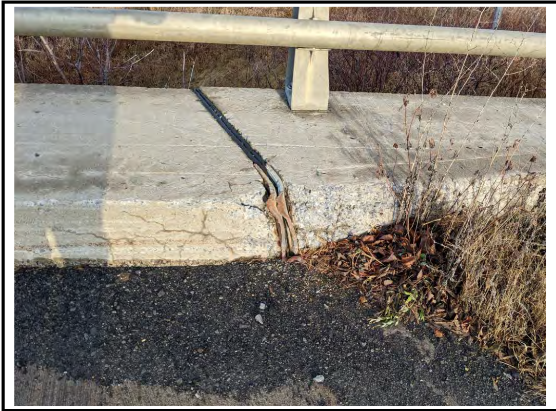
Photo 17 Scaling on curb and damage at northeast joint
