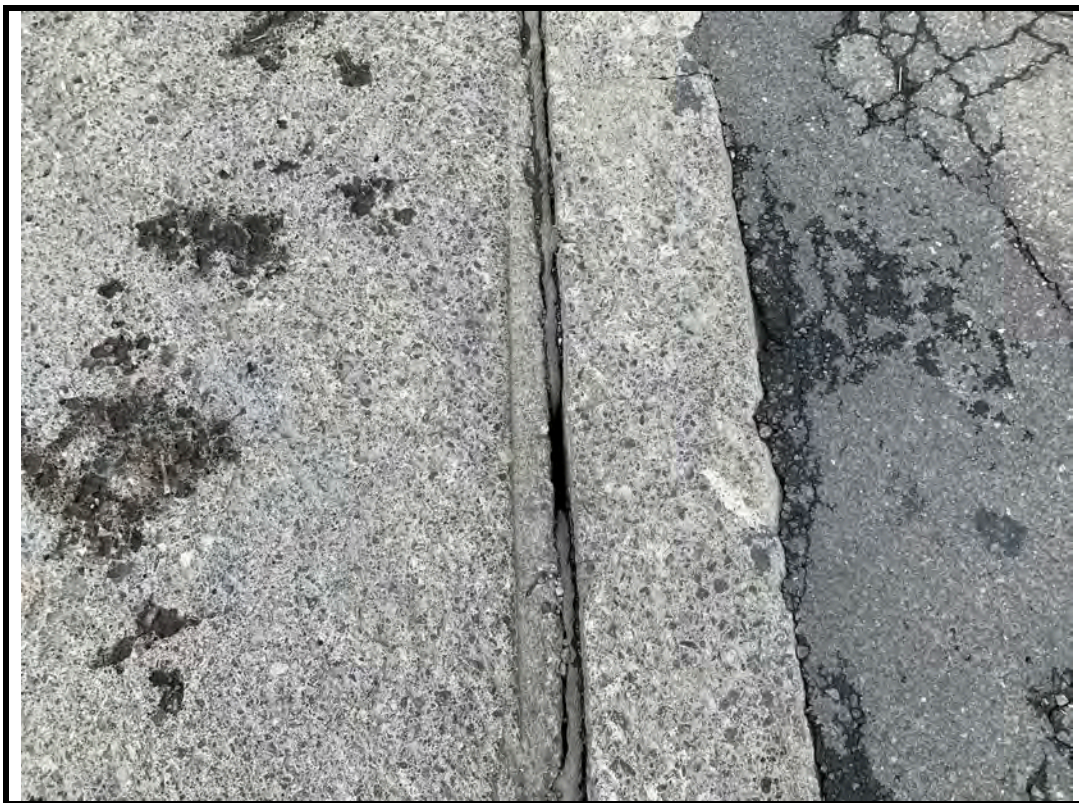
Photo 9 Missing portion of seal on north expansion joint
