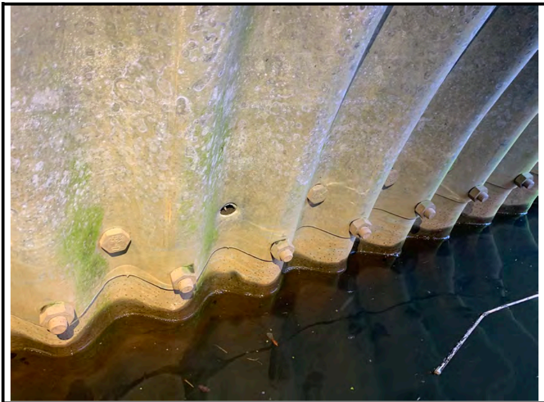
Photo 10 Missing bolt at west end of barrel
