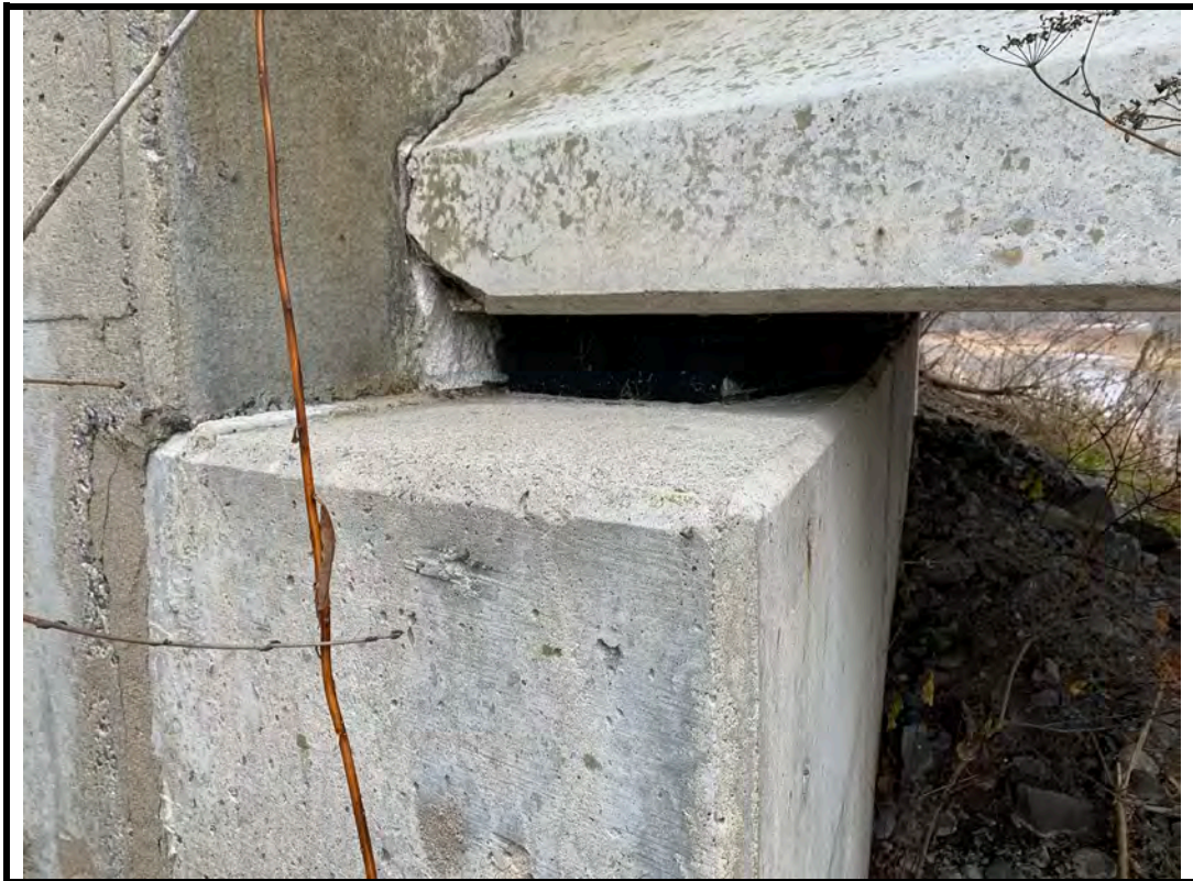
Photo 14 Small spall at west end of south girder
