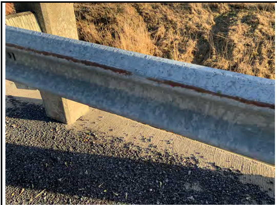
Photo 10 Collision damage on southwest corner of deck barrier
