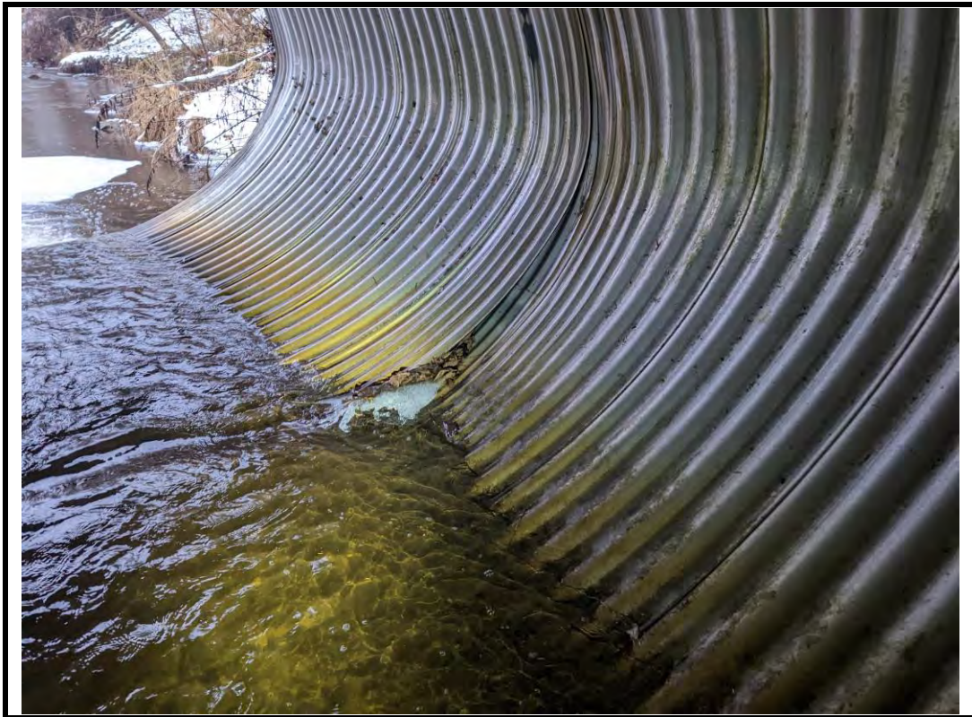
Photo 10 Separation of south barrel segment causing scour/piping
