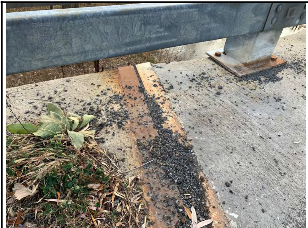
Photo 10 Light corrosion noted on visible portions of expansion joint
