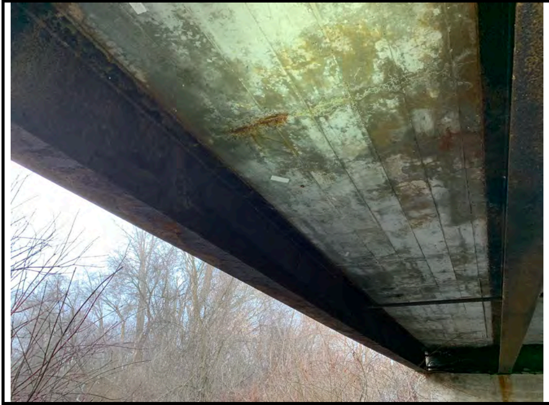
Photo 13 Rust stains efflorescence on interior soffit
