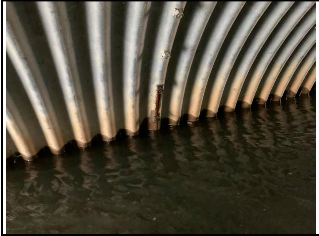
Photo 9 Evidence of leakage at east end of barrel
