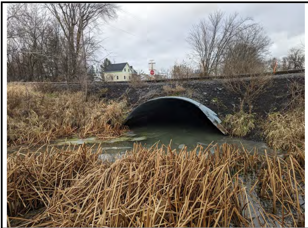
Photo 10 Deformation at inlet on the southwest corner of structure
