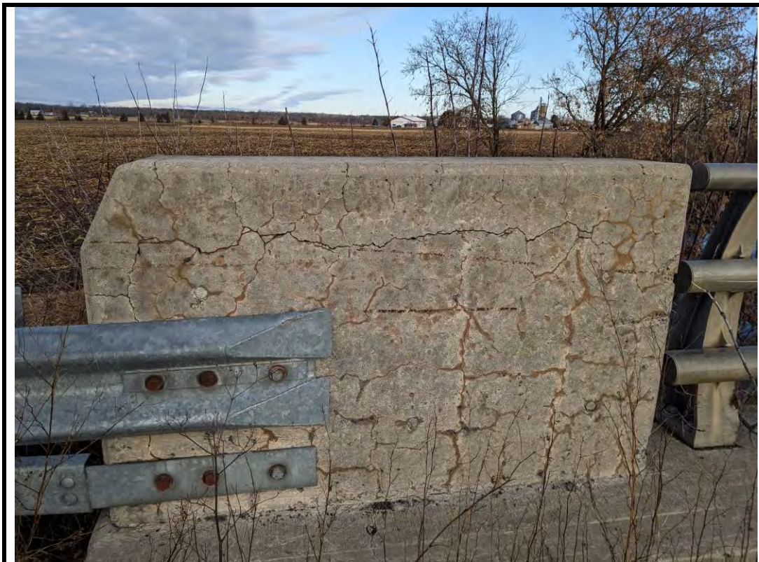
Photo 10 Wide AAR cracking at northwest barrier end wall
