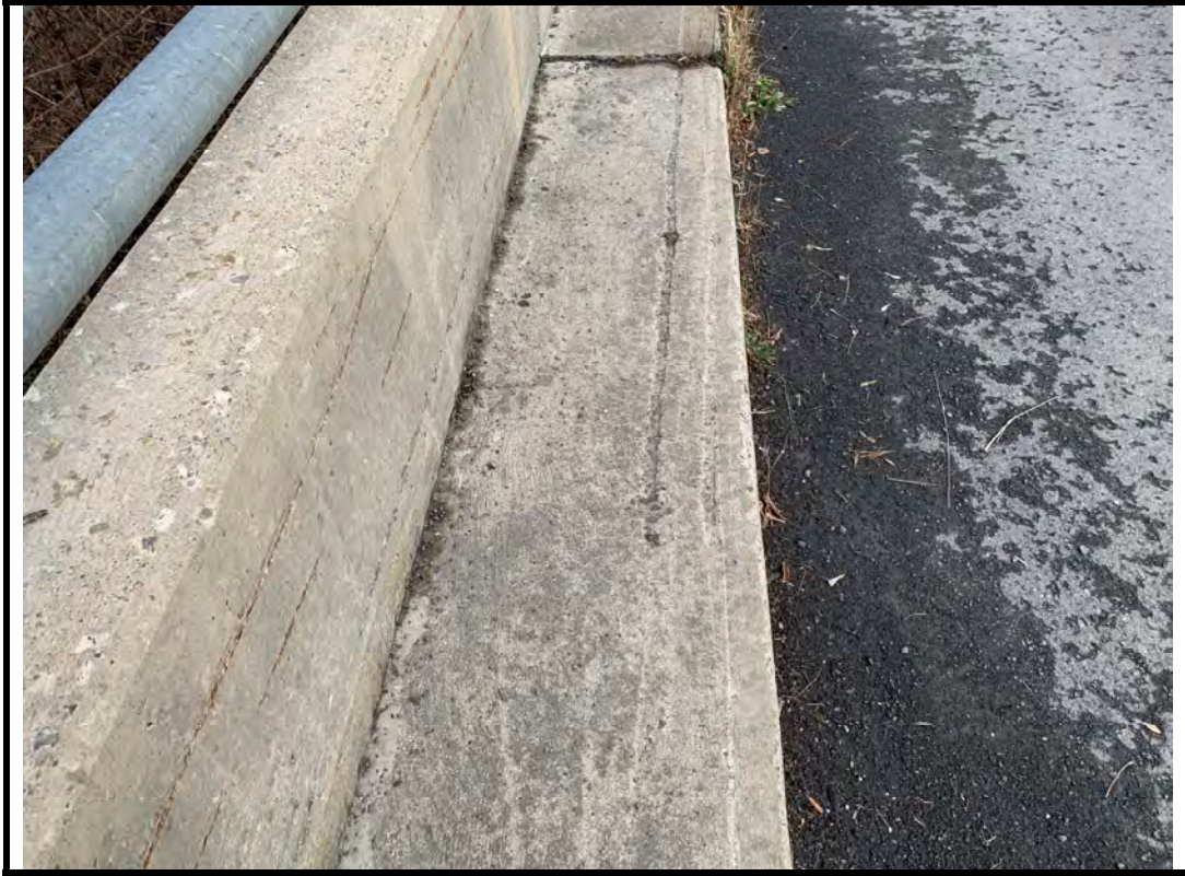
Photo 9 Abrasions on south curb
