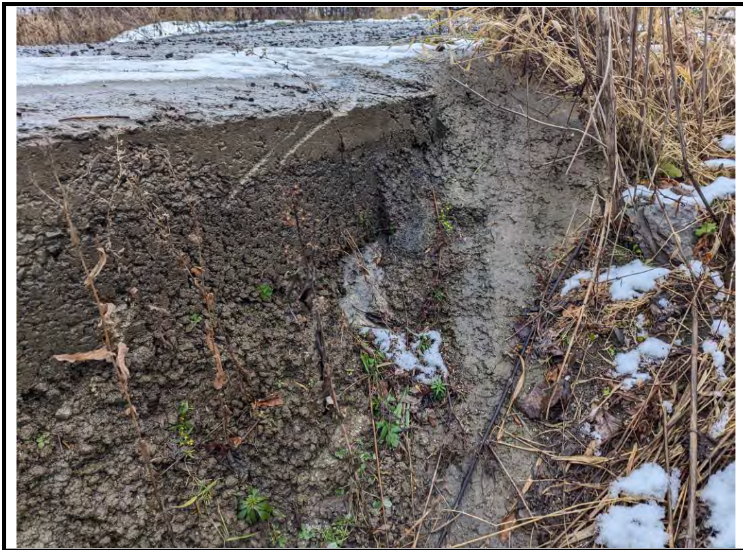
Photo 12 Severe scaling of concrete wingwalls and slab (typical)
