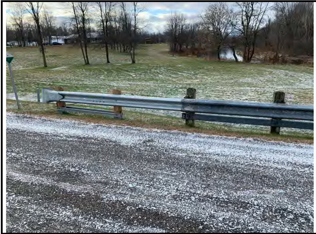
Photo 7 New end treatment at southeast corner
