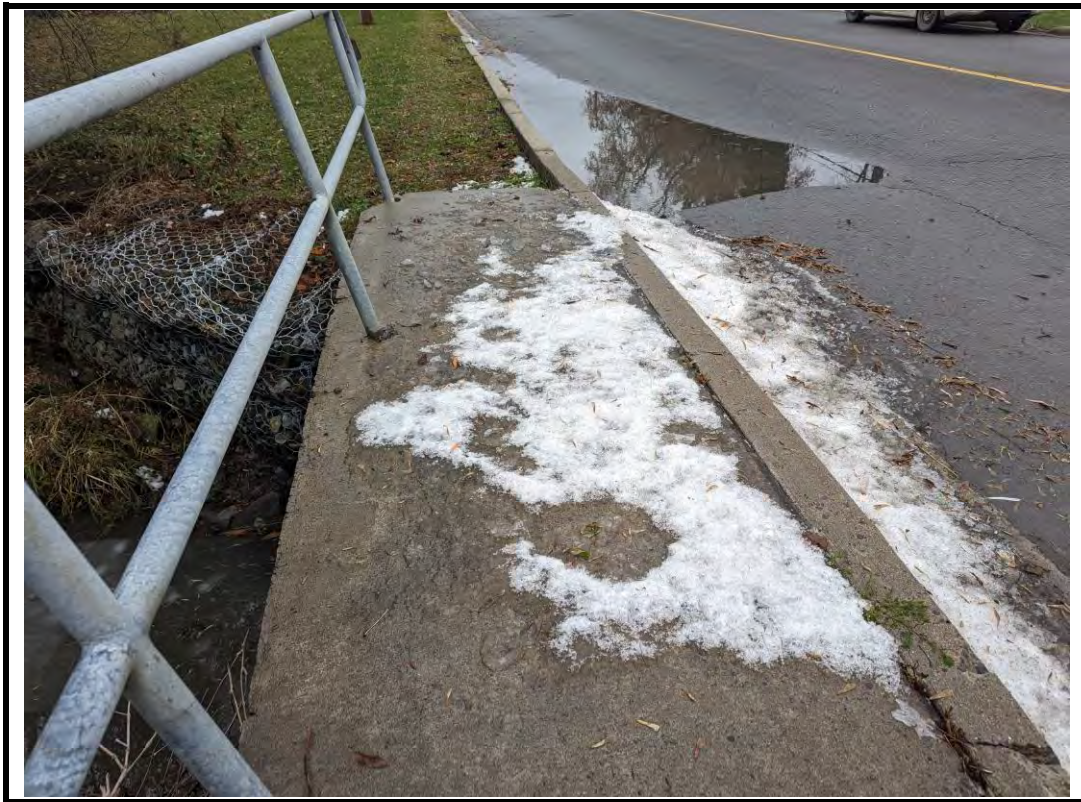
Photo 7 North barrier railing leaning outwards
