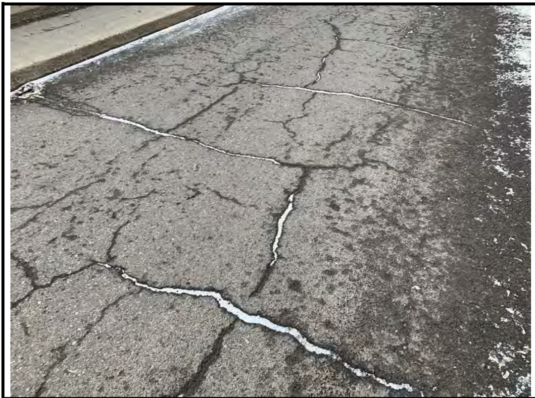
Photo 12 Wide longitudinal and transverse cracks on deck wearing surface
