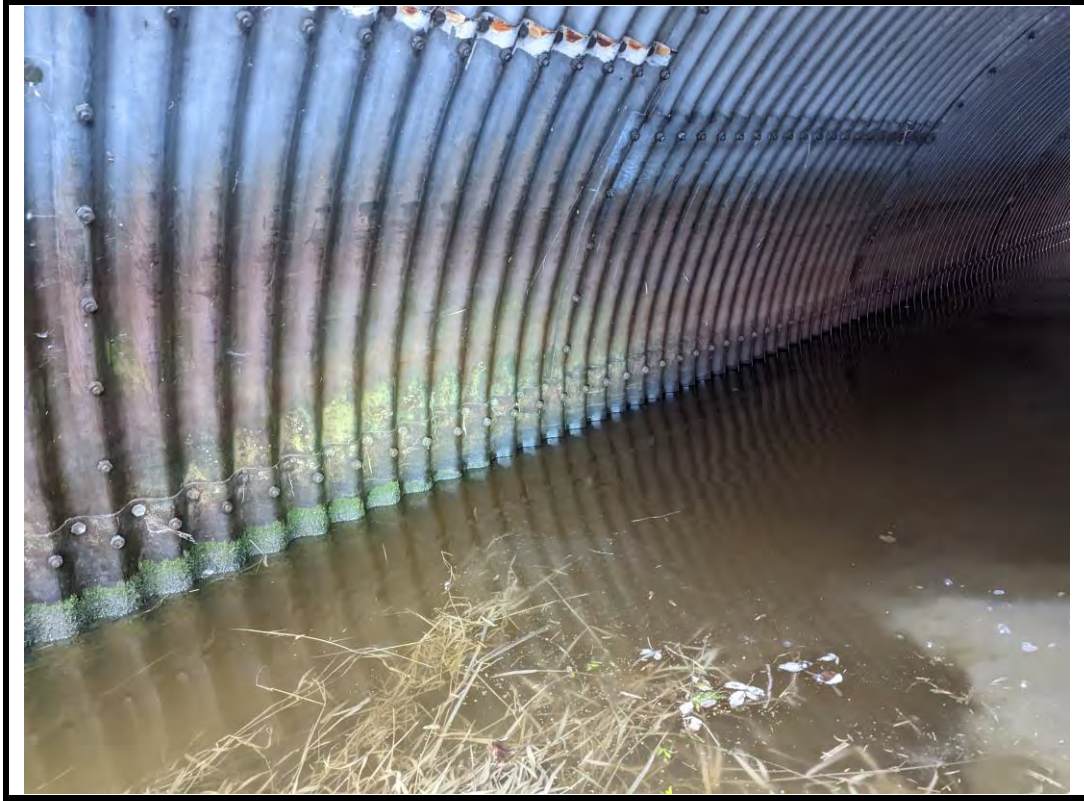
Photo 9 Corrosion and coating loss (typ.)
