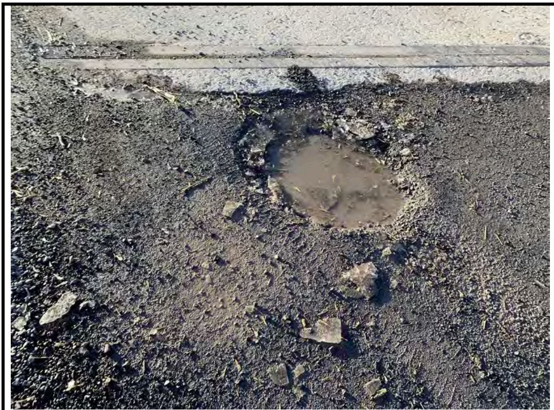
Photo 8 Large potholes and settlement noted on east approach
