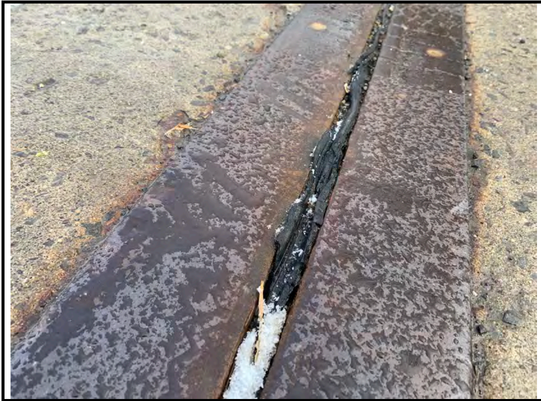
Photo 9 Damage on south joint seal
