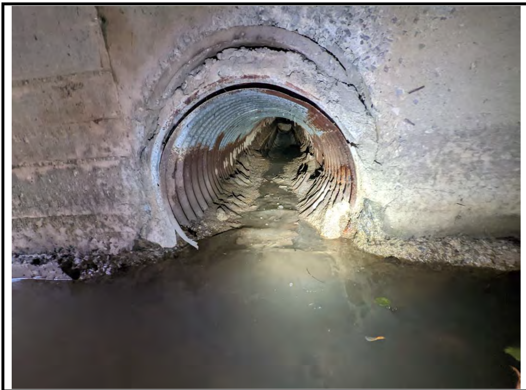
Photo 16 CSP culvert in West culvert side wall
