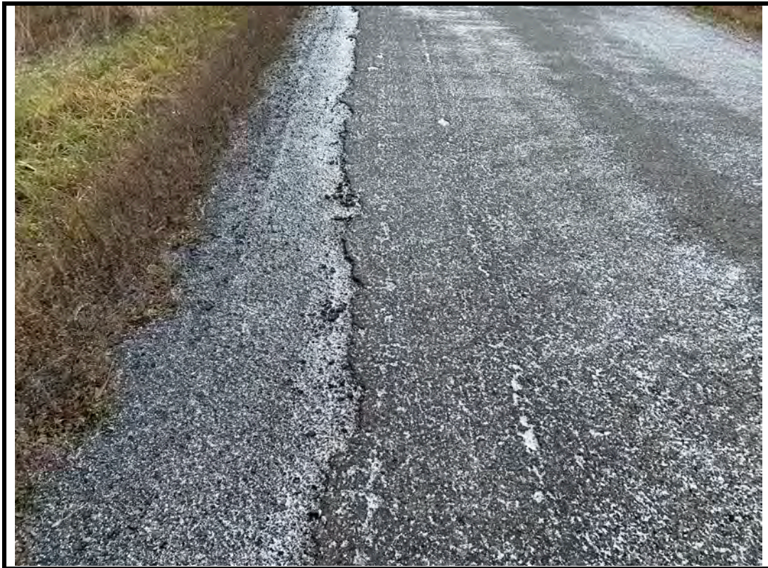
Photo 7 Section loss at east edge of north wearing surface
