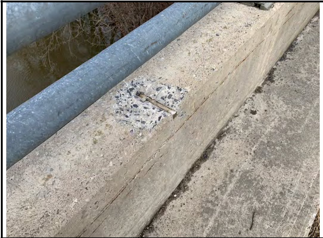
Photo 10 Spall on south barrier wall
