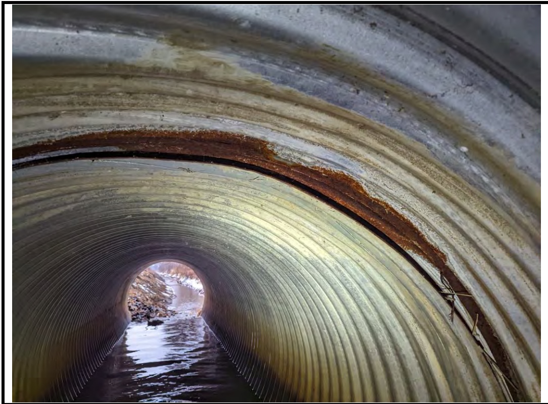
Photo 10 Misalignment of joint in east barrel and localized corrosion
