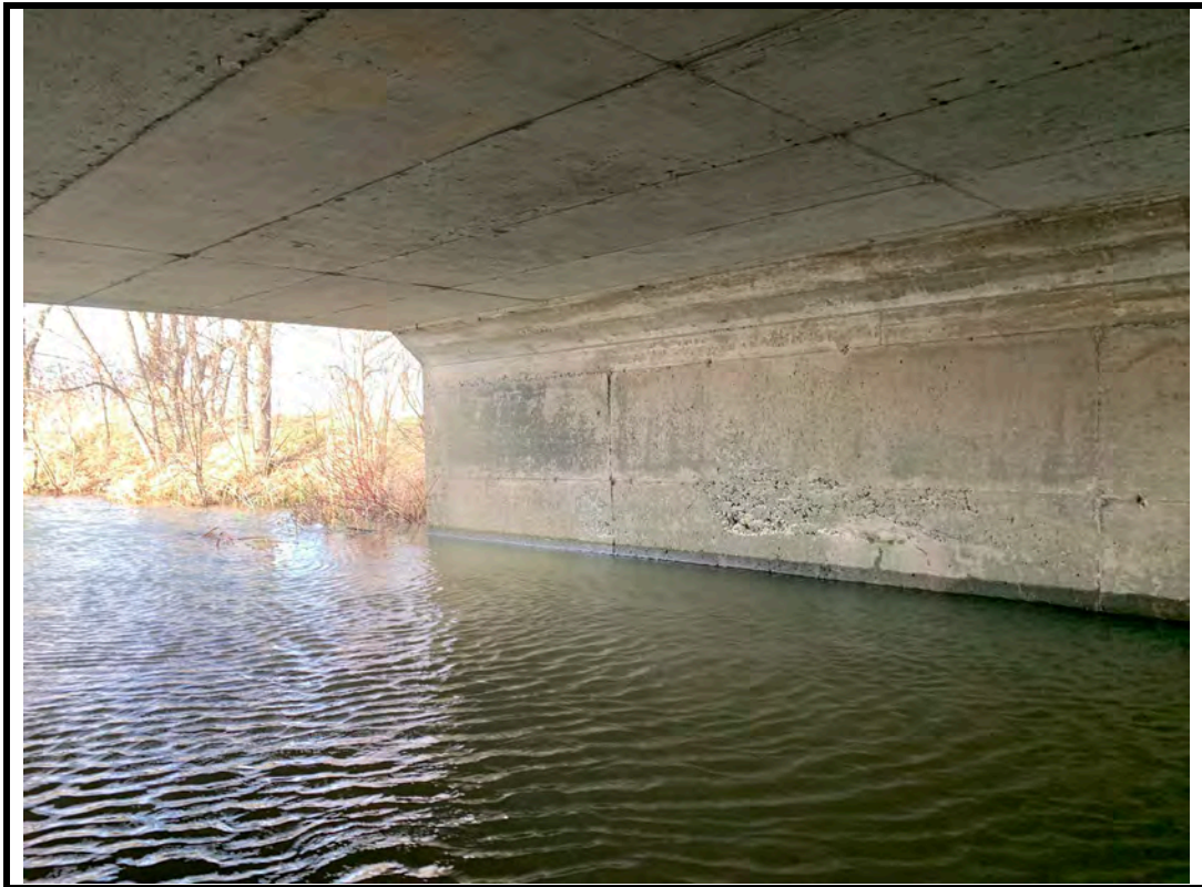
Photo 8 Honeycombing on east wall
