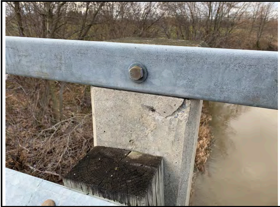
Photo 11 Small spall on concrete barrier post
