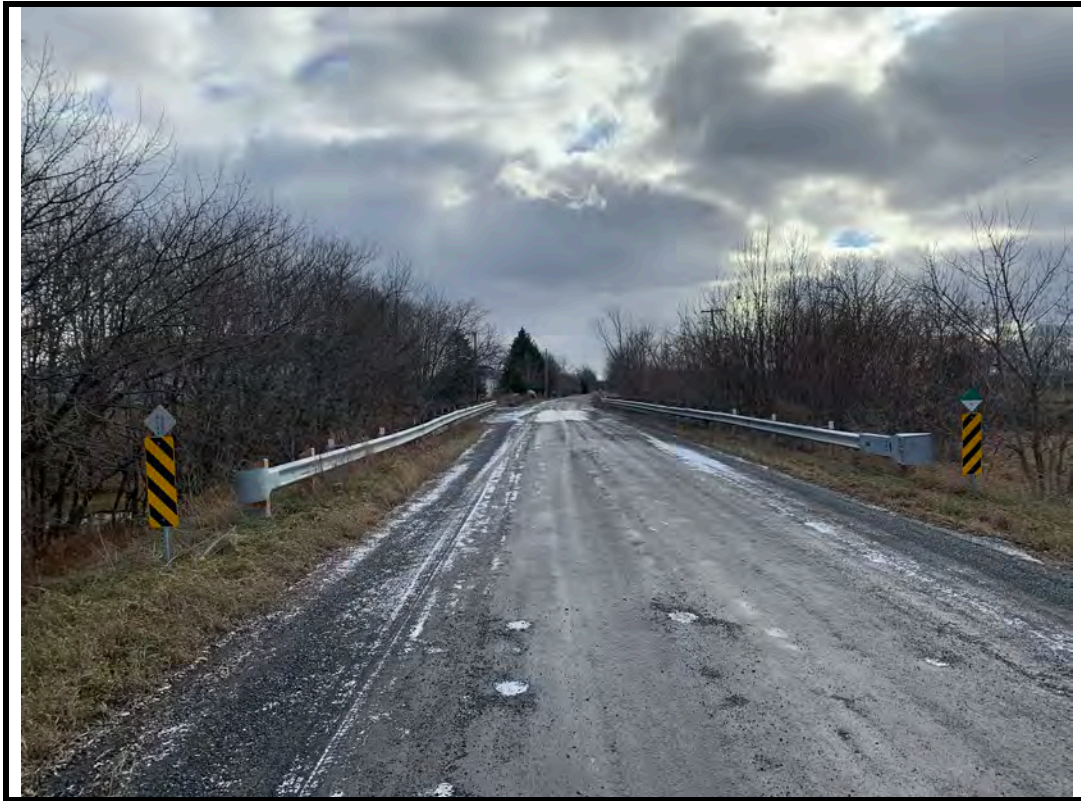
Photo 7 New end treatments installed on north approach
