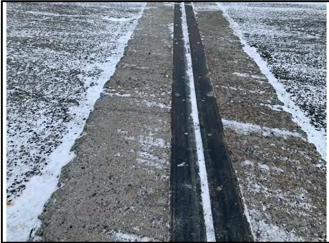
Photo 9 Abrasions on east joint armouring and scaling on concrete end dams
