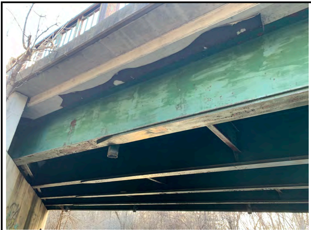
Photo 16 Light corrosion and coating failure on east exterior girder
