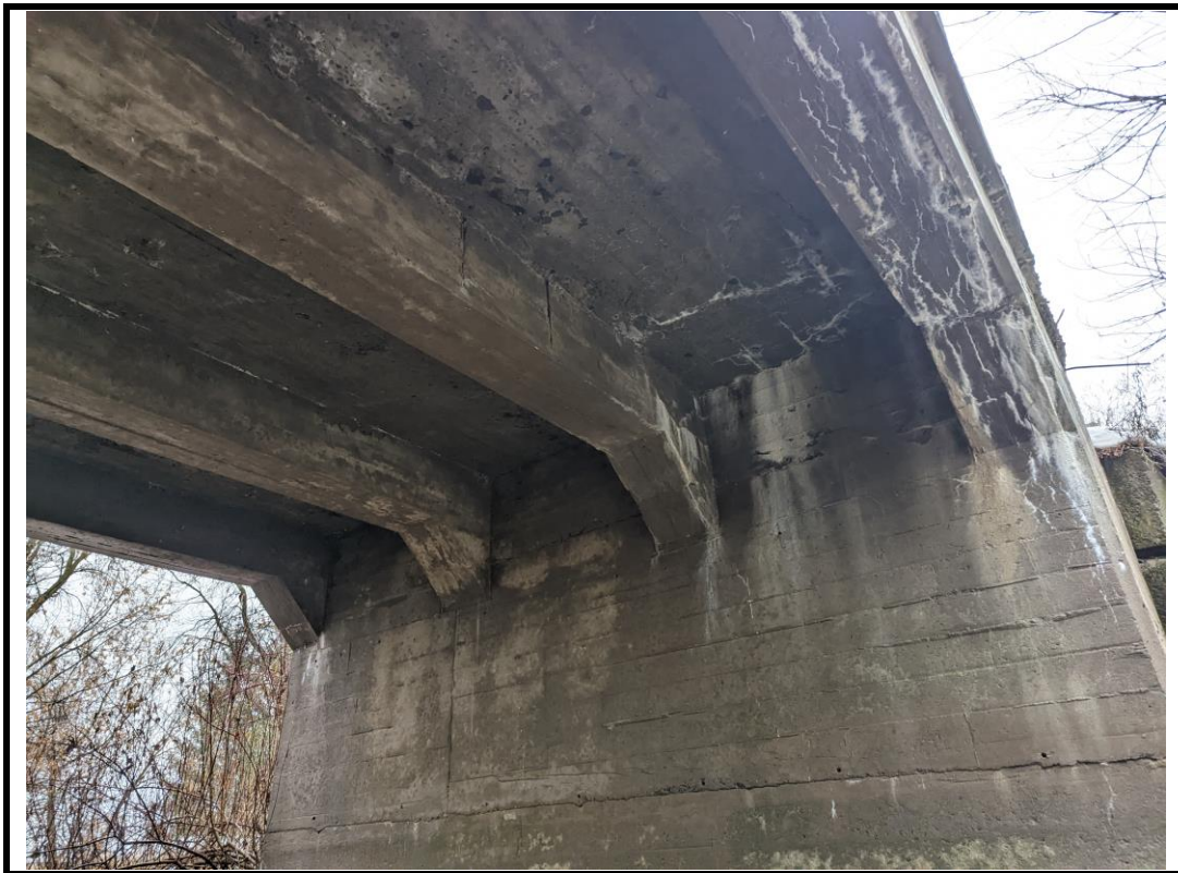
Photo 12 Efflorescence, damp stains, CR, cracks, and scaling on girders and abutment
