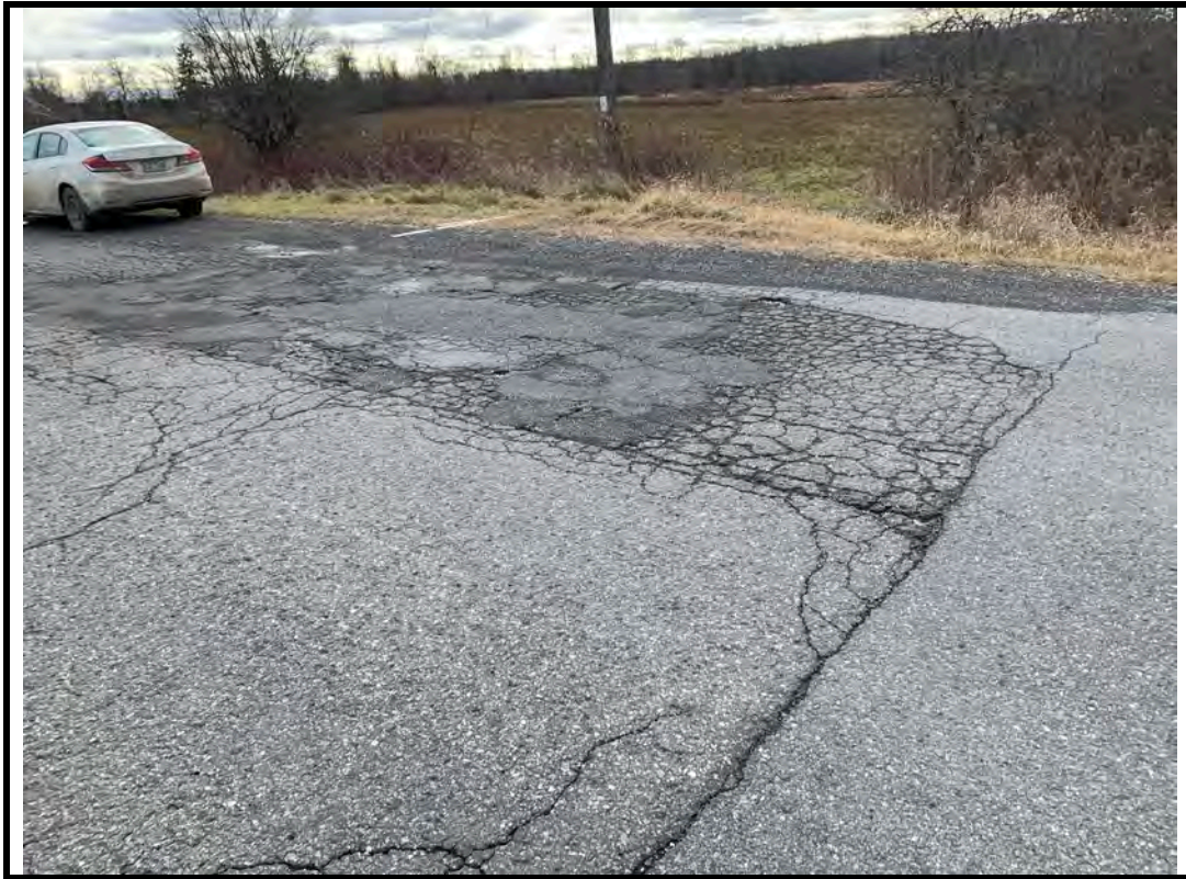
Photo 7 Wide pattern cracks, asphalt patches and potholes on south wearing surface
