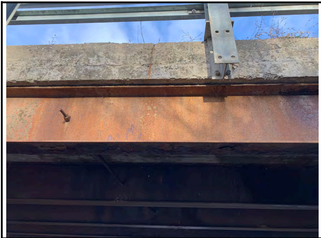
Photo 12 Moderate scaling on south exterior soffit
