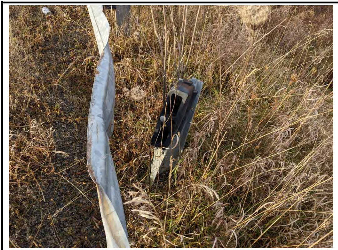
Photo 12 Disconnected and damaged barrier post
