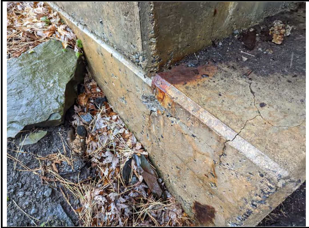
Photo 21 Crack and Spall at northwest wingwall
