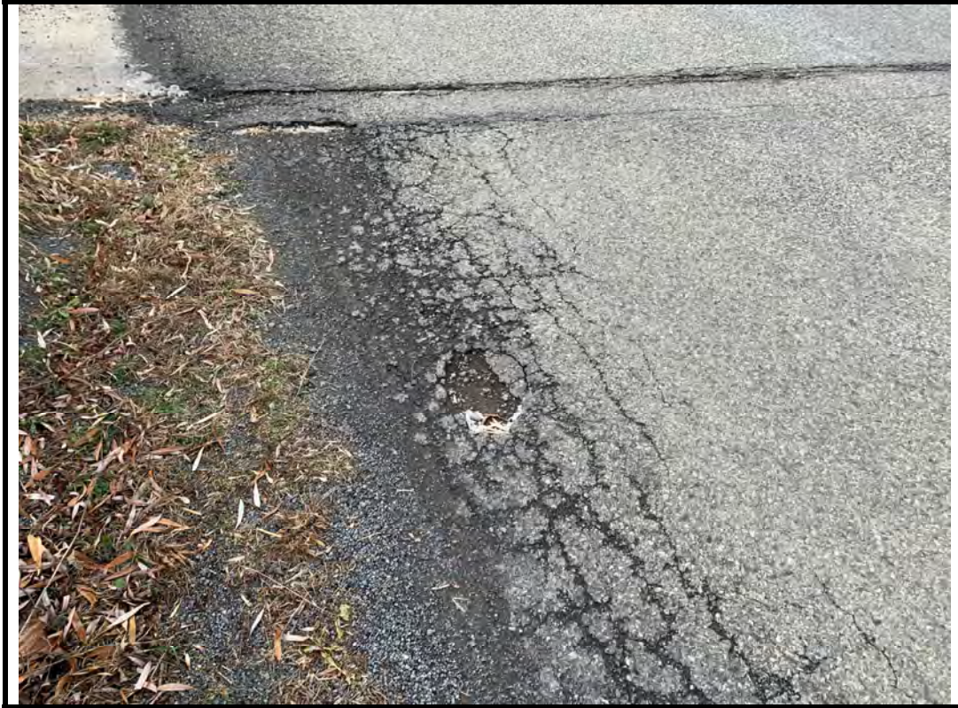
Photo 9 Small potholes at south edge of east approach wearing surface
