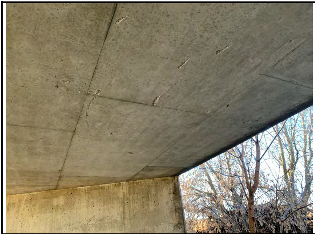
Photo 12 Localized spalls on interior soffit
