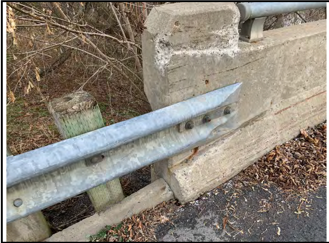
Photo 7 Light rust on southwest guiderail transition
