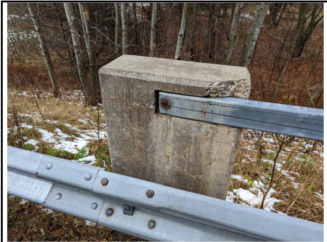
Photo 8 Spall on Northeast concrete end-post
