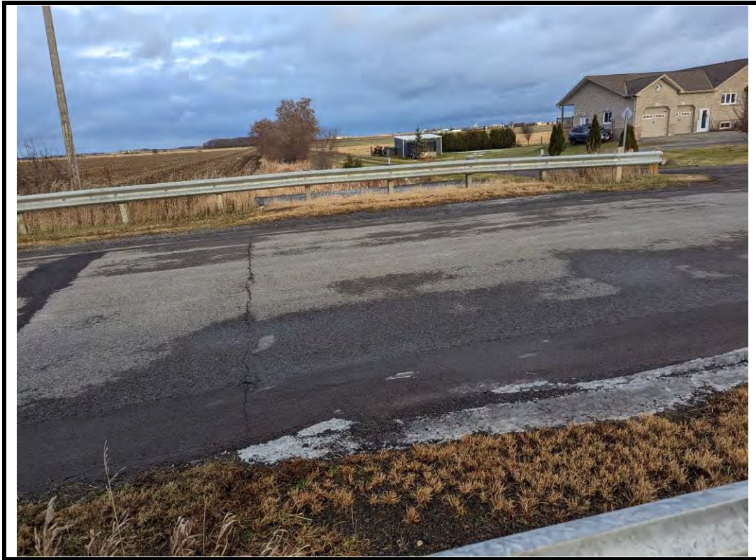
Photo 9 Wide transverse crack in wearing surface above structure with scaling and patches
