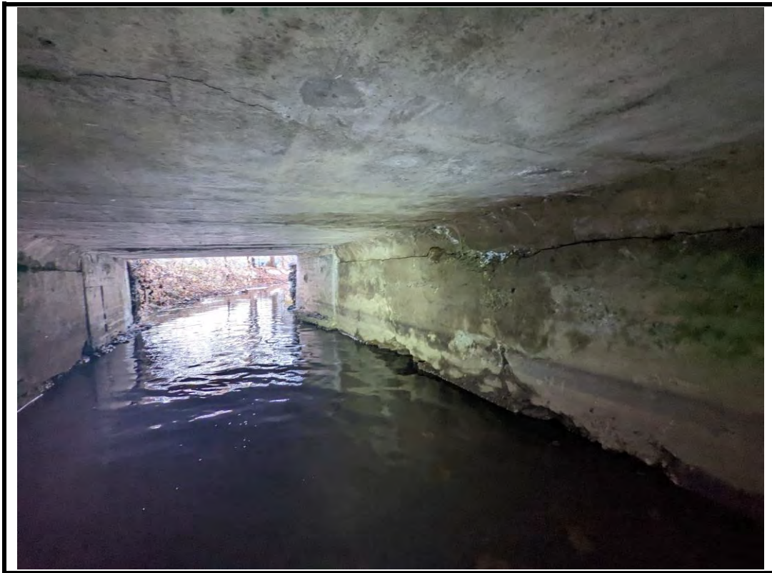
Photo 13 Cracks, scaling, spalls, staining, and scour throughout culvert (typ.)
