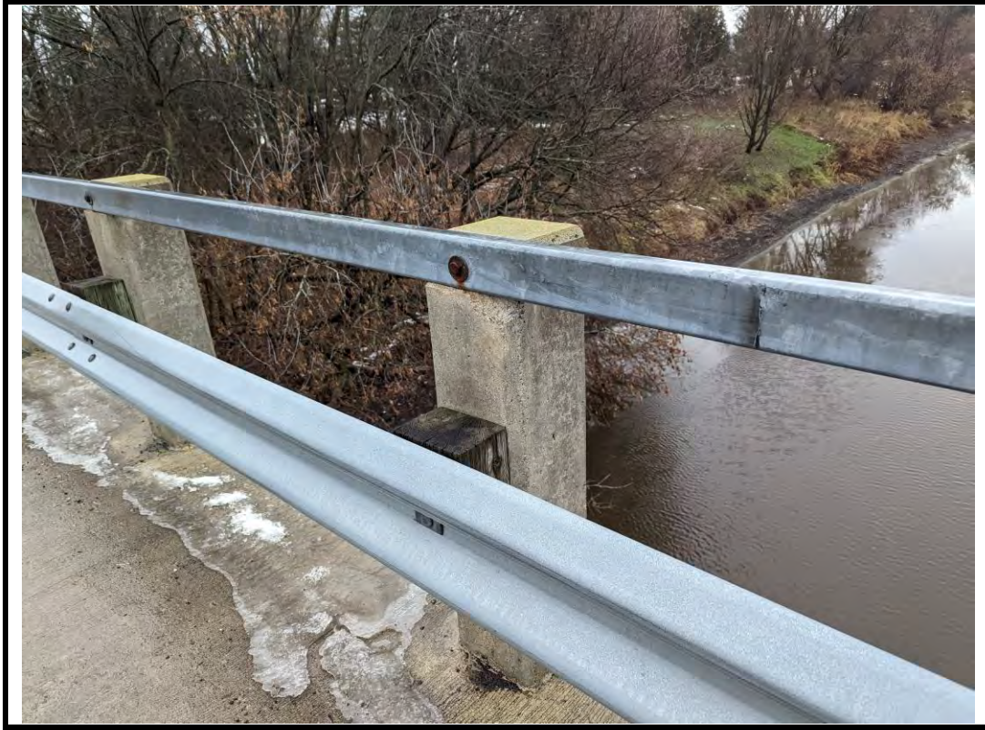
Photo 9 Spall on concrete deck post (typ.)
