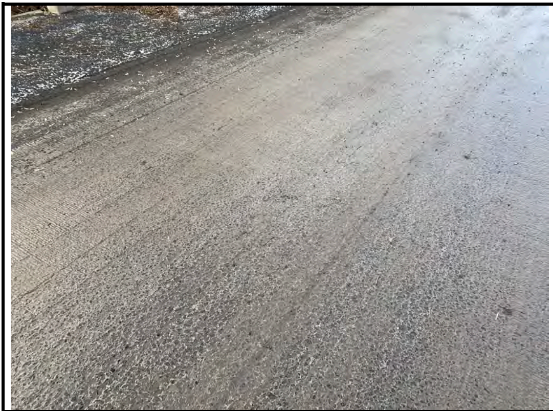
Photo 12 Wide cracks and abrasions on deck top
