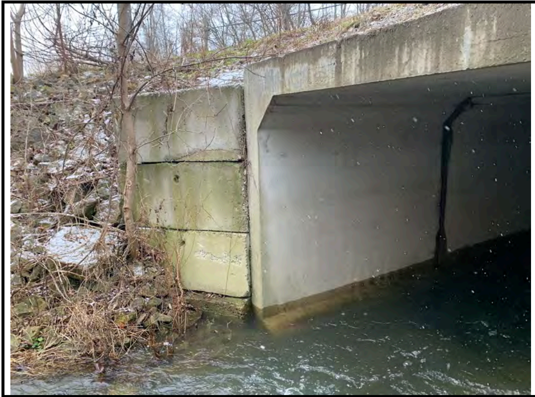
Photo 9 Honeycombing at northwest block wall
