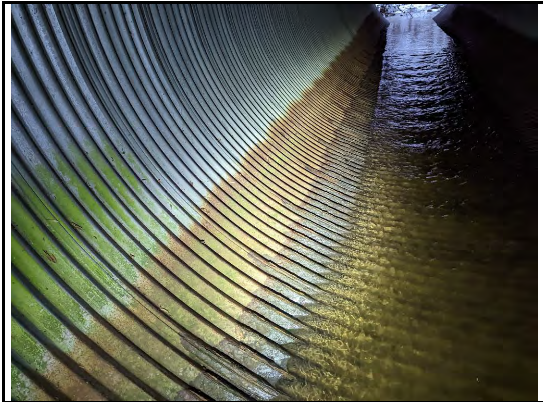
Photo 8 Corrosion along bottom of pipe
