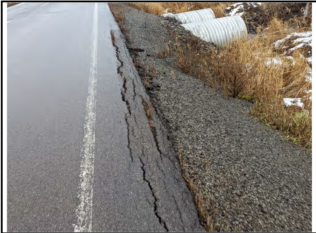
Photo 8 Longitudinal edge cracks and grade difference at shoulders
