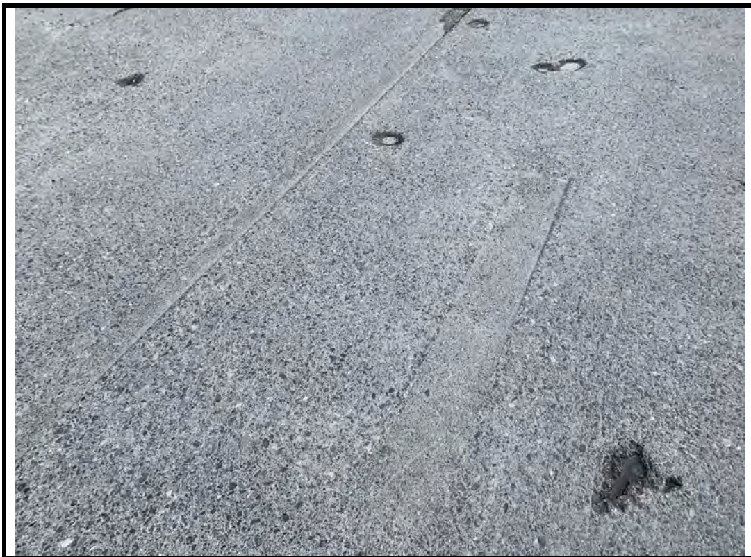
Photo 12 Abrasions and small spall on exposed deck surface
