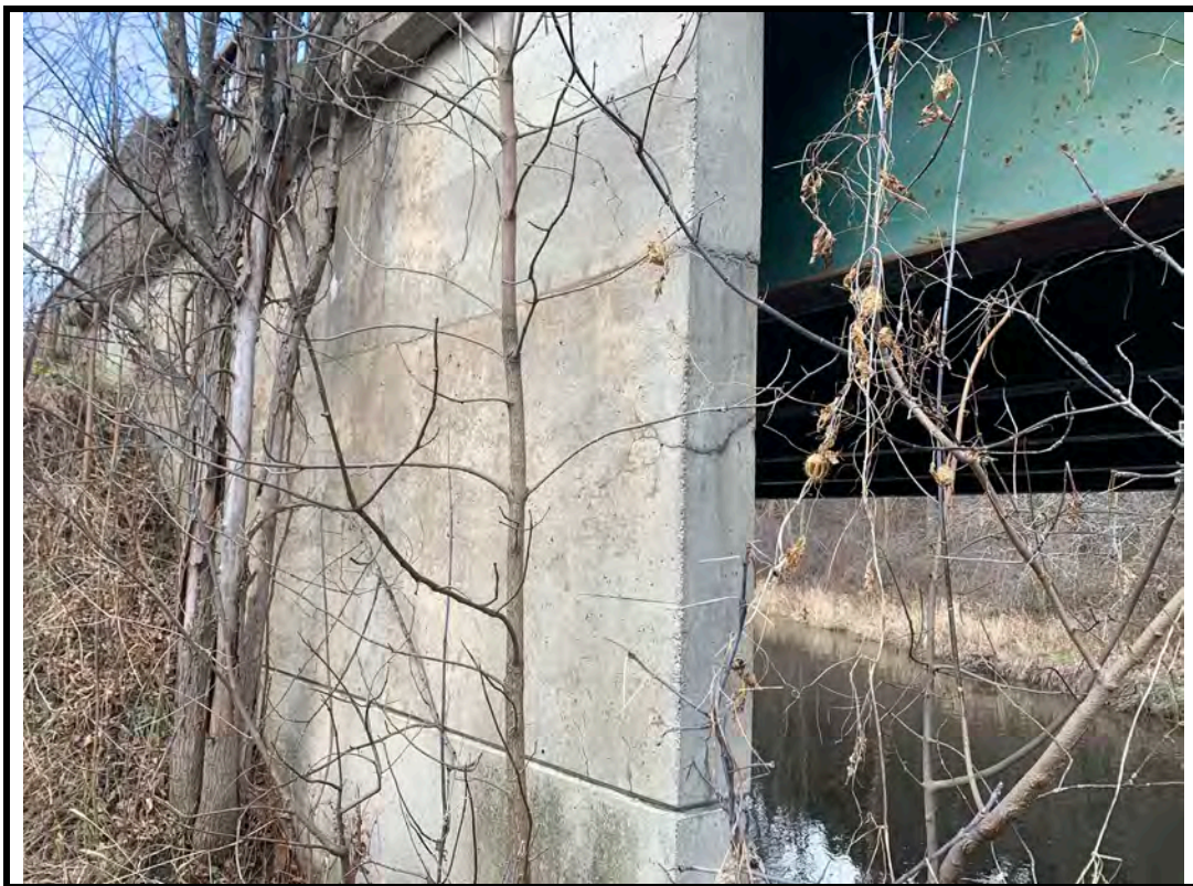
Photo 17 Crack on northwest wingwall
