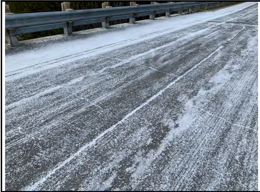
Photo 11 Wide longitudinal crack at centreline of deck wearing surface
