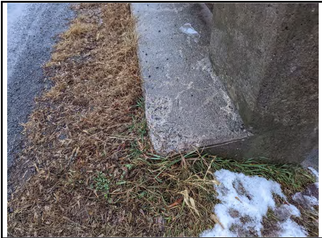
Photo 12 Spalling on east curb
