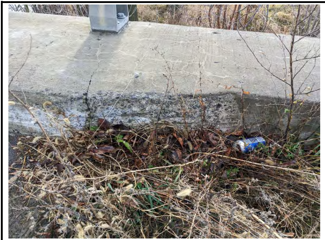
Photo 16 Scaling on deck barrier curb
