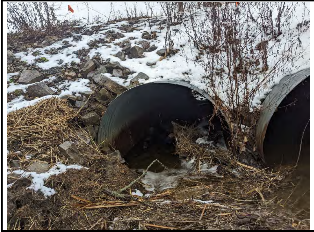
Photo 9 Debris buildup at east barrel inlet
