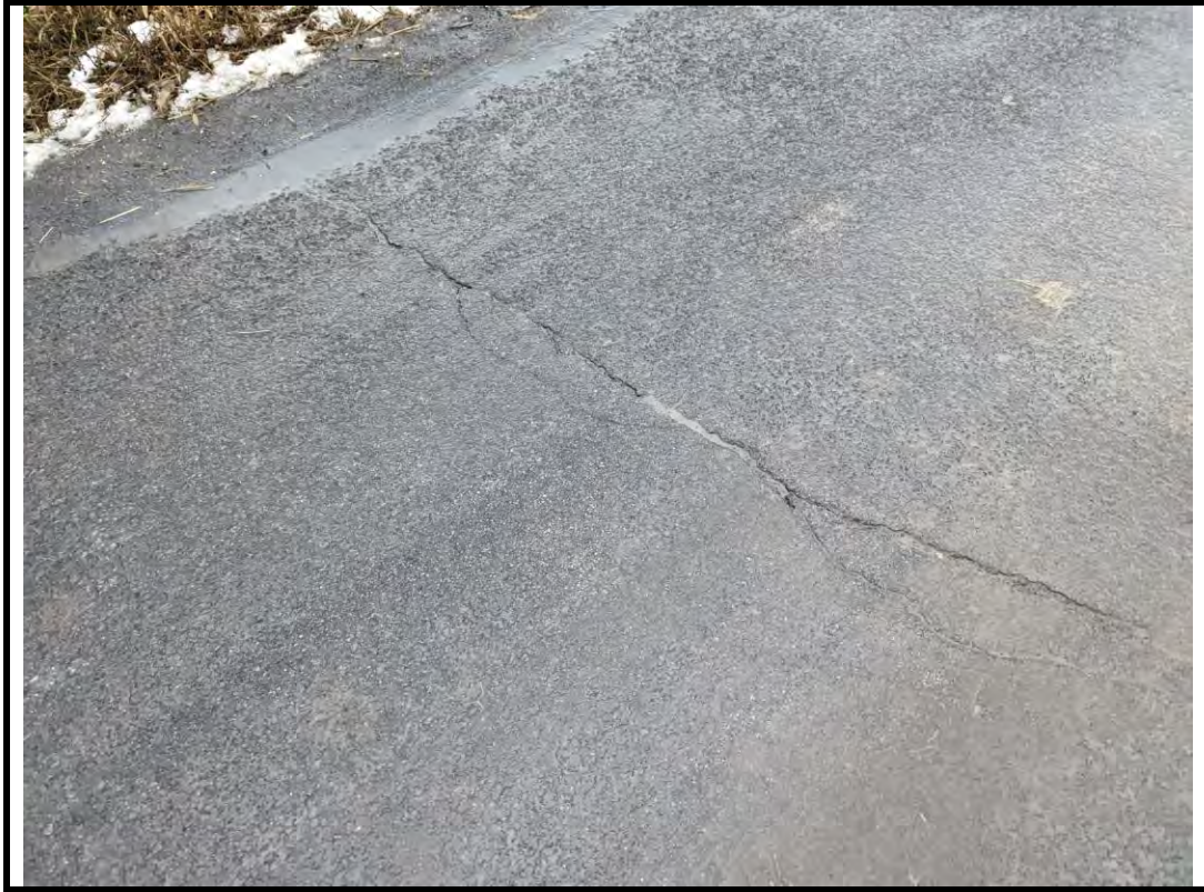
Photo 7 Transverse Crack in Approach Wearing Surface
