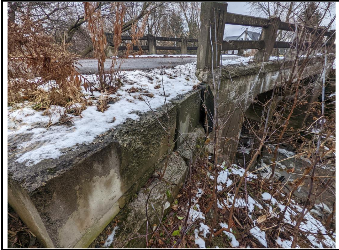
Photo9 Rotated and spalled concrete retaining walls at the northeast (typ.)
