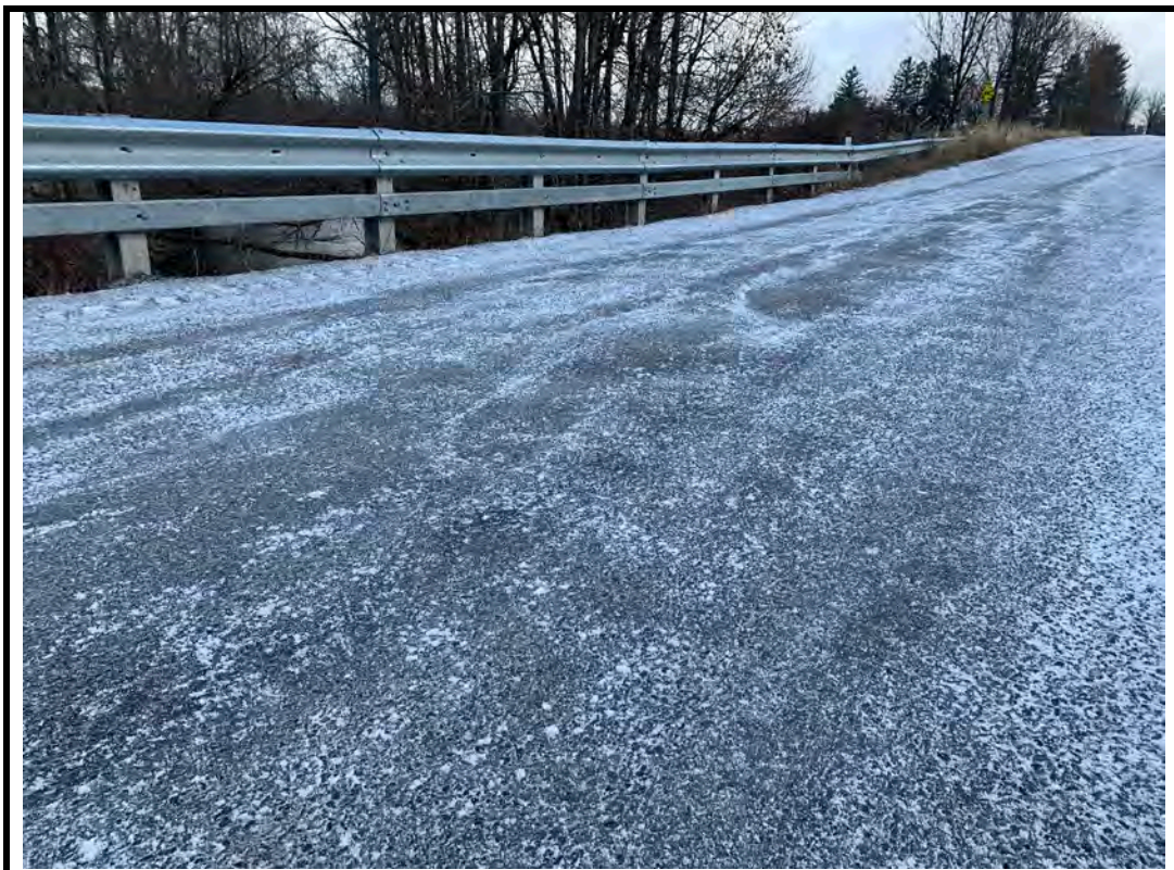
Photo 10 Moderate ravelling on deck wearing surface
