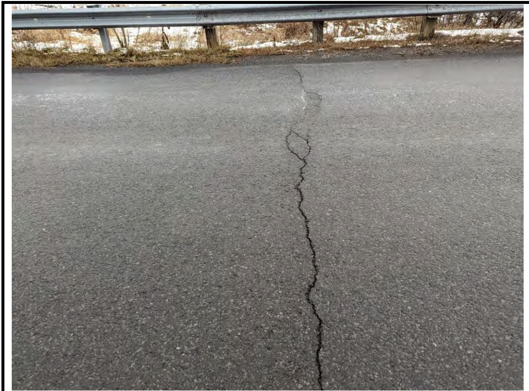
Photo 8 Wide transverse crack in asphalt wearing surface above structure
