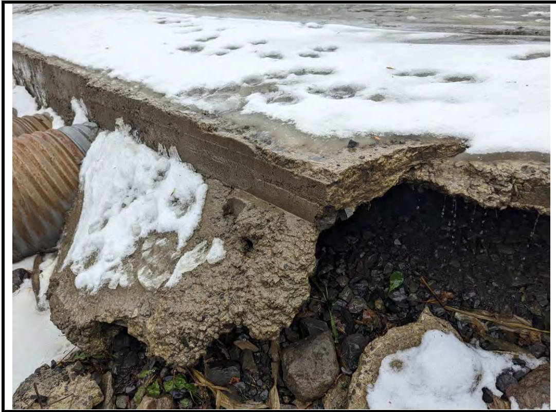
Photo 7 Severe undermining and loss of fill at North approach slab (1)
