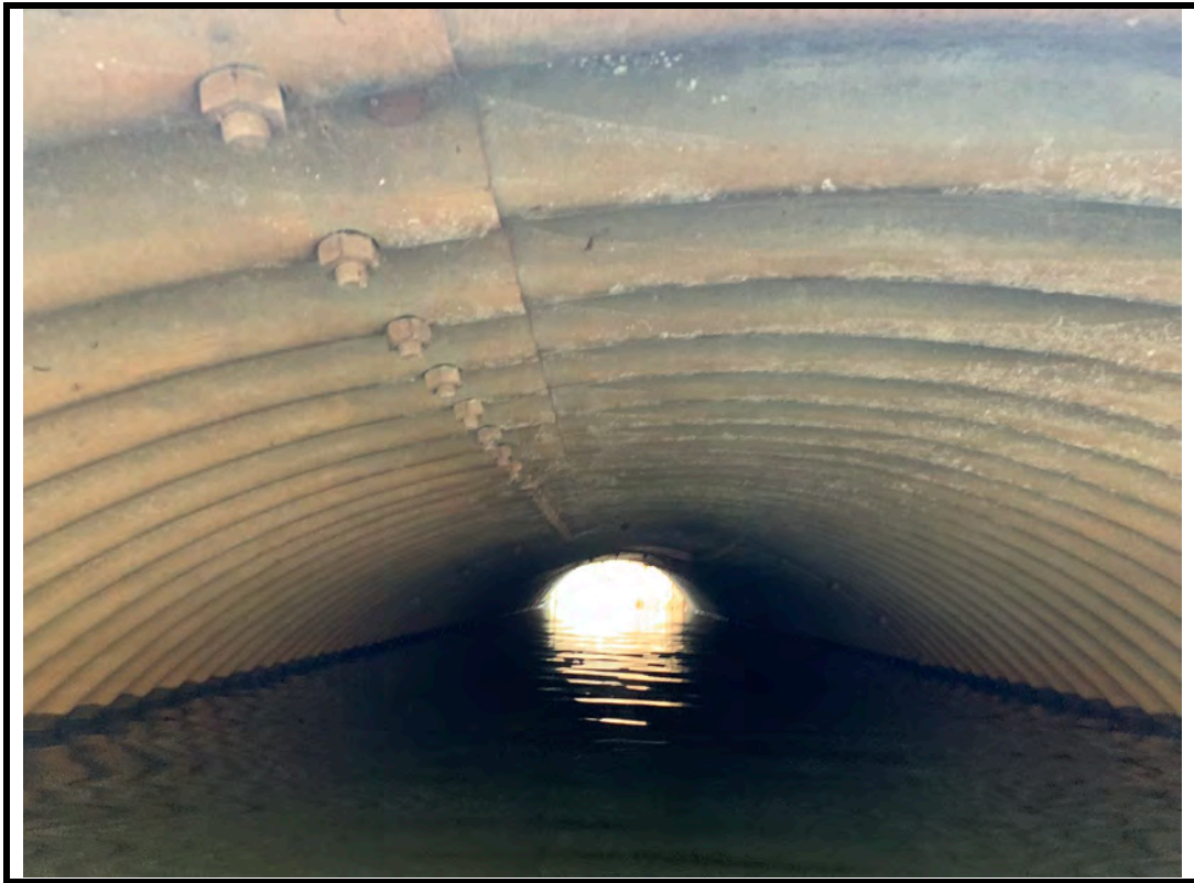
Photo 9 Slight sag in barrel under road
