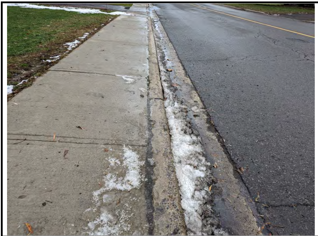
Photo 8 Scaling and cracks on southwest approach curb and gutter (typical)
