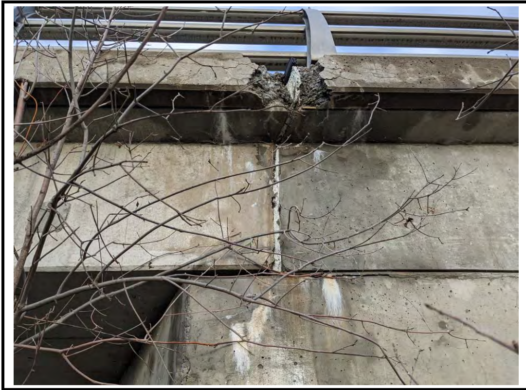
Photo 13 Spall and efflorescence at southeast joint and deck fascia
