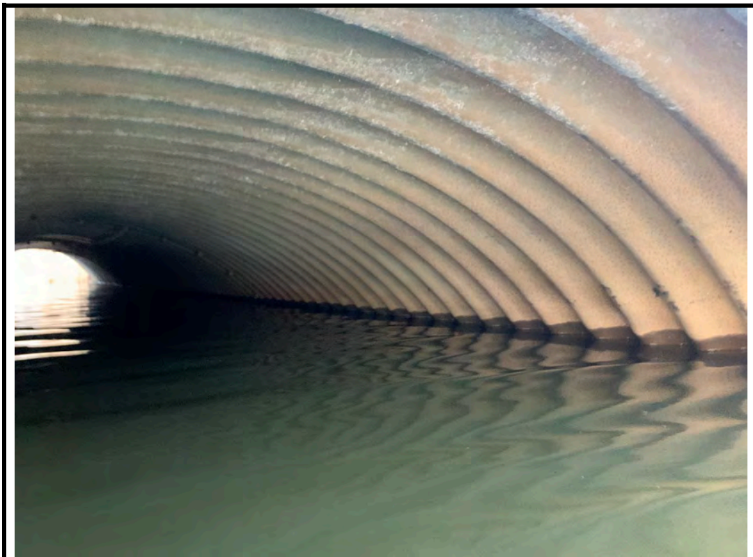
Photo 8 Light corrosion at waterline at east end of barrel
