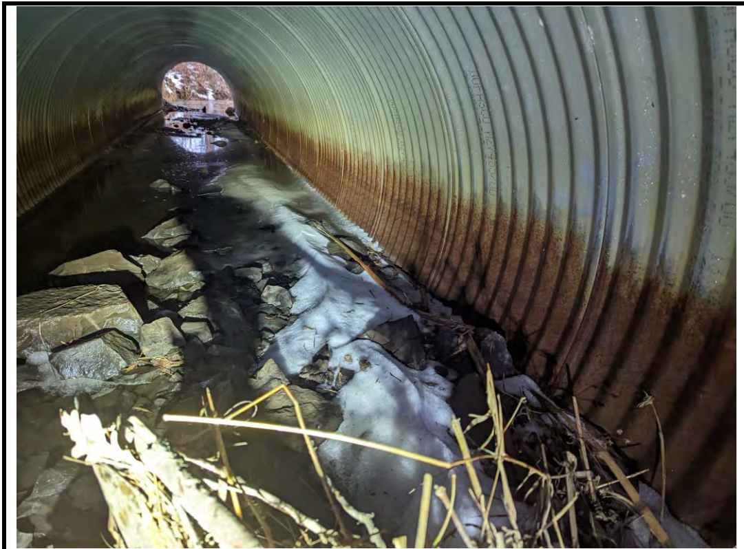
Photo 8 Corrosion and debris within east barrel
