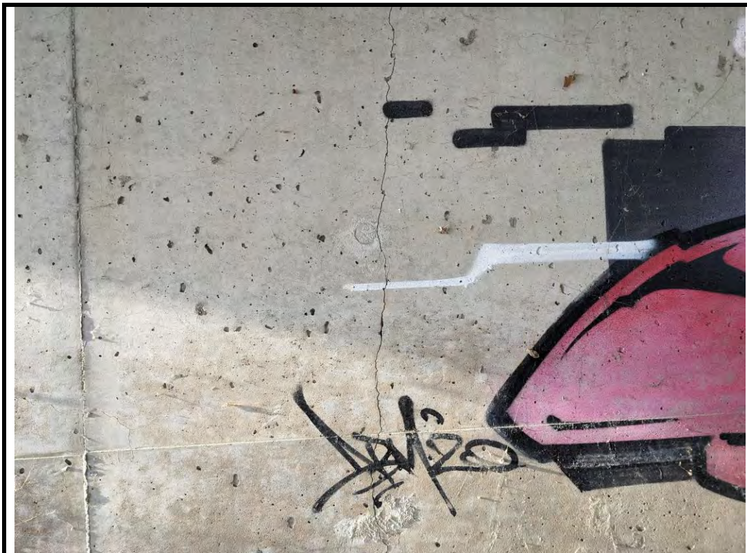
Photo 18 Crack in west abutment wall
