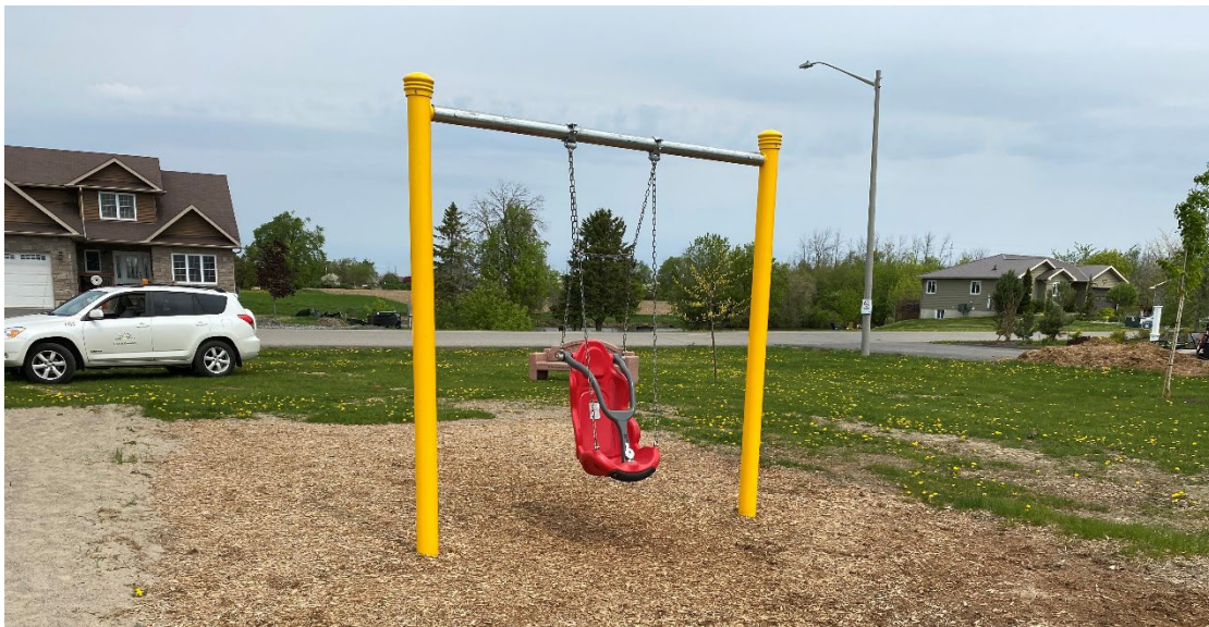
Half Bay Swing frames to accommodate one AODA Compliant swing were installed in five parks
