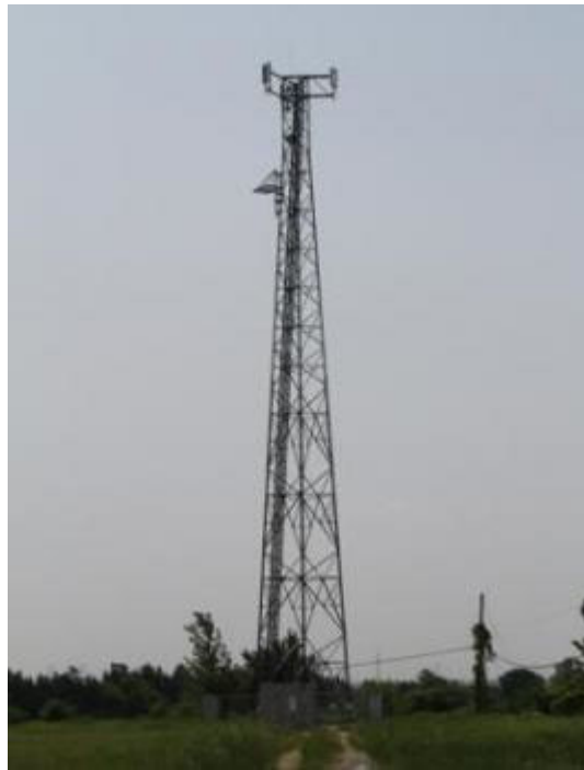
Figure 2- Example of Self Support Tower (Type S)
