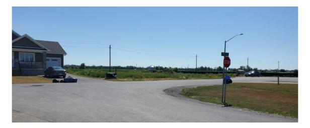
The infrastructure in this final phase of the subdivision has been constructed. Some site works are still required (parkland grading, completion of swales, lot grading, top coat of asphalt). These issues are covered under the subdivision agreement and by financial securities.
