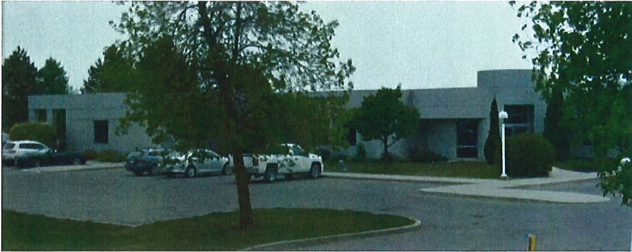
Figure 2 – 636 St. Lawrence St walkways BEFORE
